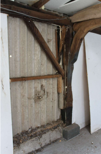
CGPF22_PhotoGraph_045Detail of a waggon shaft re-purposed as a purlin.
