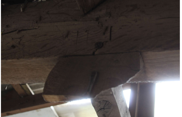
CGPF22_PhotoGraph_037Scar from concrete shoe from removed post below ti... CGPF22_PhotoGraph_038Foot of inserted post supporting tie-beam 4 resting o...
