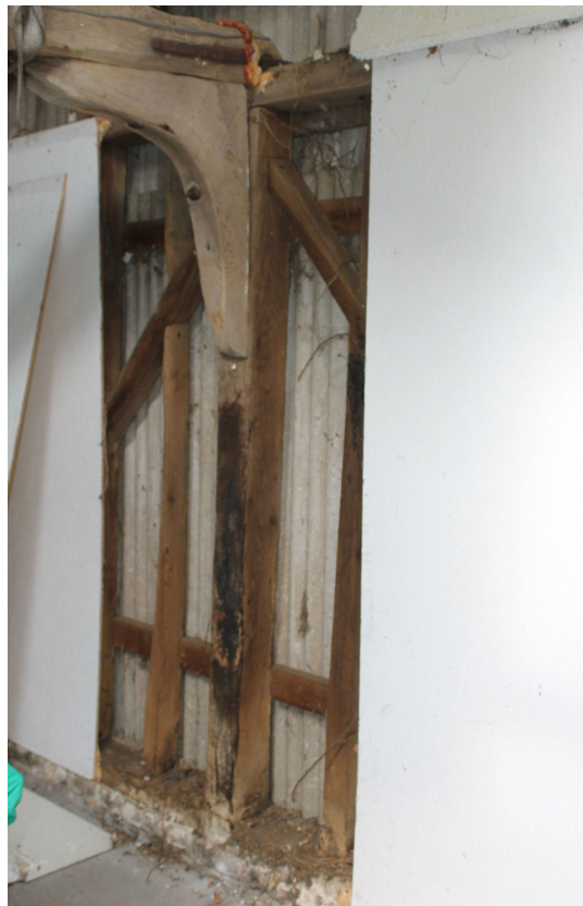
Photograph 5 Exposed timber-frame of the north wall.
