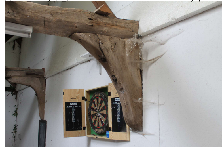
CGPF22_Photograph_019Southern knee-brace of tie-beam 2. Photograph take... CGPF22_Photograph_020Southern knee-brace of tie-beam 2. Photograph take...
