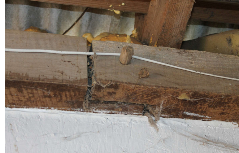
CGPF22_PhotoGraph_039Wall plate face-halved and timber-pegged scarf joint. CGPF22_PhotoGraph_040Timber-frame of northern wall. Photograph taken faci...
