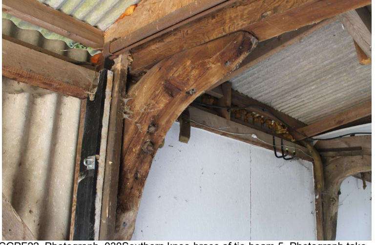
CGPF22_Photograph_030Southern knee-brace of tie-beam 5. Photograph take...
