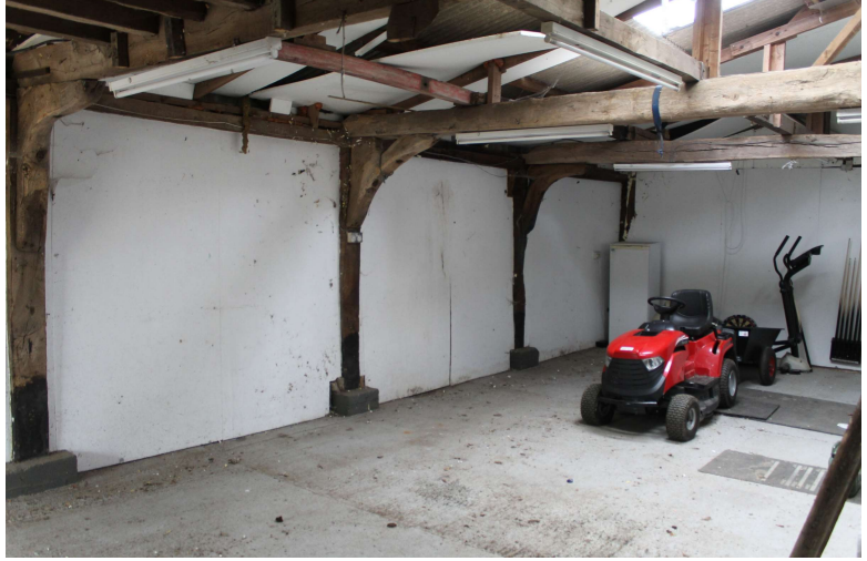
CGPF22_Photograph_012Northern knee-brace of tie-beam 1. Photograph take...
