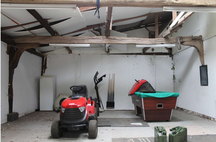
CGPF22_Photograph_013Northern knee-brace of tie-beam 1. Photograph take...
