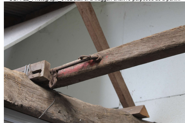
CGPF22_PhotoGraph_045Detail of a waggon shaft re-purposed as a purlin.
