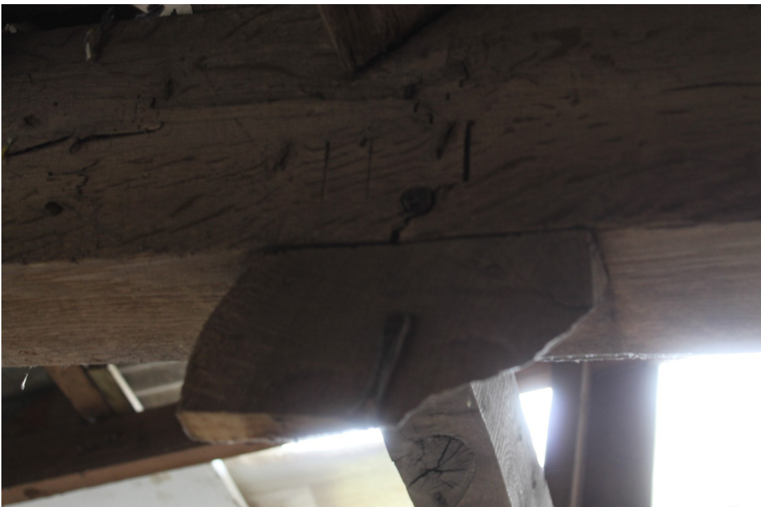
Photograph 12 Carpenter's mark on tie-beam T3 above the remains of an inserted post to support the loft.
