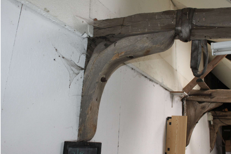
CGPF22_Photograph_015Southern knee-brace of tie-beam 1. Photograph take...
