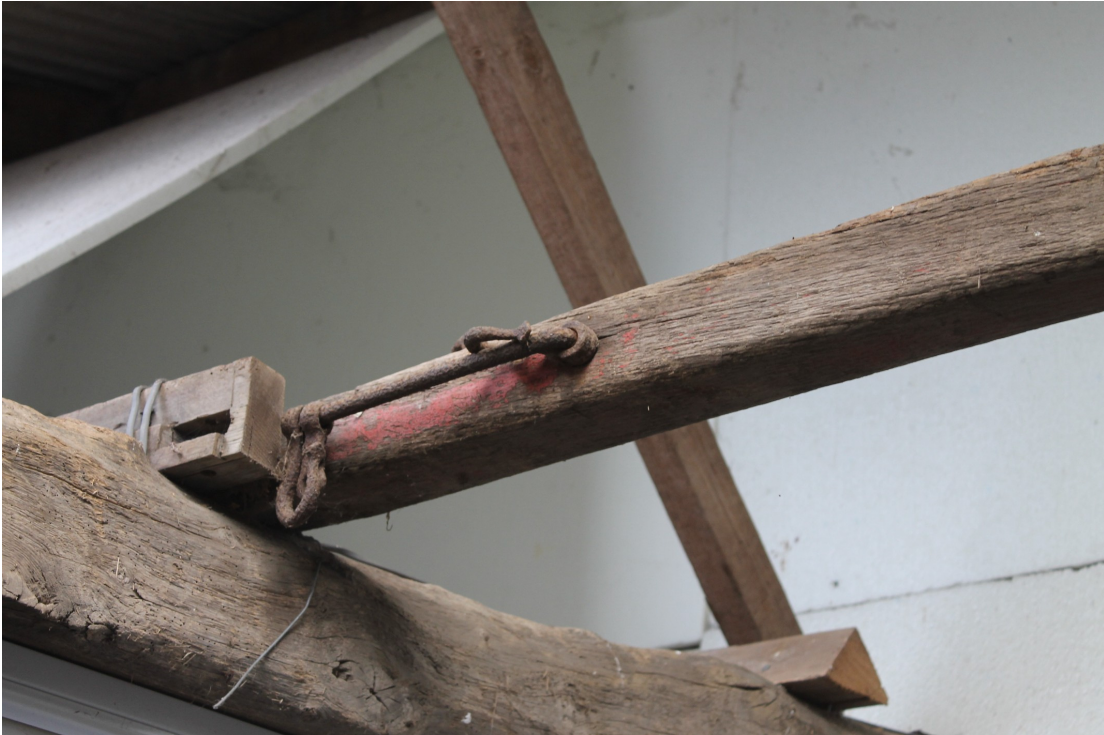
Photograph 16 Waggon shaft (complete with harness attachment) fixed to a section of door post to form a crude longitudinal purlin supporting the struts of the modern roof.
