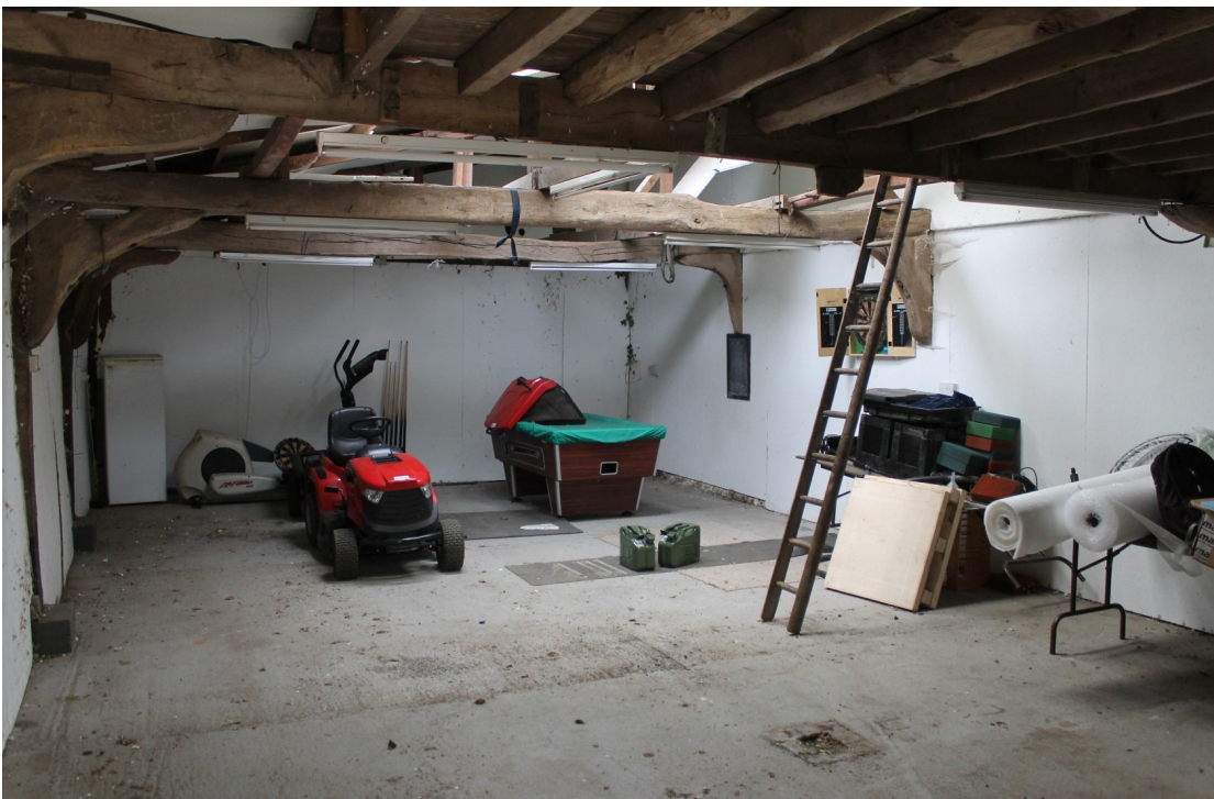
Photograph 3 Interior of the cart lodge with the north wall to the right – view north-west.
