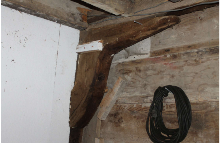
CGPF22_Photograph_028Southern knee-brace of tie-beam 4. Photograph take...
