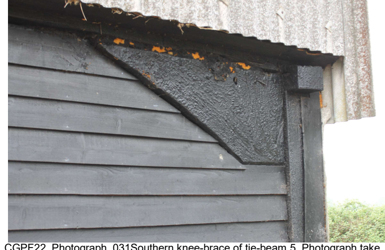
CGPF22_Photograph_031Southern knee-brace of tie-beam 5. Photograph take...
