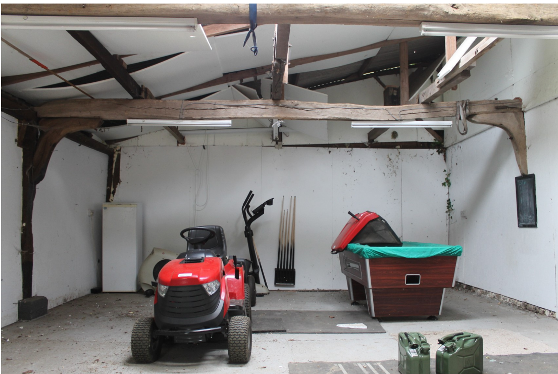
Photograph 10 Tie-beam T1 with knee braces – view west.
