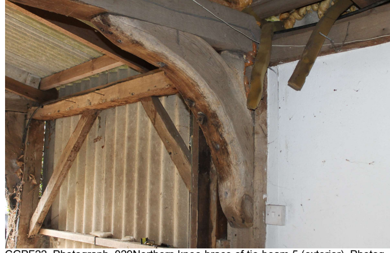
CGPF22_Photograph_029Northern knee-brace of tie-beam 5 (exterior). Photog...
