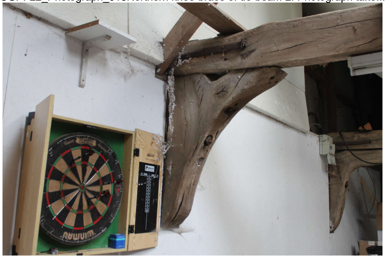
CGPF22_Photograph_019Southern knee-brace of tie-beam 2. Photograph take... CGPF22_Photograph_020Southern knee-brace of tie-beam 2. Photograph take...
