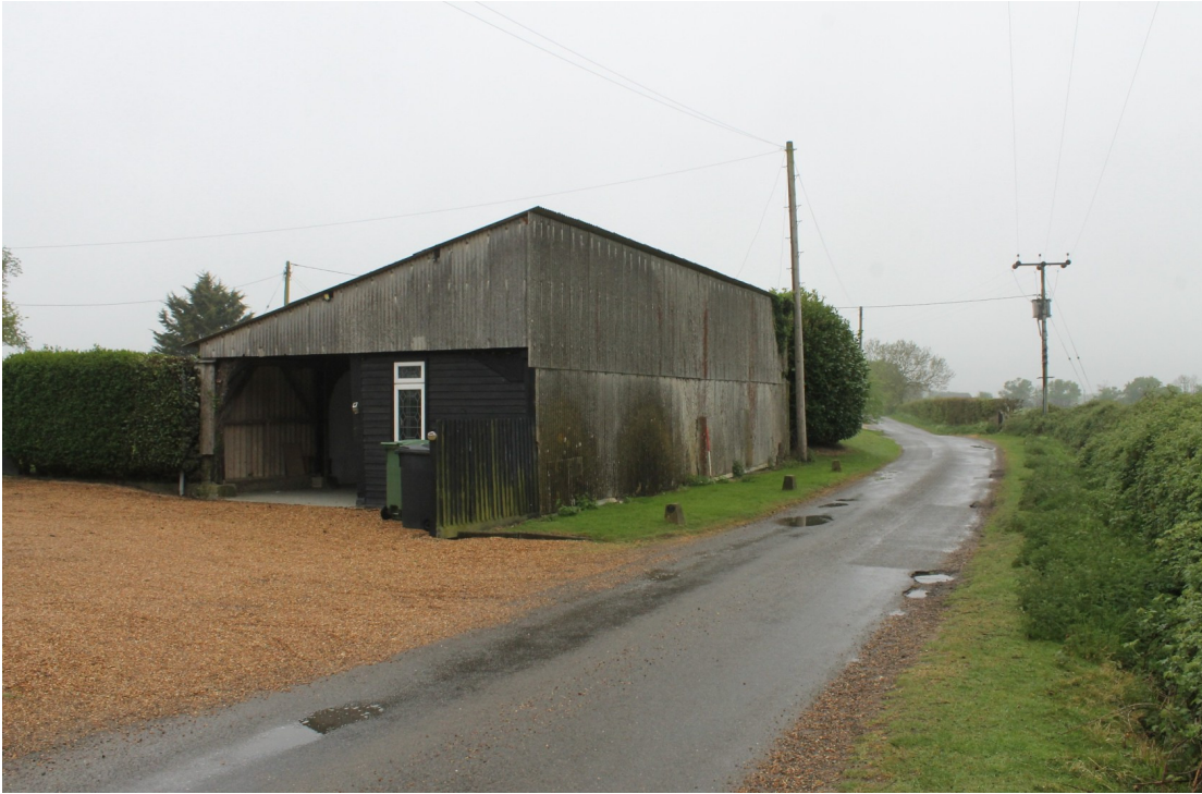
Photograph 1 North and east elevations – view south-west.
