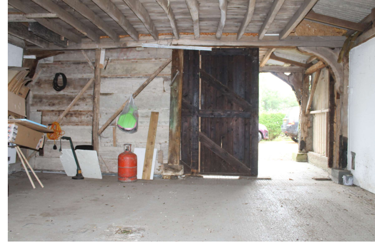
CGPF22_Photograph_027Southern knee-brace of tie-beam 4. Photograph take...
