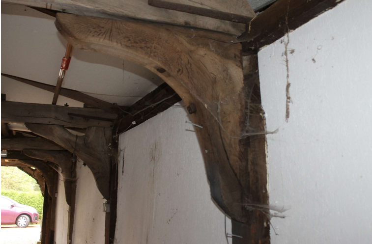
CGPF22_Photograph_015Southern knee-brace of tie-beam 1. Photograph take...
