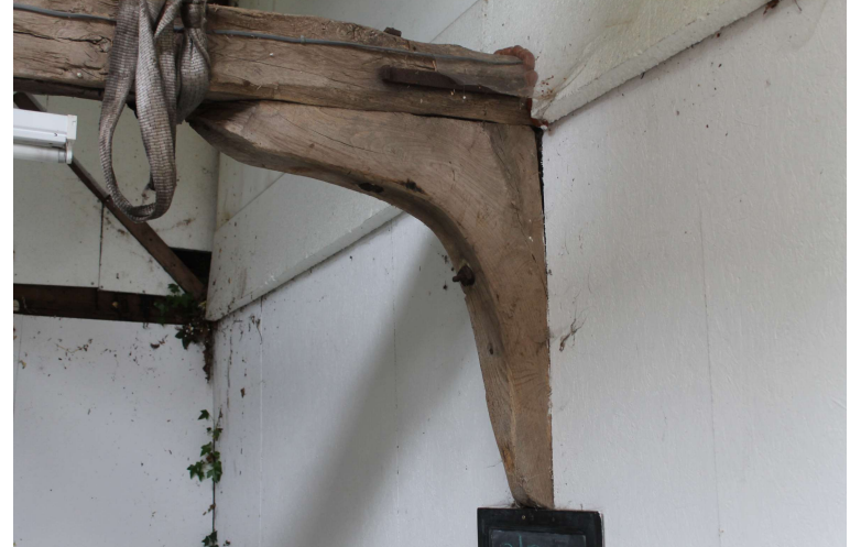
CGPF22_Photograph_014Southern knee-brace of tie-beam 1. Photograph take...
