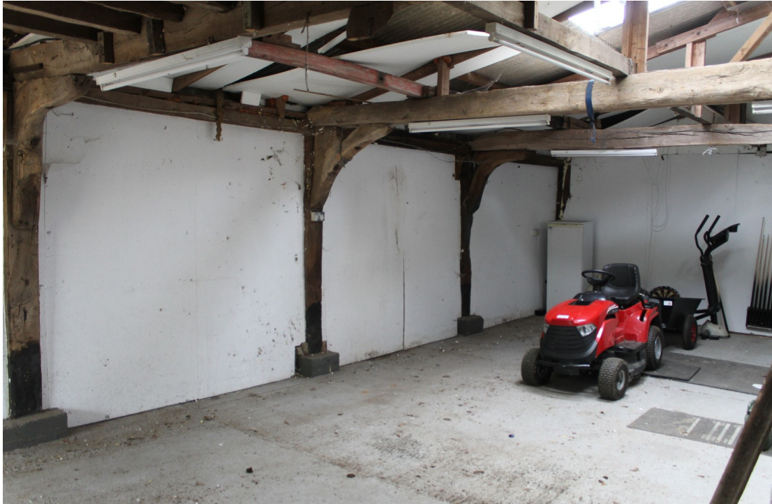
Photograph 4 Interior of the cart lodge showing the south wall with its exposed posts and protective concrete shoes – view south-west.
