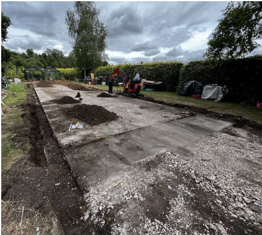
Photograph 1 View of south end of footings, looking north-east.
