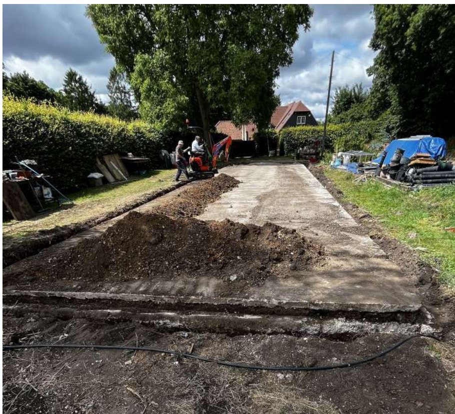
Photograph 2 View of north end of footings, looking south-west.
