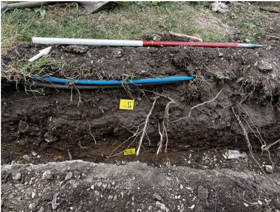
Photograph 4 Section of footings showing modern pipes and significant rooting. Looking roughly north-west.
