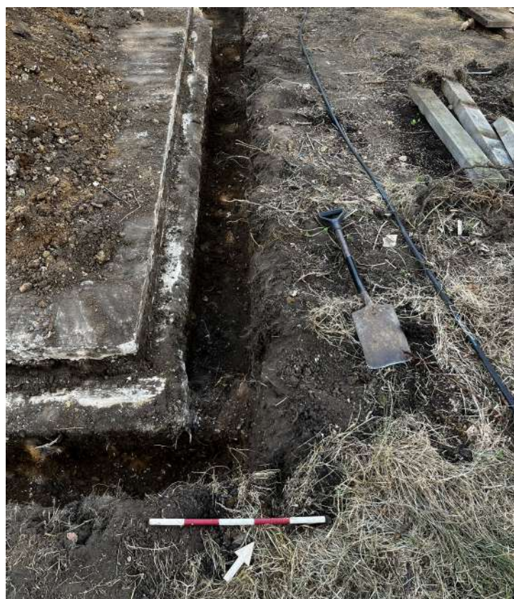
Photograph 3 North end of footings, showing concrete from former outbuilding, looking north-east.
