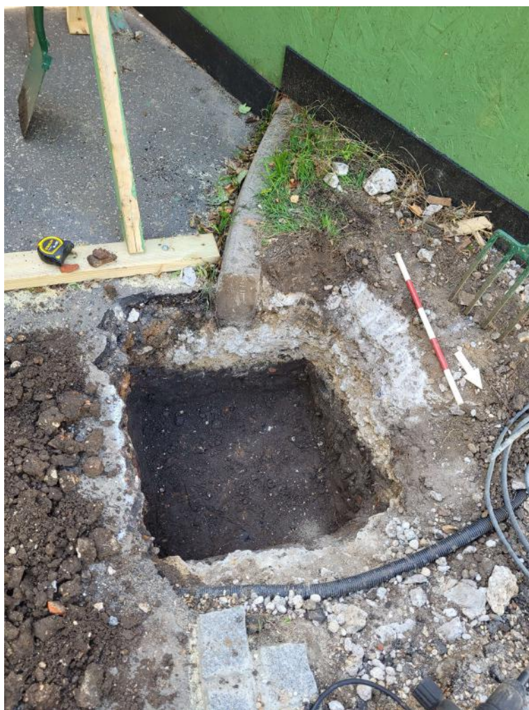
Photograph 2 Post-excitation shot of foundation pad 1, looking south-south-west
