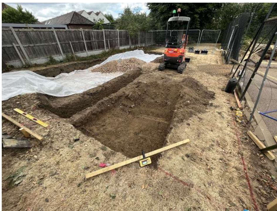
Photograph 2 Excavation of Pad 2, looking north-west
