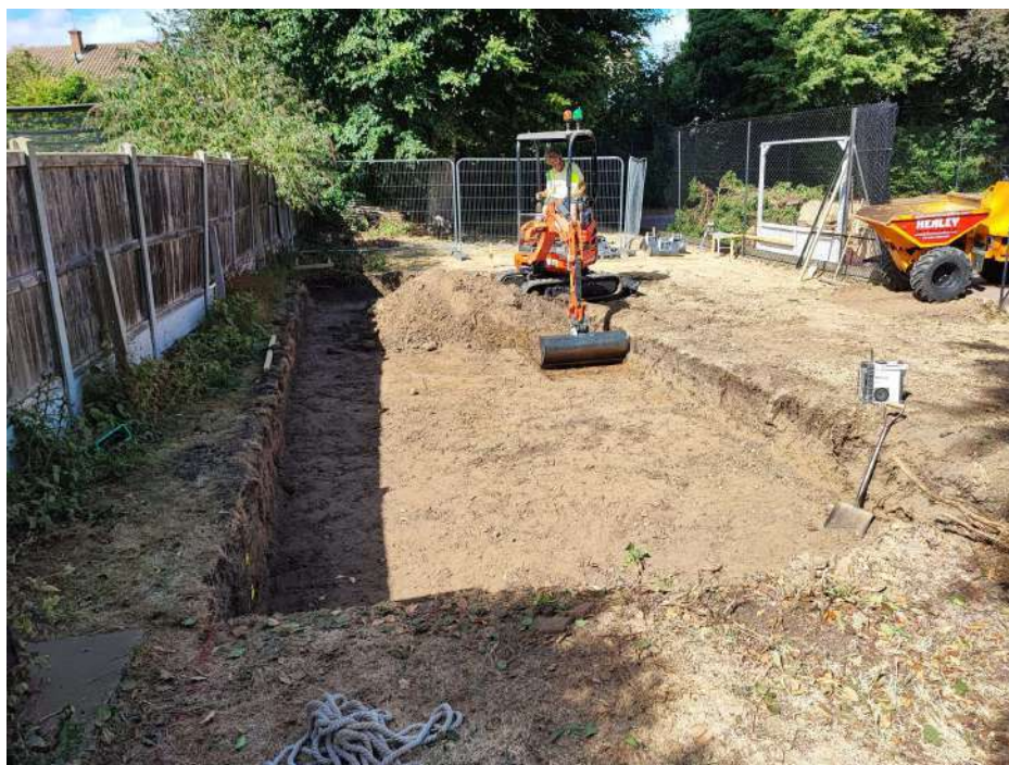
Photograph 1 Pad 1, looking north-east
