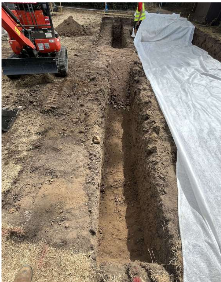
Photograph 3 Excavation of drainage trench, looking north
