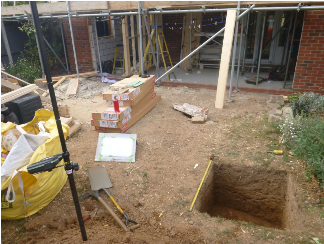
Photograph 1 Test-pit looking north-west towards the new extension.
