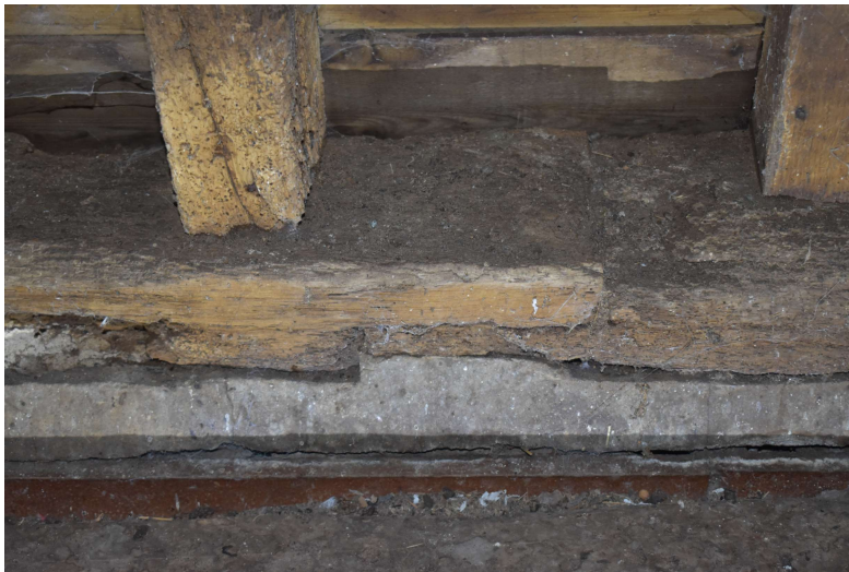
SOWBF22_PhotoGraph_063Detail of cement-filled mortices on sill-bea... SOWBF22_PhotoGraph_064Detail of timber frame in store 4. Photogra...
