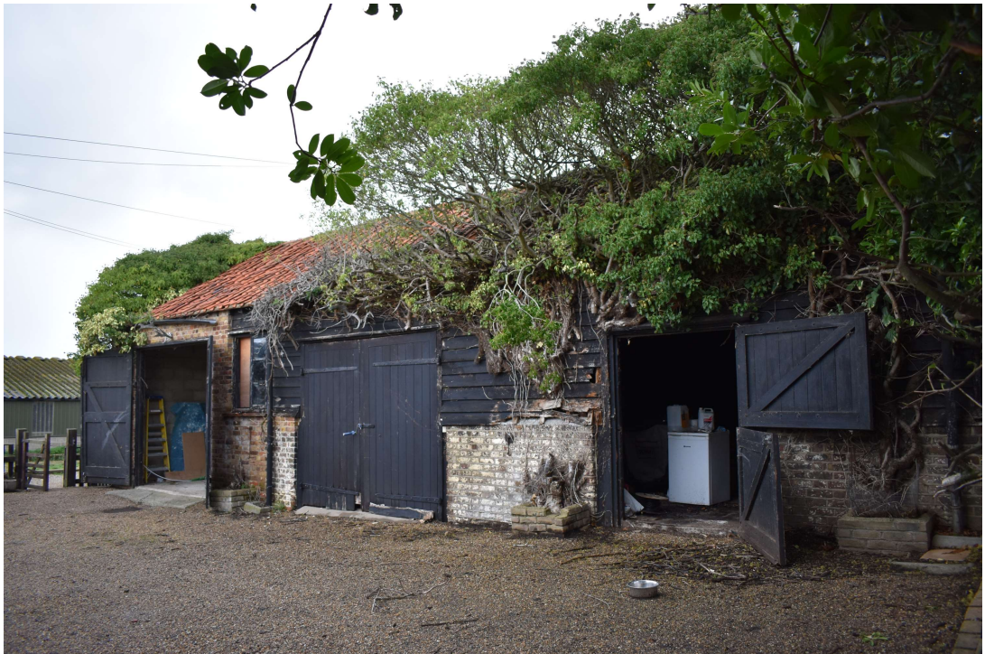
Photograph 1 South-east elevation. Photograph taken facing north north-west.
