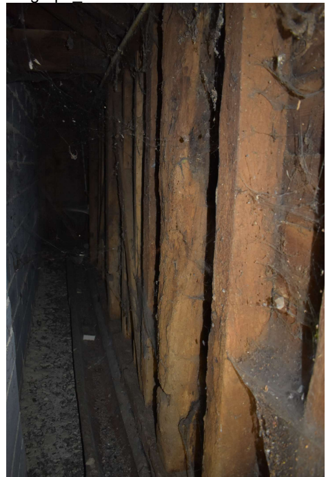
SOWBF22_PhotoGraph_065Detail of scarf joint in sill-beam in store 3. ... SOWBF22_PhotoGraph_066Detail of metal strap in tie-beam between ...
