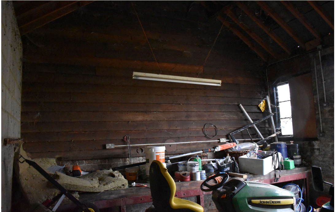
Photograph 9 Interior of Store 1. Photograph taken facing south-east.
