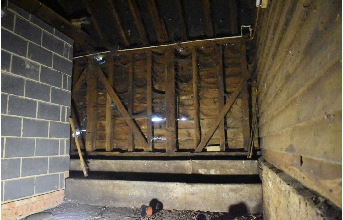
Photograph 13 Interior of Store 4. Photograph taken facing north-east.
