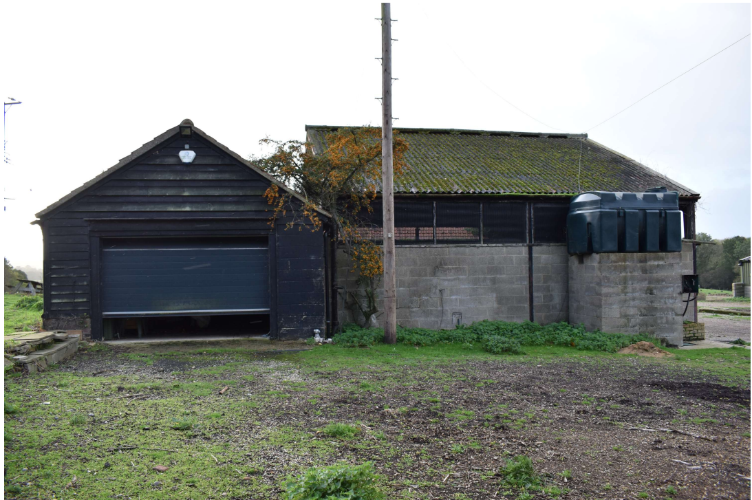
Photograph 4 North-west elevation. Photograph taken facing south-east.
