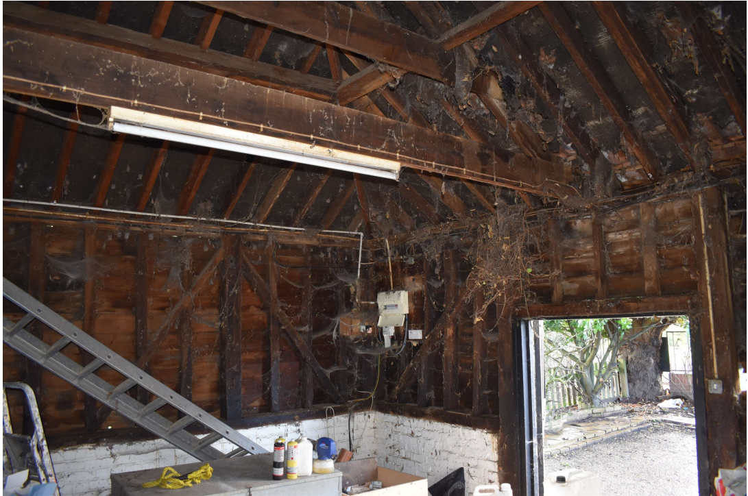
Photograph 11 Interior of Store 3. Photograph taken facing south-east.
