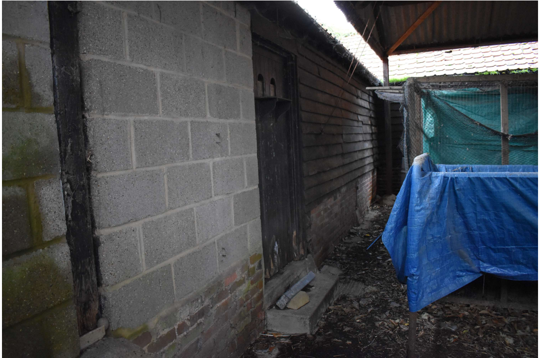
Photograph 6 Internal elevation in Store 5. Photograph taken facing south-east.
