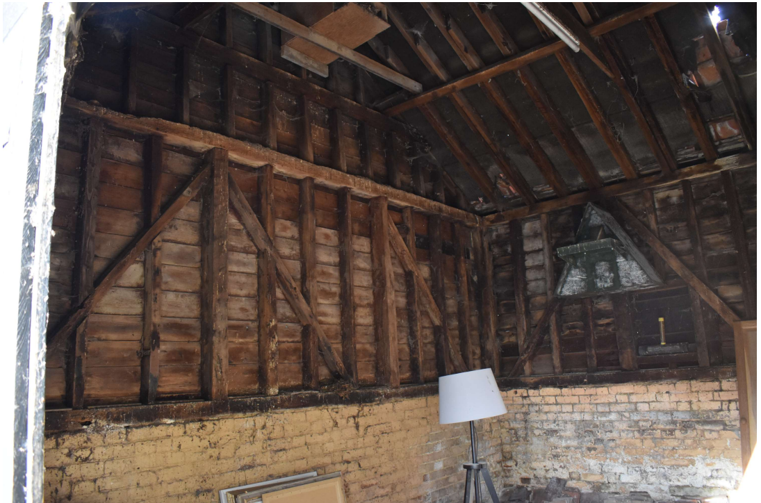
Photograph 10 Interior of Store 2. Photograph taken facing north-west.
