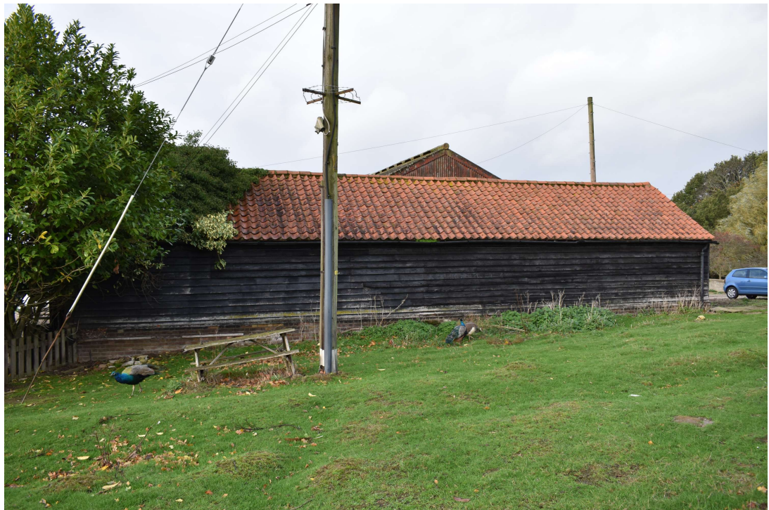
Photograph 5 North-east elevation. Photograph taken facing west.
