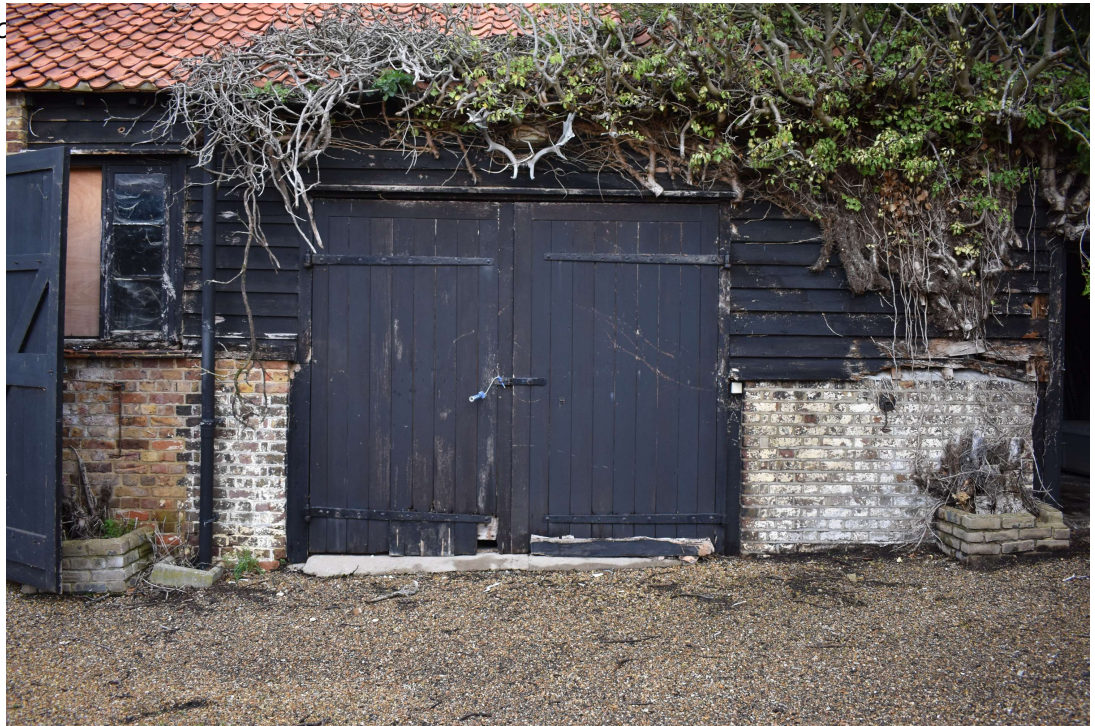
Photograph 2 Detail of double-doors on south-east elevation. Photograph taken facing north-west.
