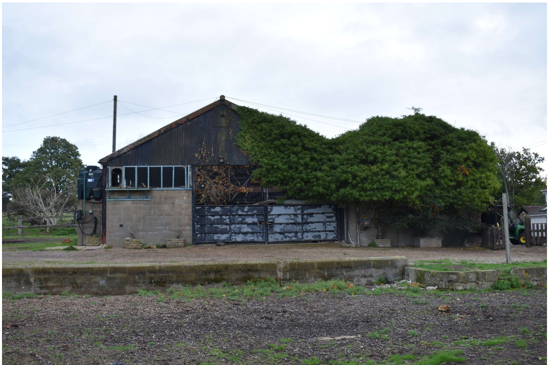
Photograph 3 South-west elevation. Photograph taken facing north-east.
