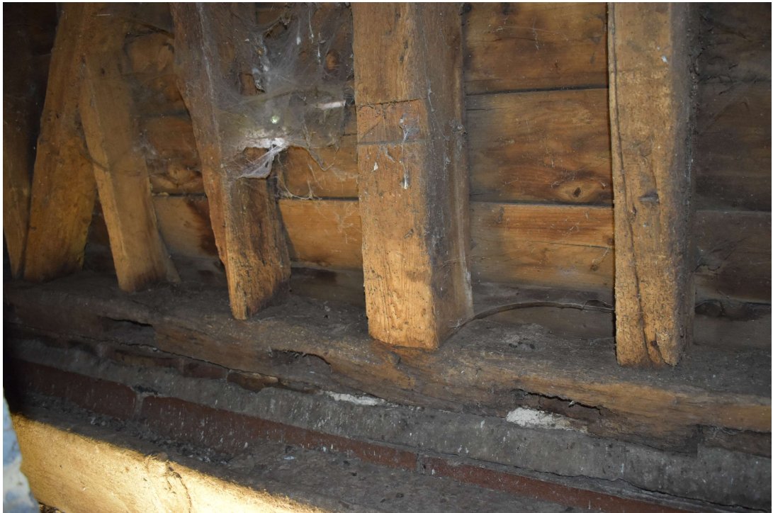
Photograph 14 Detail of reused timber for sill-beam in Store 4. Photograph taken facing north-east.
