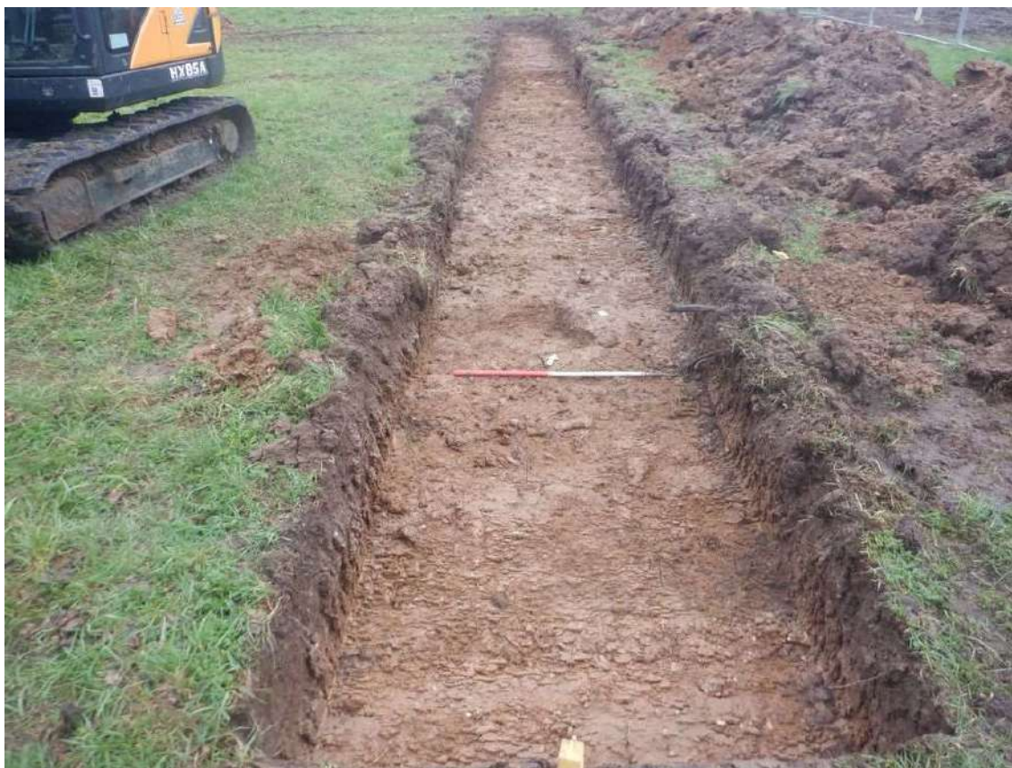
Photograph 4 Trench 5, looking north-west.
