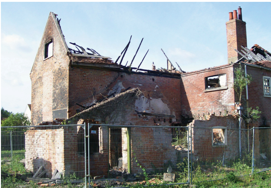
Plate 6: the east elevation (oblique angle).
