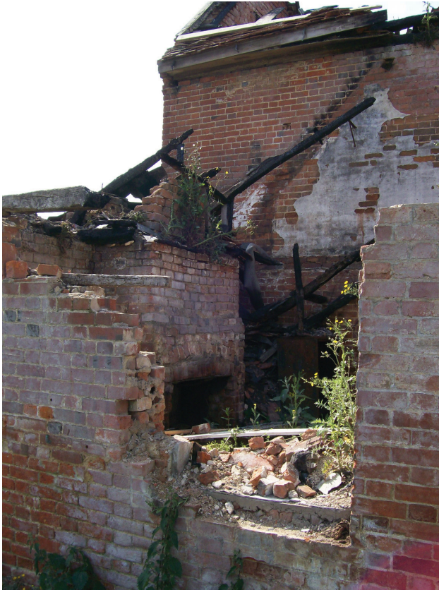
Plate 11: north elevation, showing pantry fireplace.
