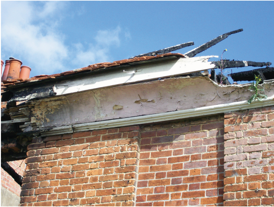
Plate 7: detail of the plaster cornice and eaves.
