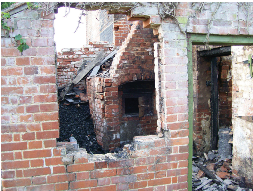
Plate 12: north elevation - boiler room, showing furnace.
