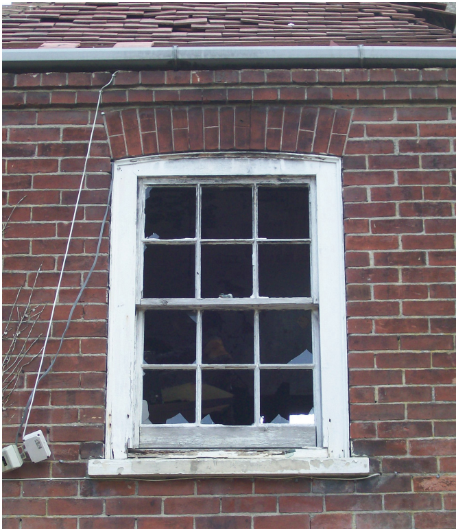
Plate 8: west elevation upper-storey sash window.
