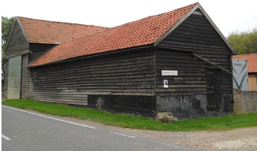
Plate 17 Building attached to large barn (D), viewed from south-east.
