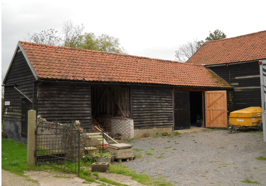
Plate 14 Building attached to large barn (D), viewed from south-east.
