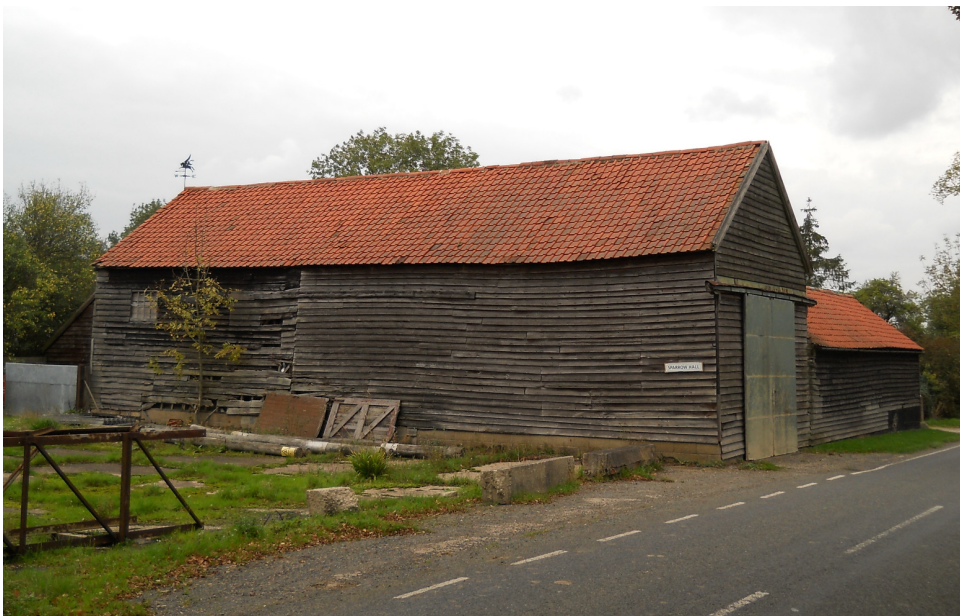
Plate 7 Large barn (E), south-west wall and south-east wall, viewed from south.
