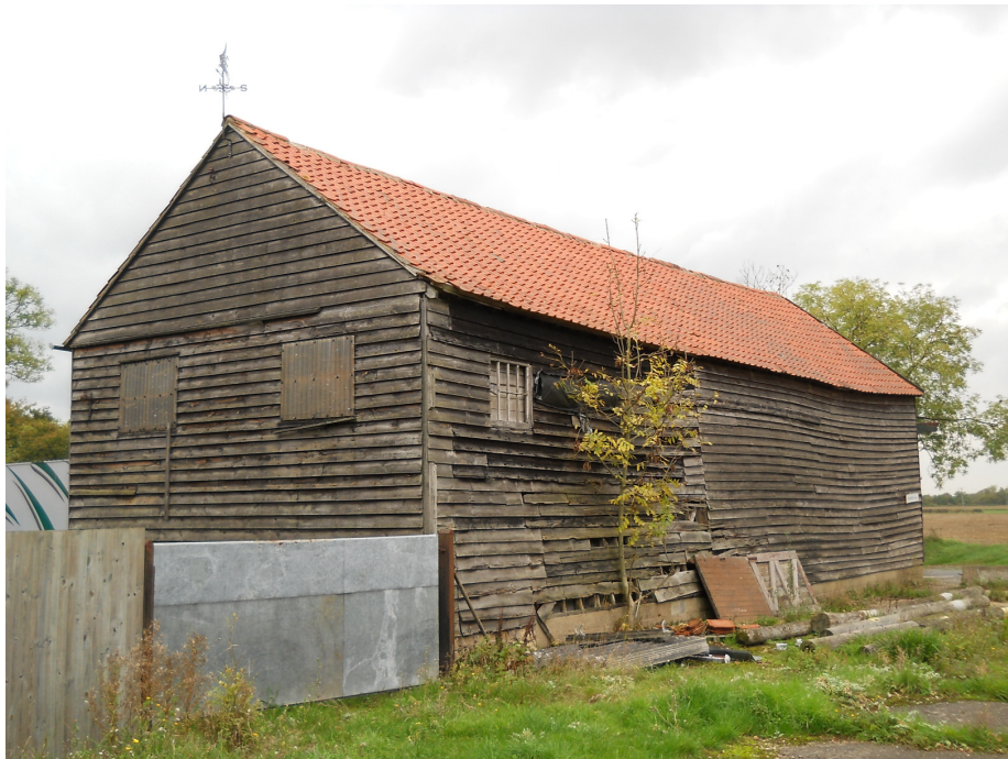
Plate 3 Large barn (E), south-west wall, exterior, viewed from west.
