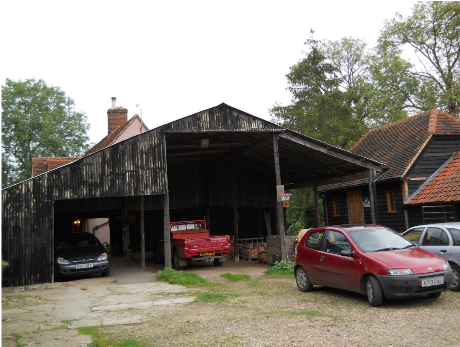
Plate 50 Pole barn (H), viewed from south-west.
