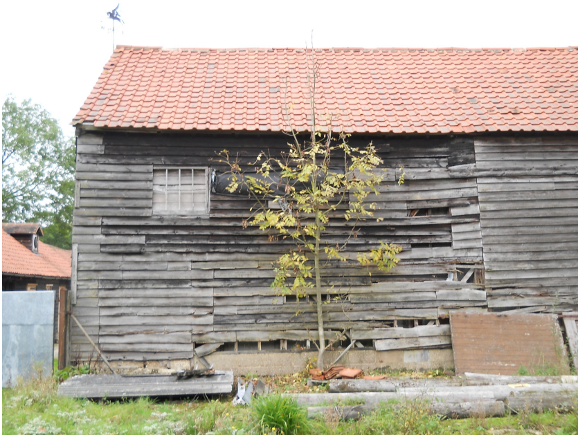
Plate 5 Large barn (E), south-west wall, exterior, showing position of former lean-to.
