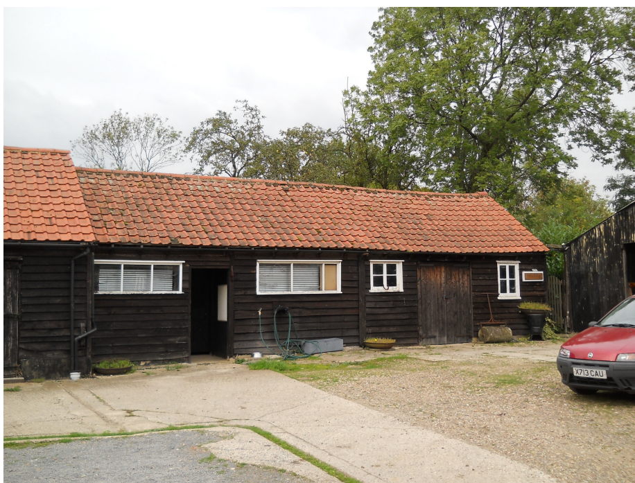
Plate 31 Cart lodge attached to stables (G), viewed from south-east.
