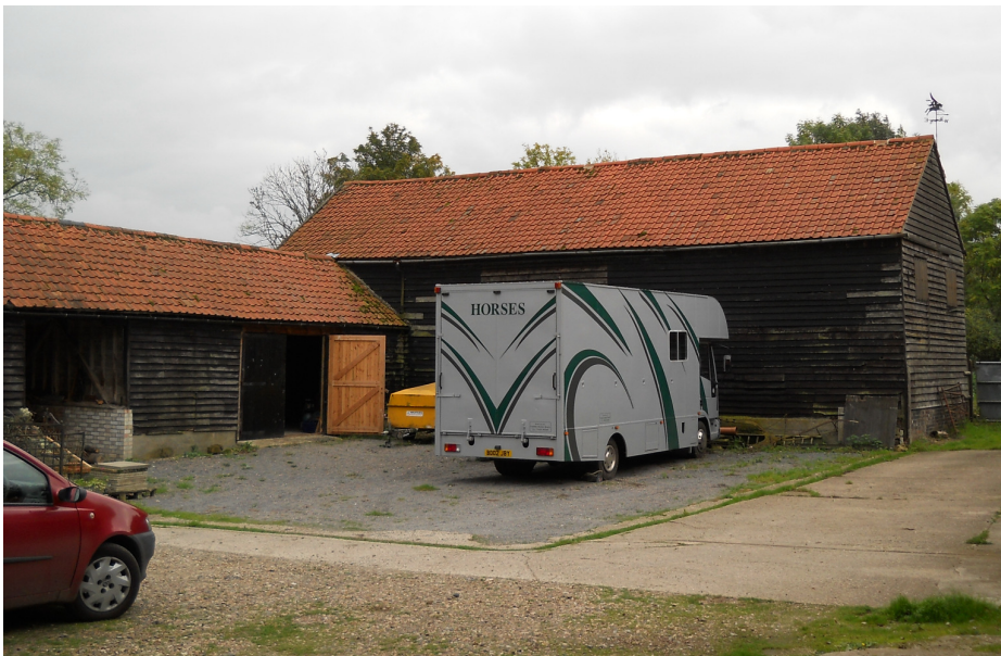
Plate 1 Large barn (E) with attached building (D), viewed from north-east.
