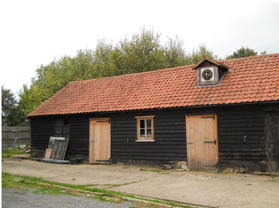
Plate 29 Loose box/stables (F), viewed from south-east.
