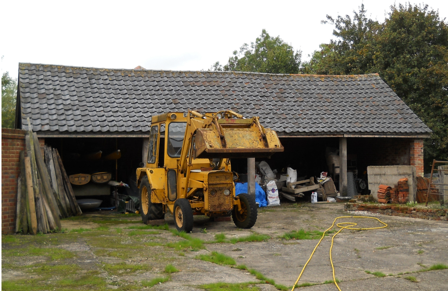
Plate 9 19th-century cart lodge (Q) between ruined barn (S) and house converted from barn (O) to south, viewed from the east.
