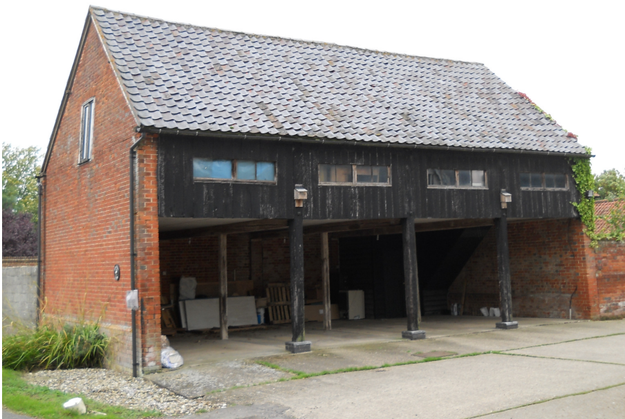
Plate 2 19th-century cart lodge/granary (M), viewed from the south-east.
