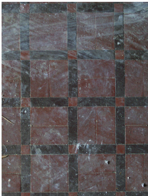
Appendix Plate 9 Detail of original lounge floor tiles.
