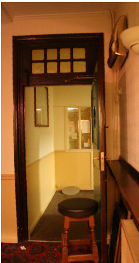
Appendix Plate 12 Original external doorway in west wall.
