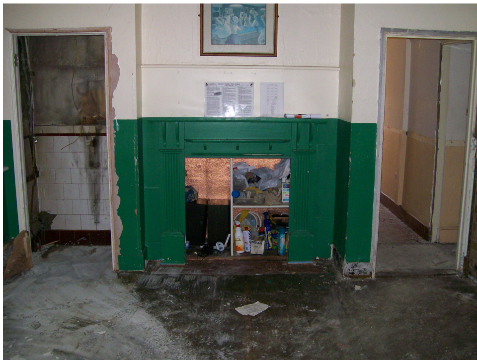
Appendix Plate 17 The “backroom” detail of fireplace and original tiling.
