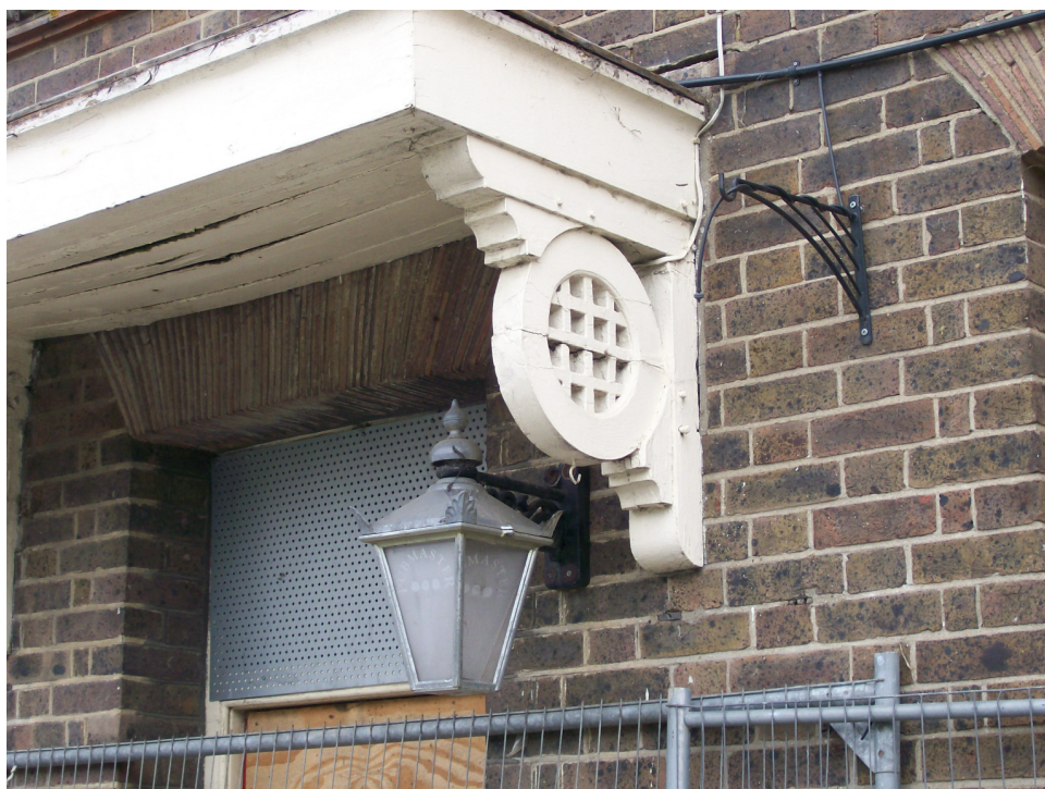
Appendix Plate 2 Detail of porch brace on south elevation.
