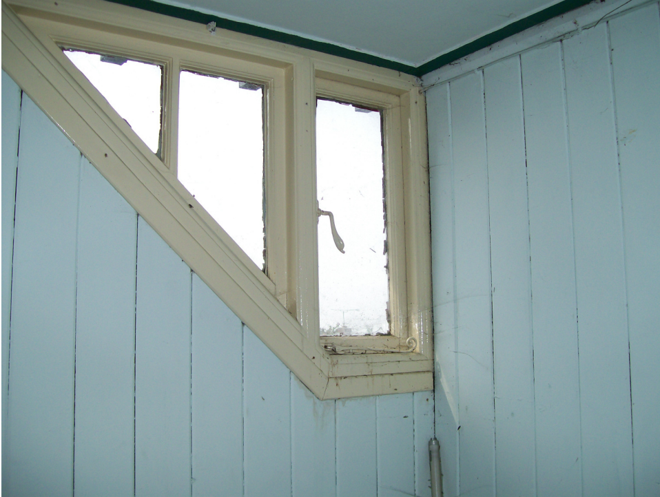
Appendix Plate 21 Detail of lights west side of north dormer.
