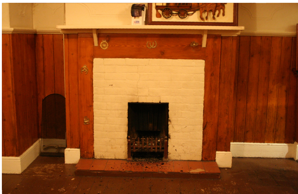
Appendix Plate 15 The fireplace in the saloon bar.
