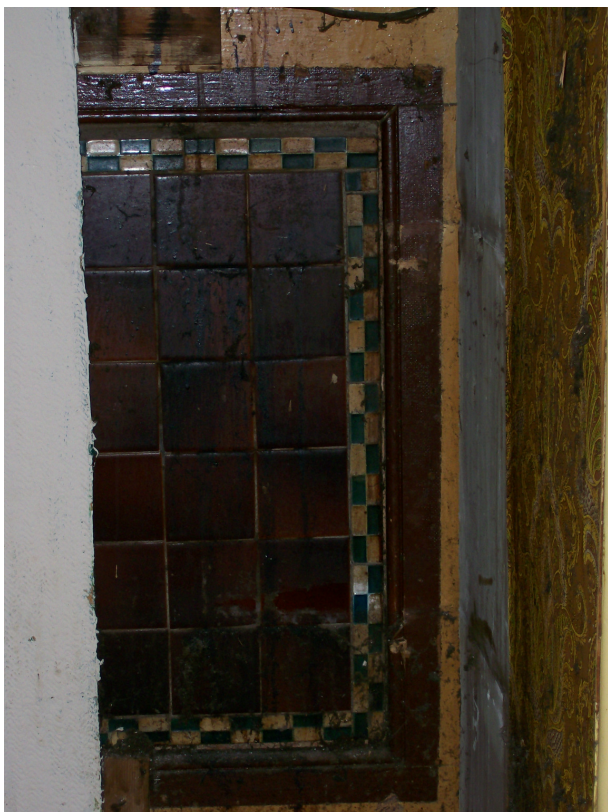
Appendix Plate 11 Detail of original wall tiles in lounge bar.
