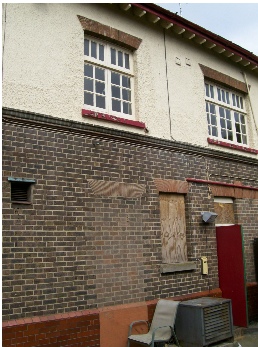
Plate 5 The east elevation showing the blocked door and window.
