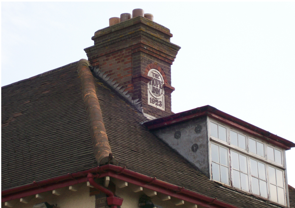
Plate 2 Glazed plaque showing date of construction.
