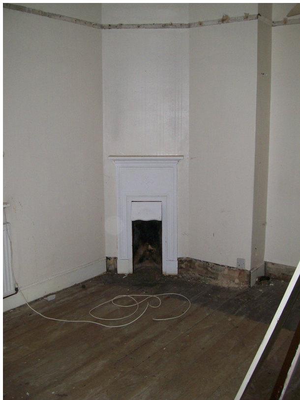
Appendix Plate 19 Fireplace in northwest bedroom, first floor.
