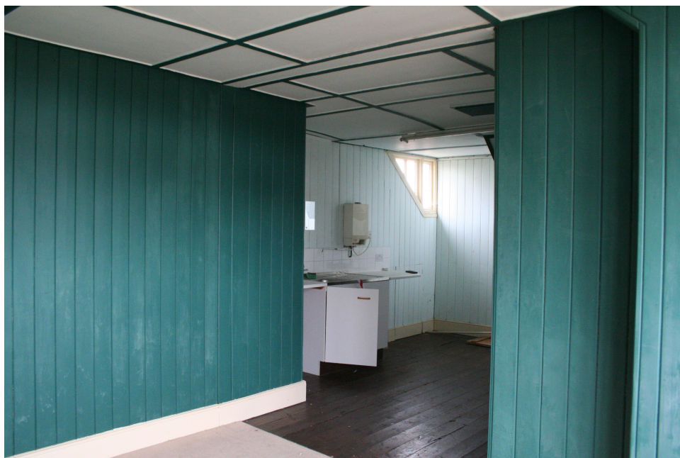
Appendix Plate 20 East attic showing removed dividing wall to north attic.
