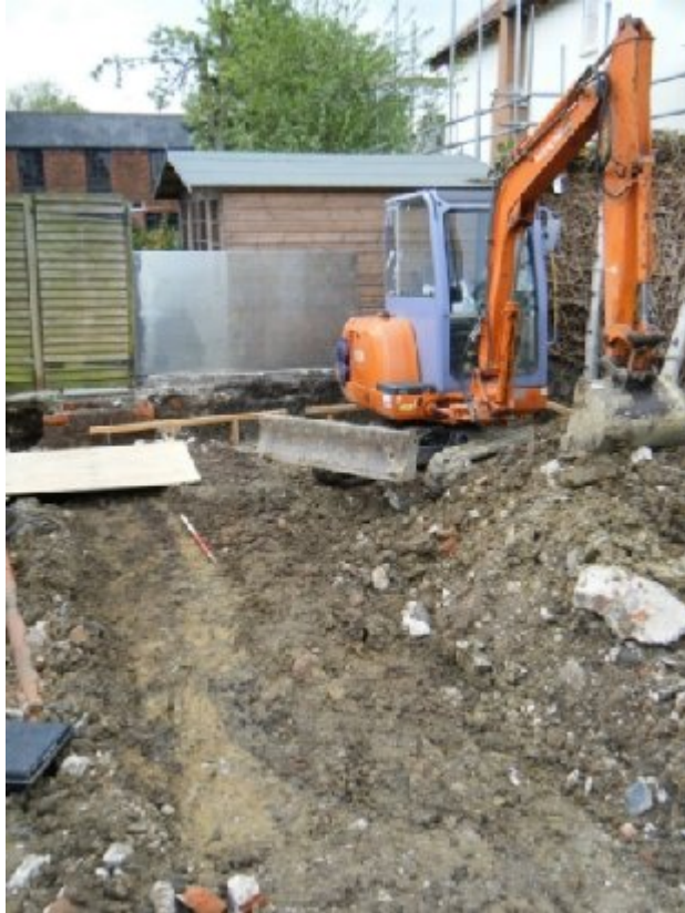
Plate 1: general view of site looking SW
