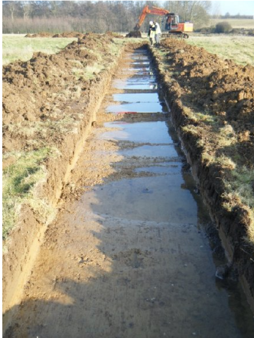
Plate 1: Trench 4, view east, showing typical ground conditions
