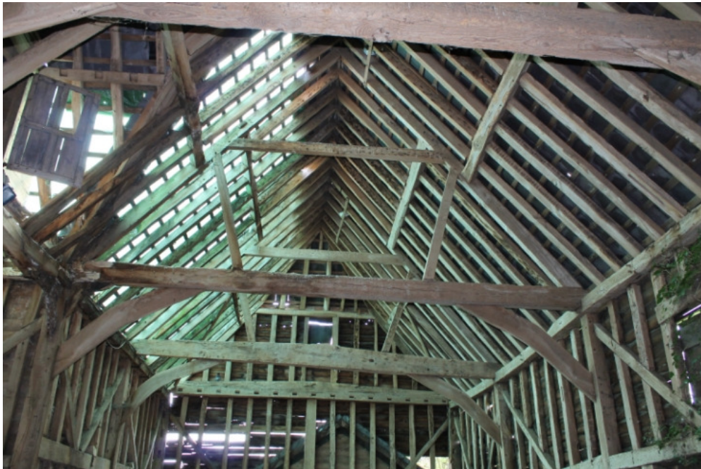
Plate 26 Barn 3a detail of roof truss – view south
