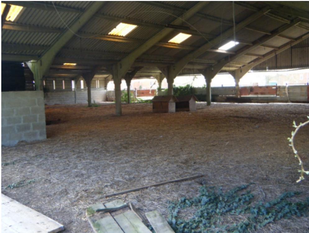
Plate 40 Interior of covered livestock pen 6 – view south-east
