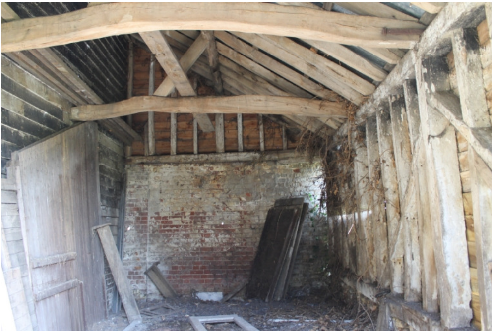
Plate 10 Interior of lean-to 1f, showing the timber frame and lightly-cambered bridging beams – view north-east
