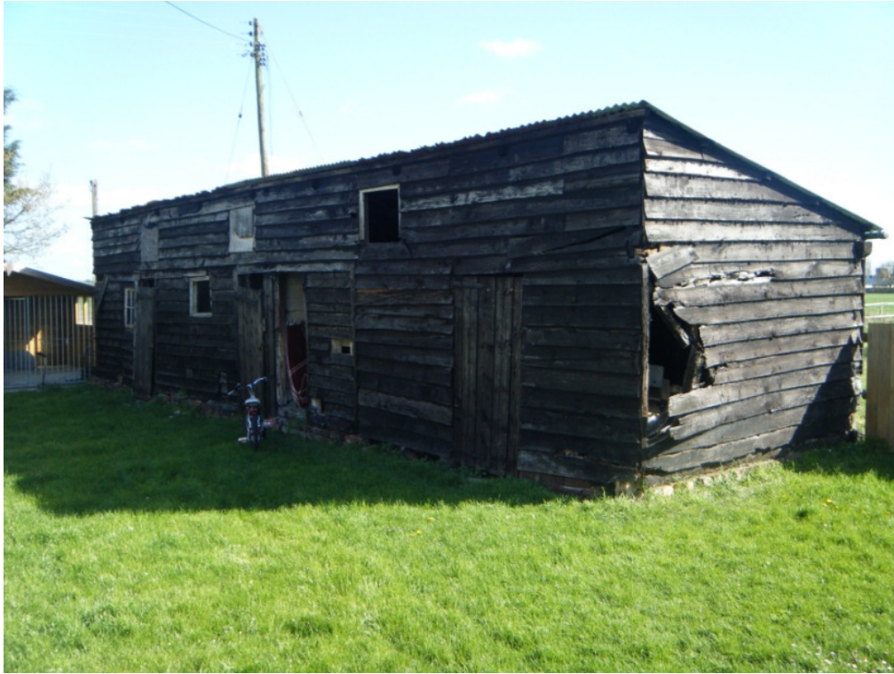
Plate 43 Structure 10, former poultry house – view north
