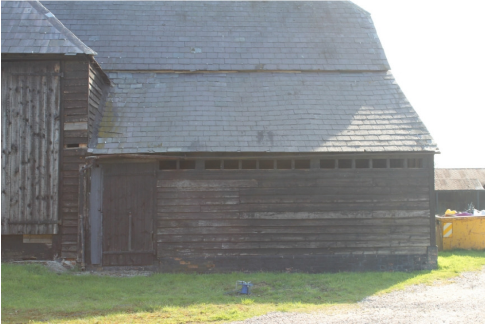
Plate 7 Lean-to 1d, showing infilled open front – view north-east
