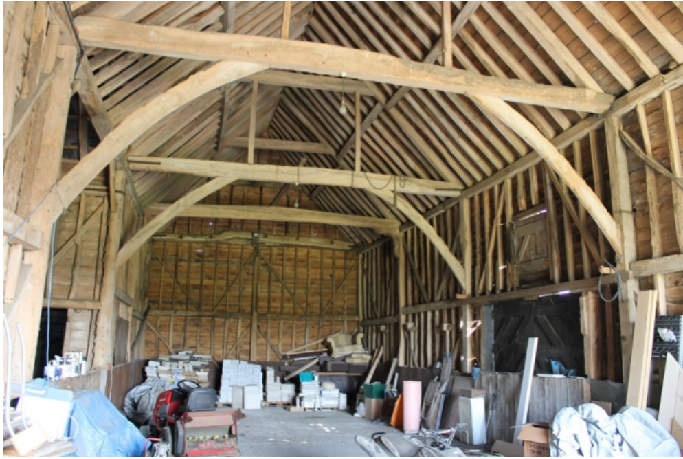
Plate 3 Interior of barn 1a – view north-west
