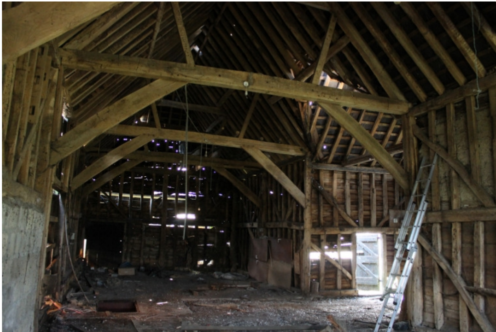
Plate 12 Interior of barn 2a - view west
