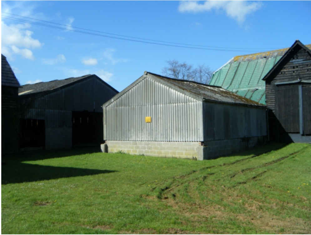
Plate 39 Structures 6 and 7, covered livestock pens – view south-west
