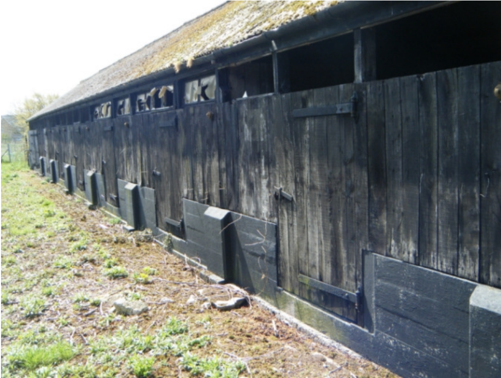
Plate 41 Structure 8, stable block – view south-west
