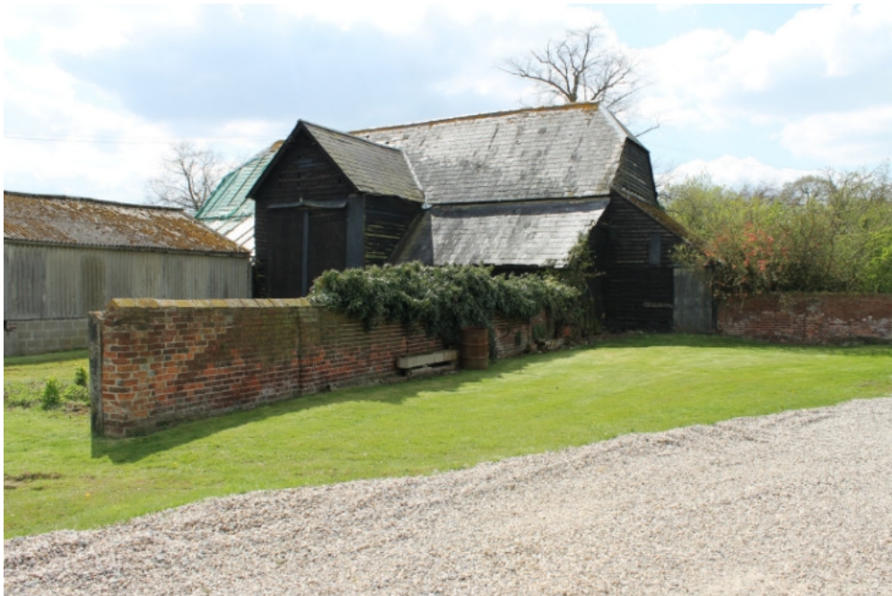
Plate 20 Structure 3 – view south-west
