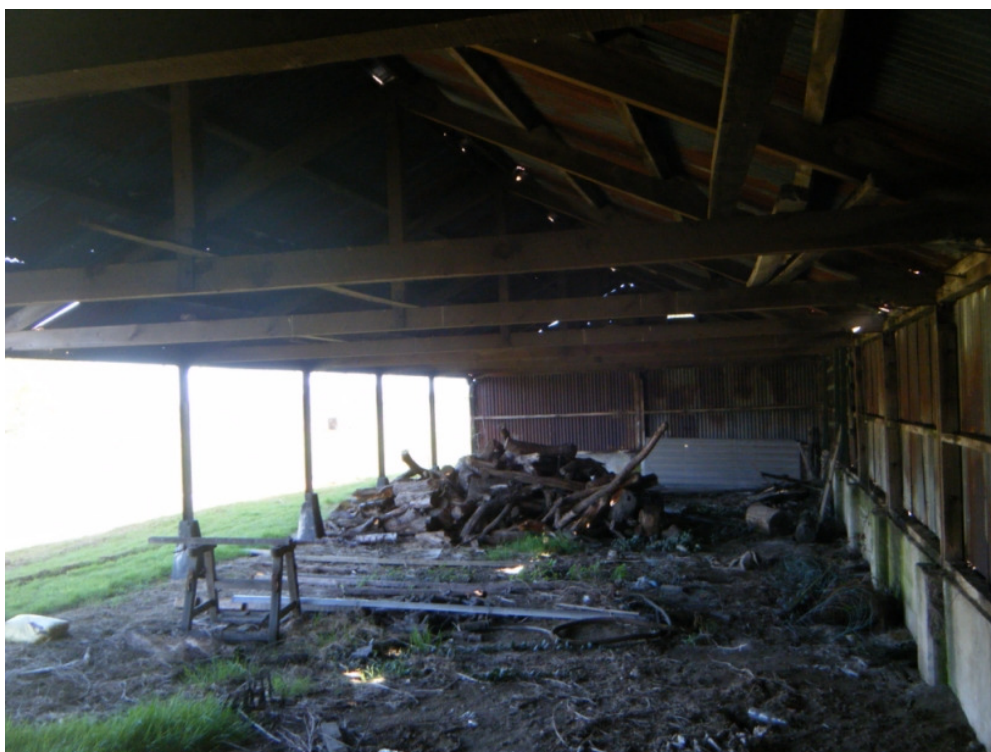
Plate 38 Structure 5, interior of cart lodge – view north
