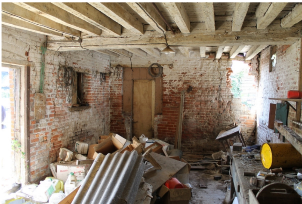
Plate 37 Interior of stable 4a – view south-west
