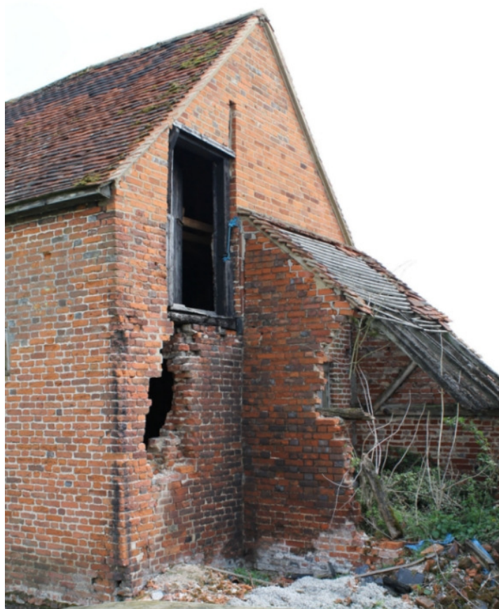
Plate 36 Stable/granary 4a with lean-to 4b and elevated doorway to granary loft – view east
