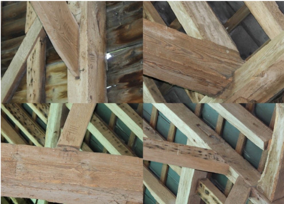
Plate 30 Barn 3a, examples of carpenters' marks on trusses
