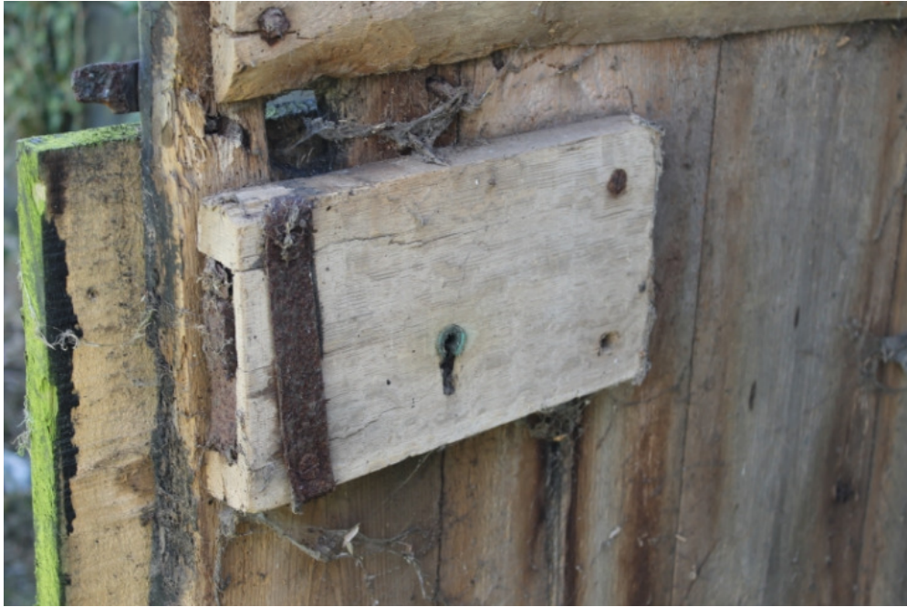
Plate 19 Detail of original lock housing on door to granary 2c
