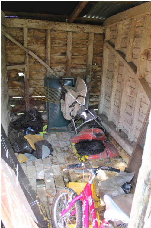
Plate 44 Interior of structure 10, showing timber frame and brick floor - view north-east
