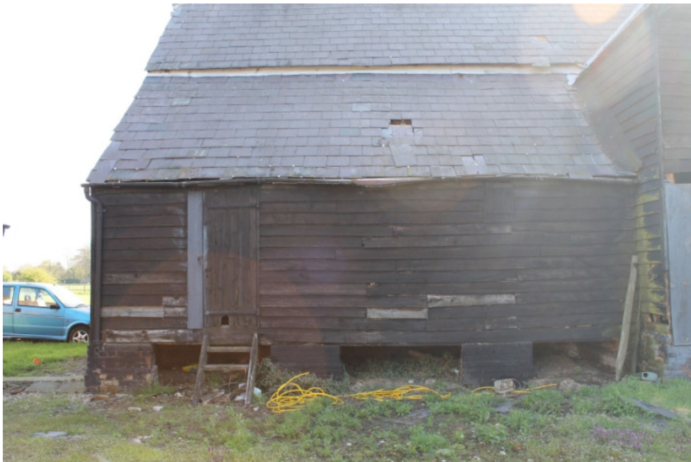
Plate 6 Granary 1b/c – view north-east
