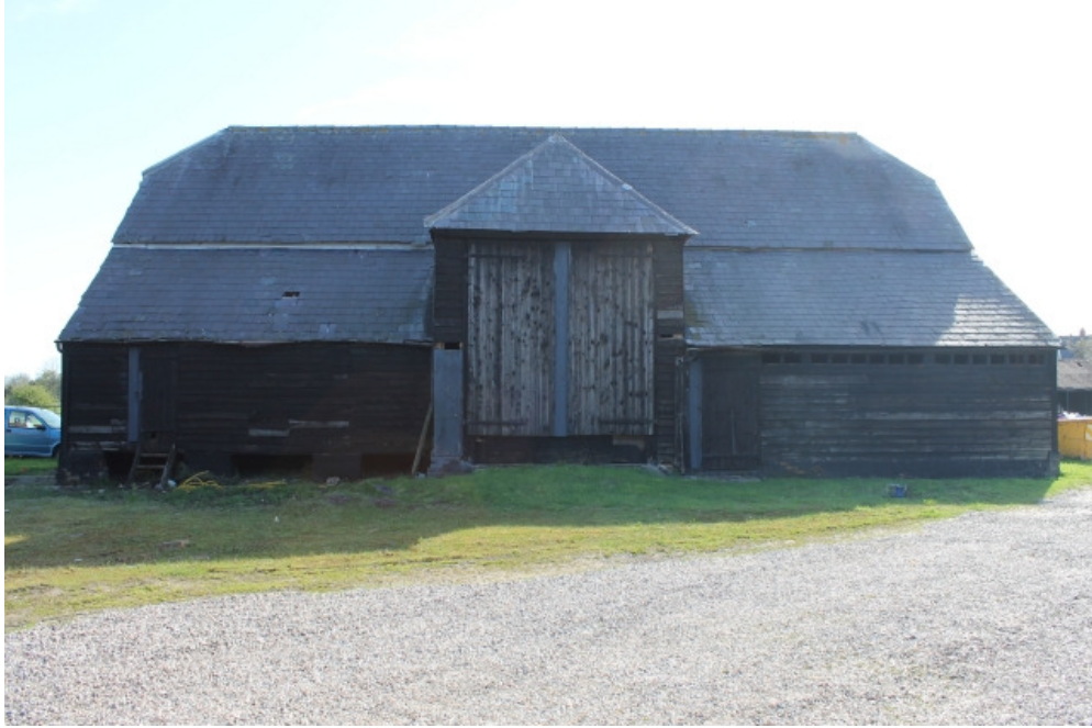
Plate 1 South-west elevation of structure 1, with granary 1b/c to the left, the midstrey of barn 1a and lean-to 1d to the right - view north-east
