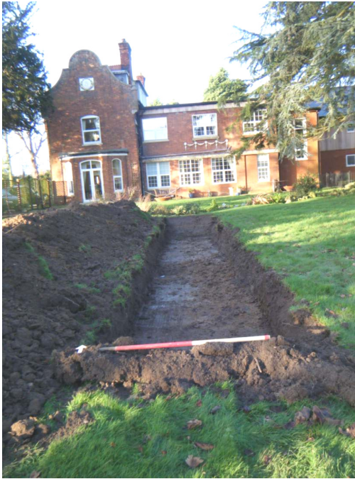
Plate 2: T3, view north towards Hall
