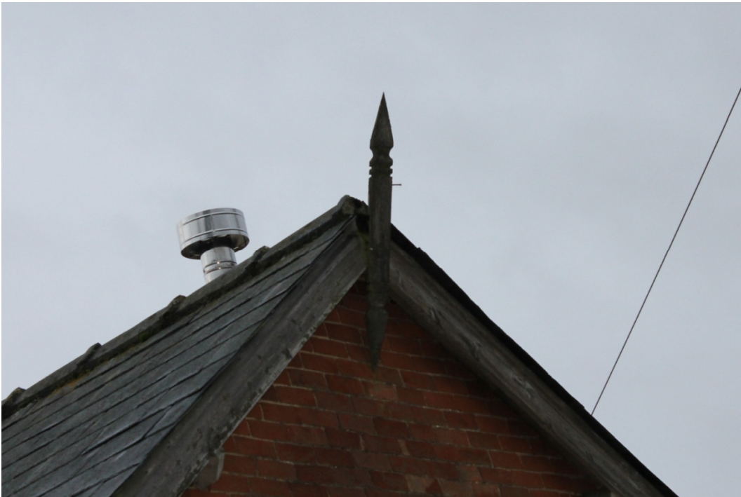
Plate 2 Turned finial on apex of north-west gable – view south-west
