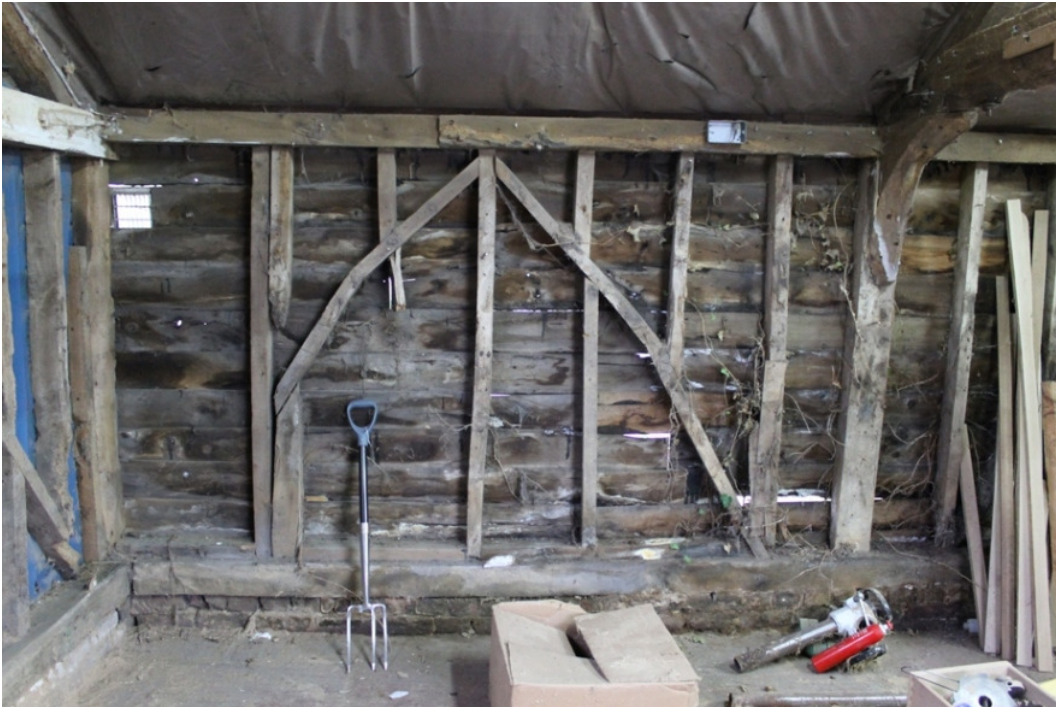
Plate 13 Former loose box, timber framing of bay 3 with arched primary bracing and scarf joint in wall plate – view north-west
