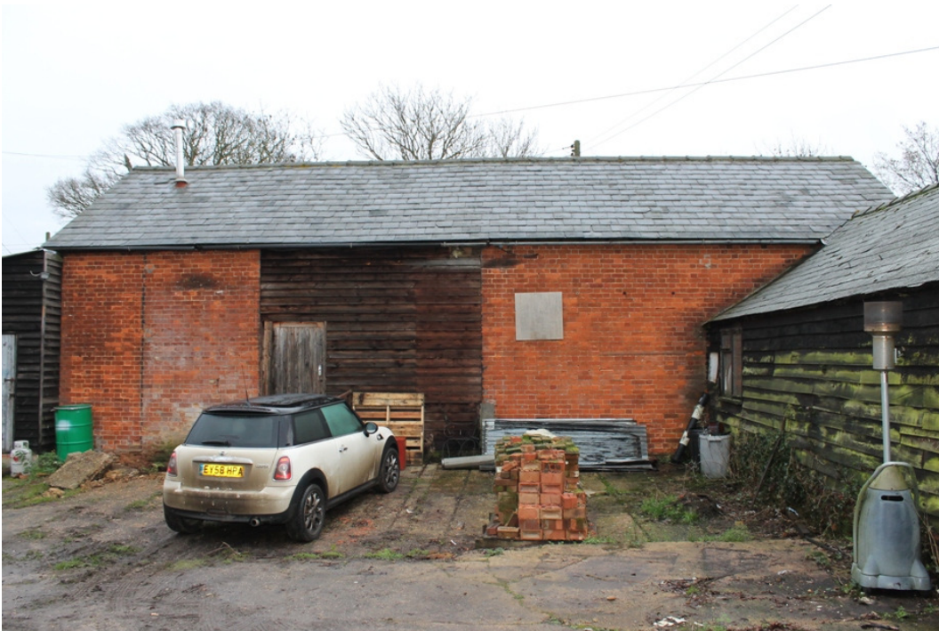
Plate 4 South-west elevation of the barn, with the blocked cart door opening – view north-east
