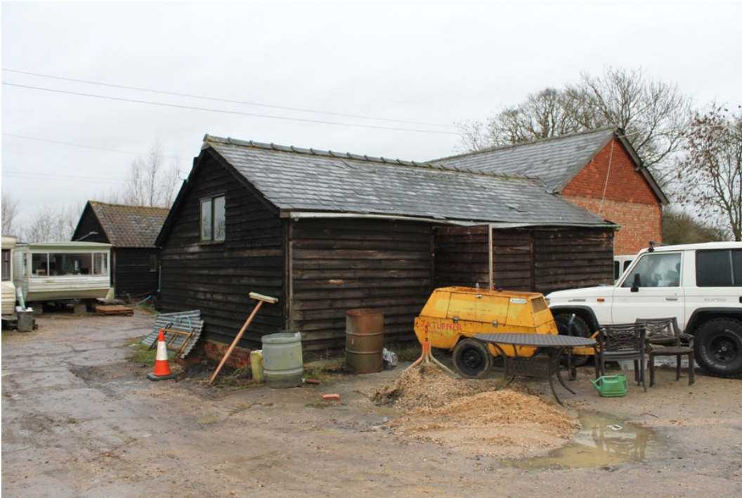
Plate 11 Former loose boxes, showing the asymmetrical roof and the blocked openings that would have faced the yard – view north
