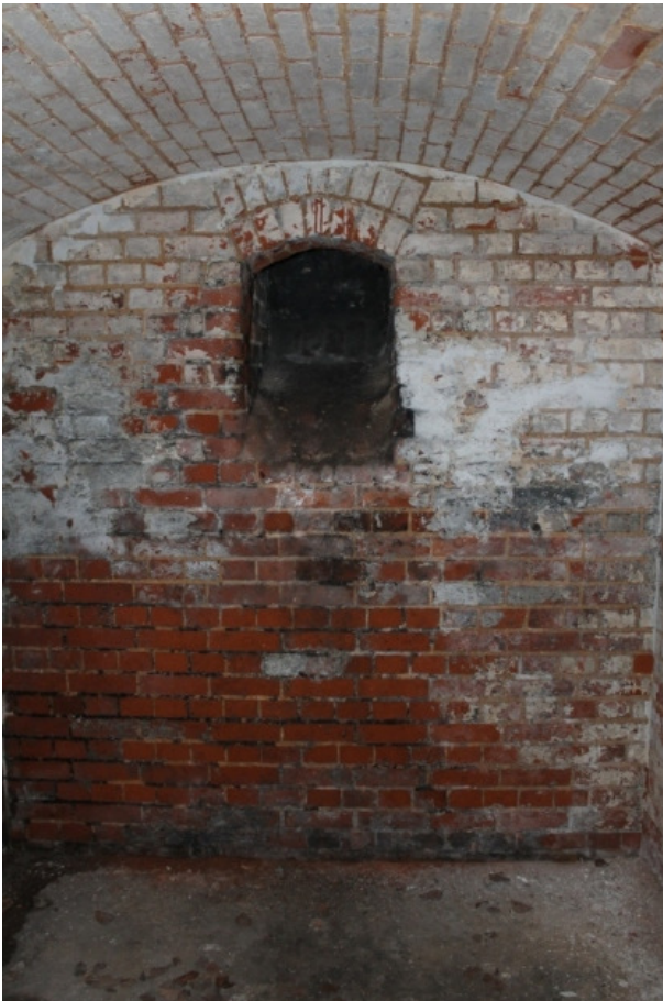
Plate 40 Room 34, the brick vaulted coal store with the original coal chute – view north-east
