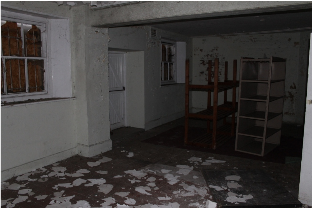
Plate 44 Rooms 39 and 38, the former kitchen and mess manager's room, with the dividing wall removed and a doorway inserted through one of the windows of the mess manager's room – view south
