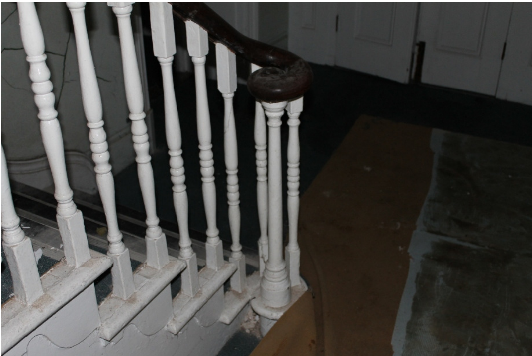
Plate 16 Stairwell iv , detail of the mahogany banister with spiral end and the turned balusters of the open string staircase
