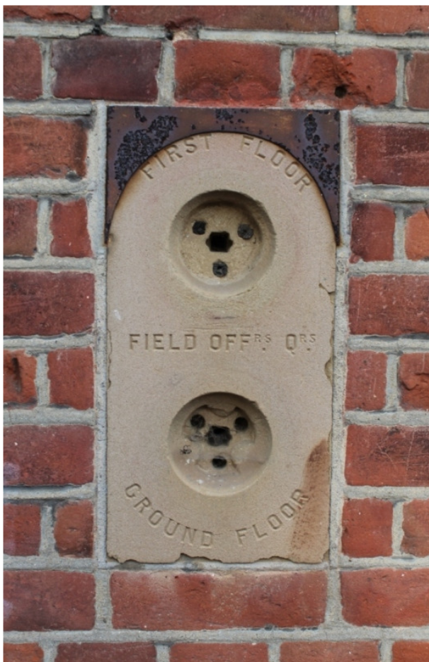
Plate 7 Detail of the sandstone block housing the bell pulls to the Field Officers' Quarters on entrance way i
