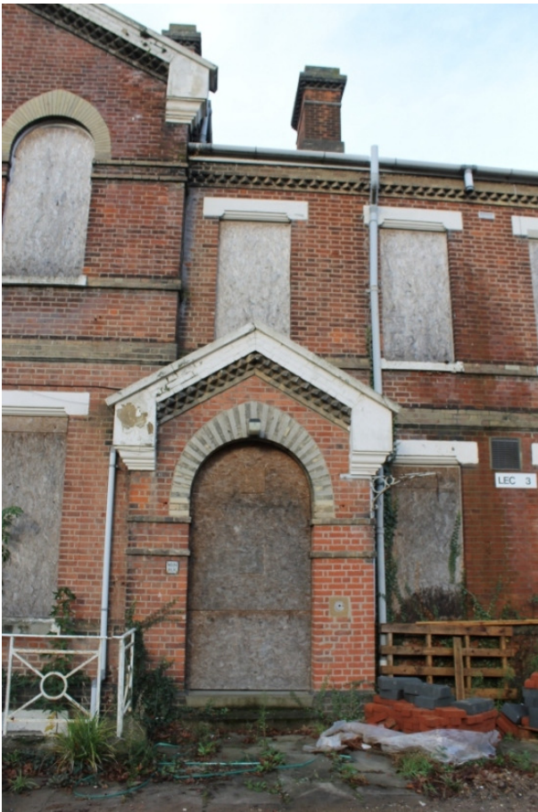
Plate 4 Entrance way iii , showing the projecting gabled porch with the yellow stock brick embellishments, sandstone bell pull and iron bracket for gas lamp – view north-west
