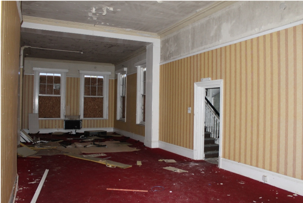
Plate 25 The mess room with the 1922-62 extension to the rear and the original doorway to the servant's stairs in the right-hand wall – view north
