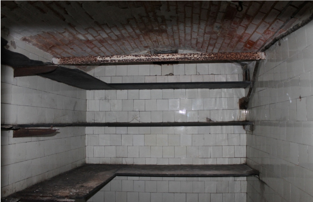
Plate 43 Room 31, the larder with the original glazed wall tiles and slate shelving – view north
