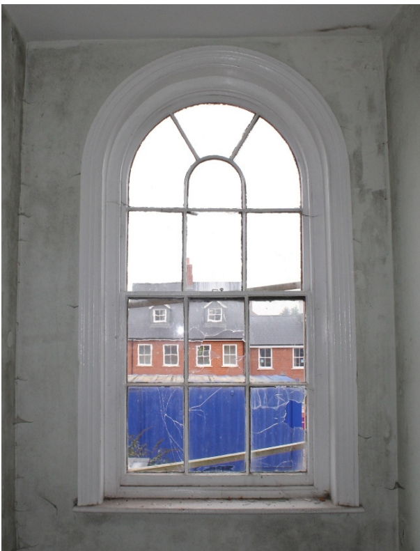
Plate 30 Example of the Italianate sash windows found in rooms 18-21
