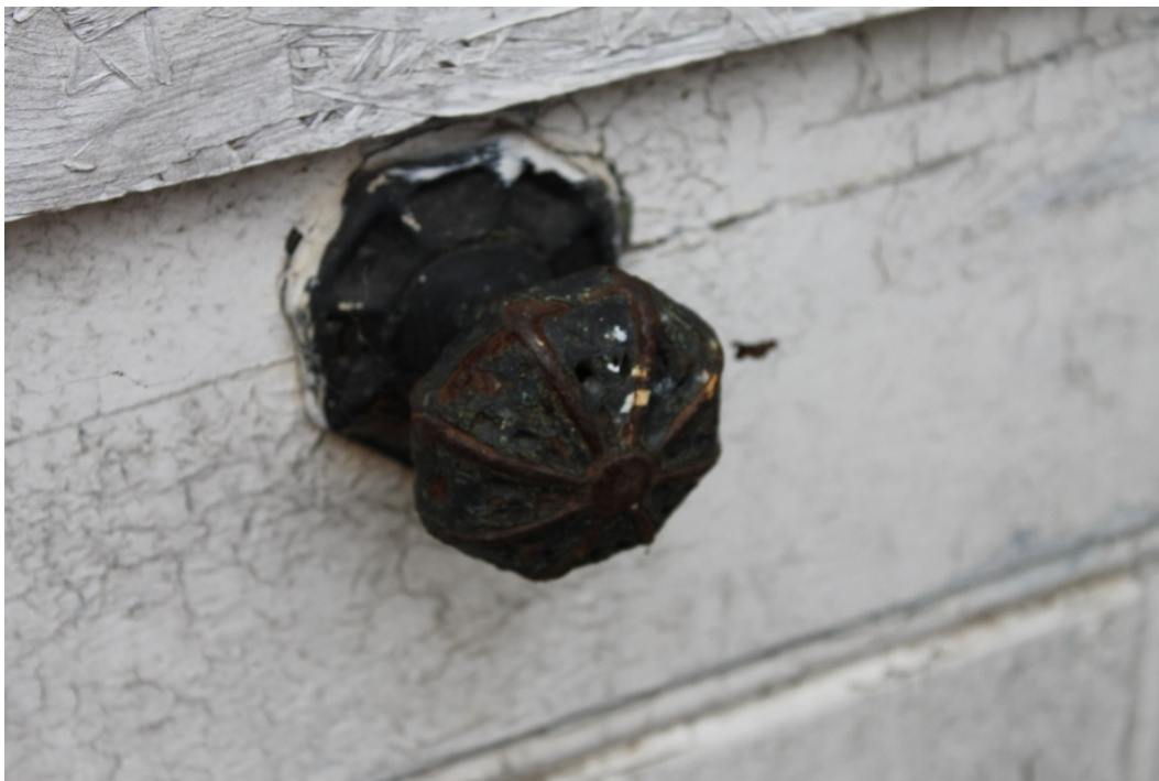
Plate 5 Detail of the original door knob on the entrance way doors
