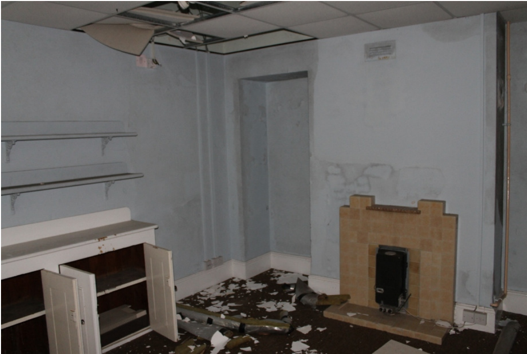
Plate 31 Room 18, formerly quarters for the servants of Officers Nos.1, 6 and 7, showing the bricked-in original doorway to the left of the chimney breast and the double-width dresser on the dividing wall – view south
