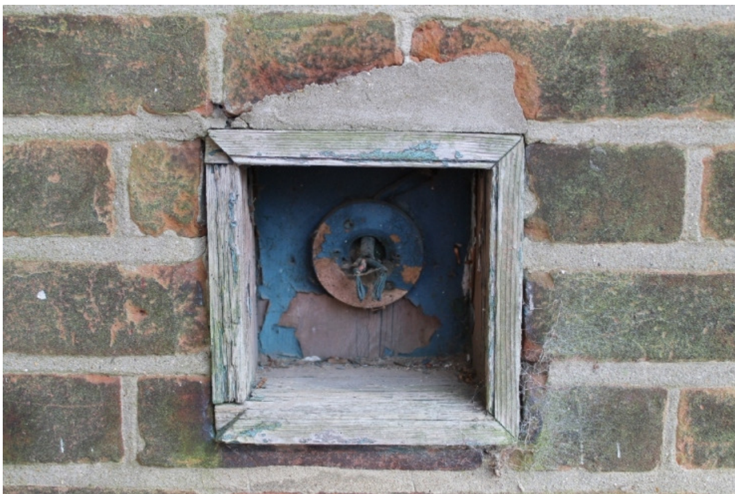
Plate 8 Detail of the wooden housing for electric door bell to the 1904 extension, inserted into the side wall of entrance way i
