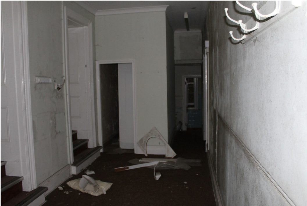
Plate 35 The converted landing of the former stairwell iii , with the inserted shower room, the 1904 ablution block to the rear and the original doorways to the servants' quarters in the left-hand wall – view north-west
