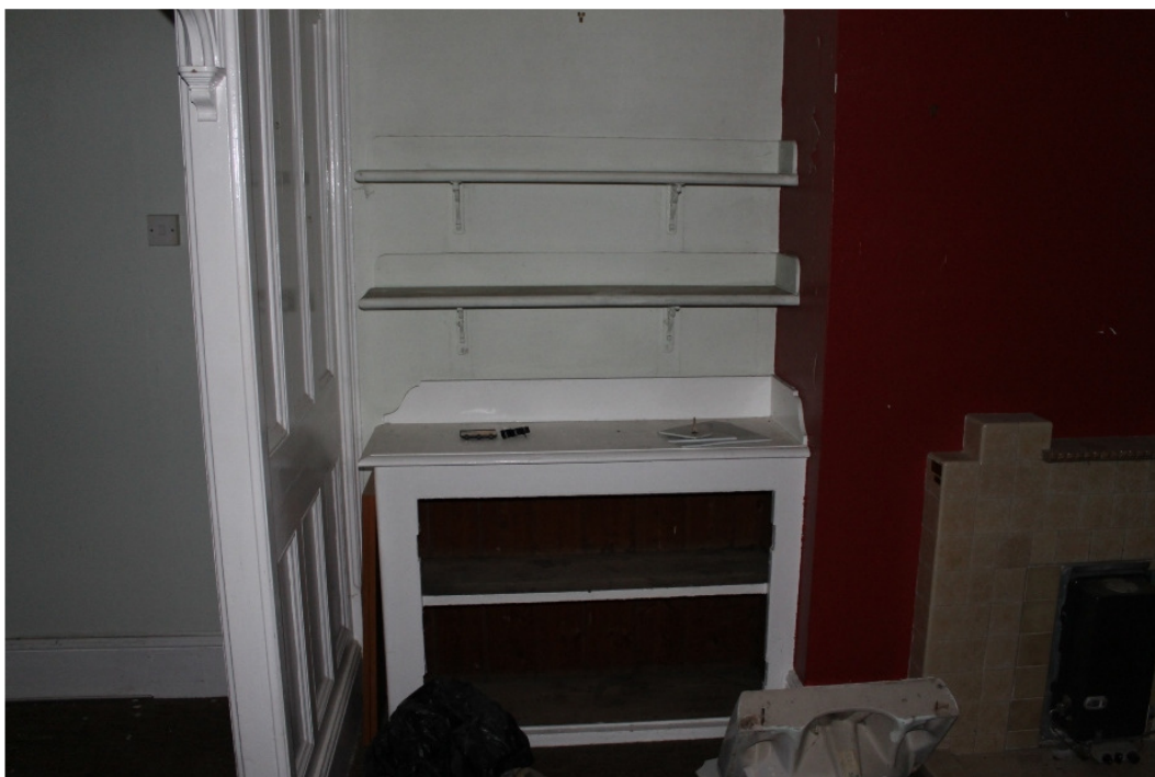
Plate 20 Dresser and shelving in room 2, either relocated from the 1876 rooms or faithfully reproduced – view north-west
