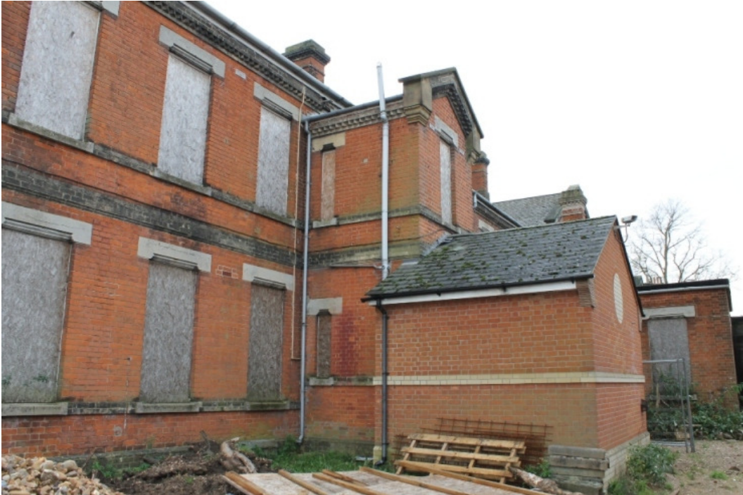
Plate 11 The north-west elevation showing the 1904 extensions, with the additional officers' accommodation to the left, the projecting ablution block and the 1980s toilet block – view south
