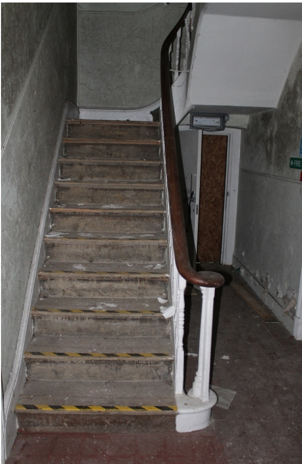
Plate 38 Stairwell v, the basement stairs with the same mahogany banister with spiral end and turned balusters as the staircases of the entrance ways – view north-west
