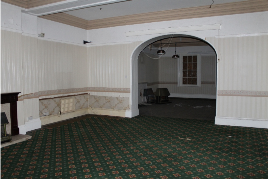
Plate 27 The 1904 bar converted from the quarters for Officers Nos.2 and 3, with the extension through the archway and the inserted fireplaces on the left-hand walls – view west
