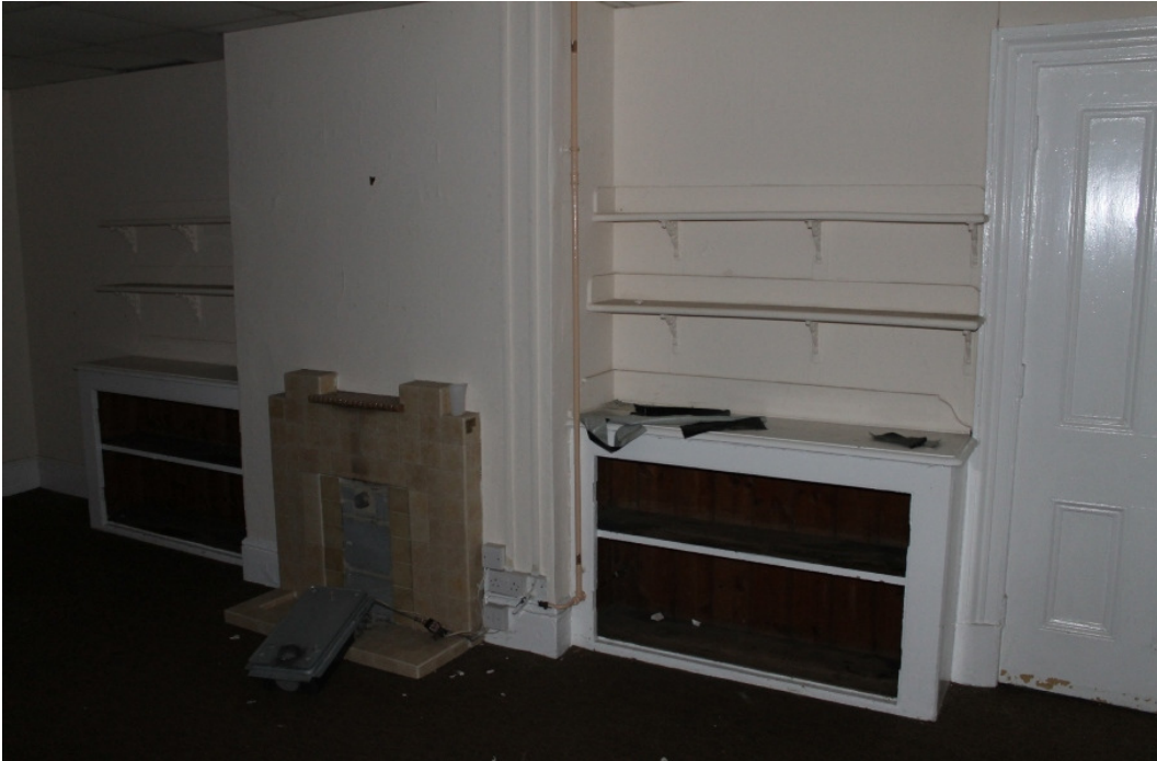
Plate 23 Room 4, formerly the sitting room of the second Field Officer, with the original four-panel door leading to the bedroom of said officer – view west
