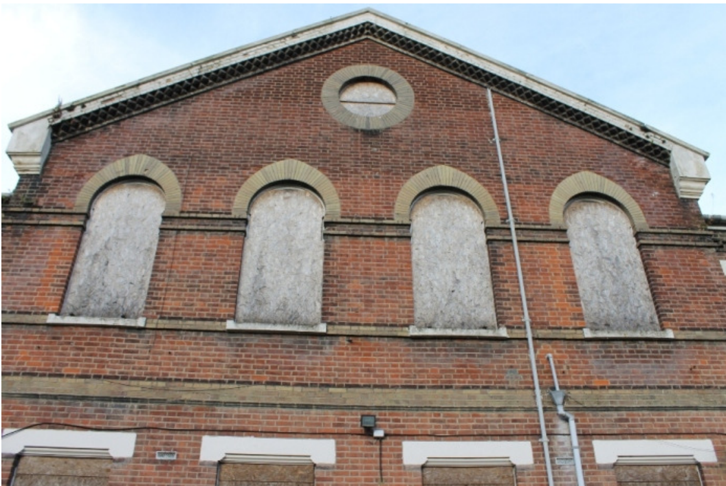
Plate 2 Central projecting gabled section of south-east elevation, showing the pointed arches of the first floor windows and the oculus above – view north-west
