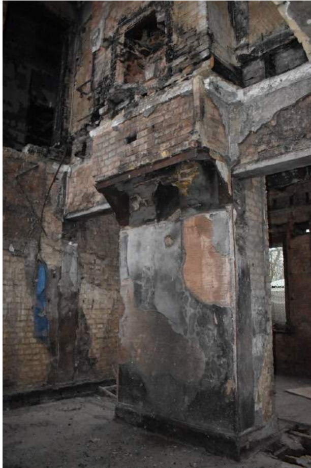
Plate 27 Chimney with removed fireplace below room 24 - view east.
