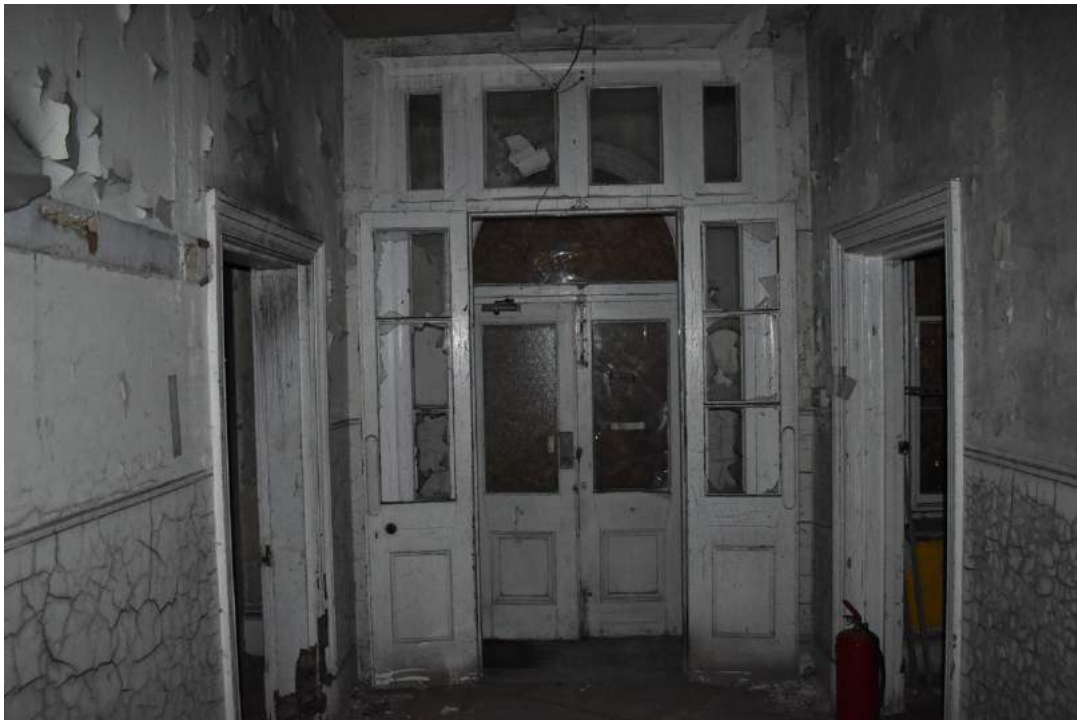
Plate 1 Entrance way ii, showing the original inner and outer doors of the porch and original coat hooks on the left wall - view south-east. Photo from November 2013 above, photo from December 2019 below.
