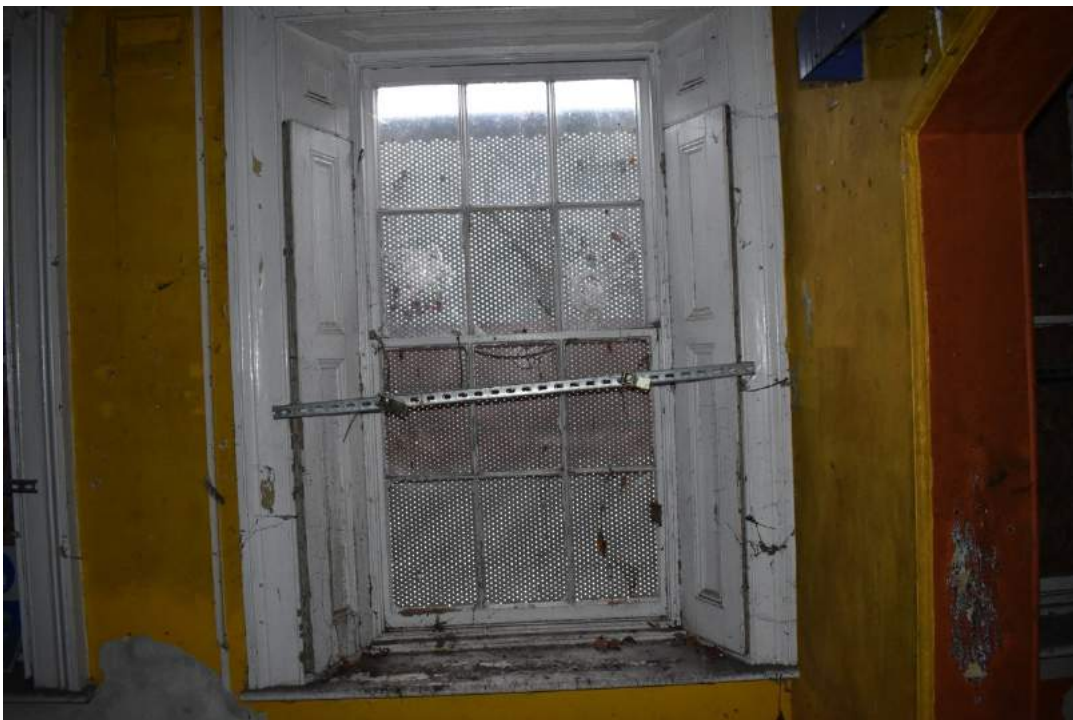
Plate 7 Example of the sash windows with recessed wooden shutters in the ground floor rooms of the 1874-5 building - view south-east. Photo from November 2013 above, photo from December 2019 below.
