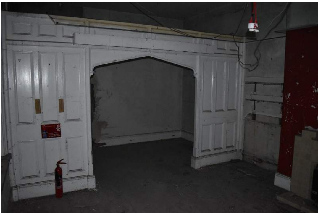
Plate 5 Original wooden partition in room 2 separating the sleeping area from the sitting room – view south-west. Photo from November 2013 above, photo from December 2019 below.
