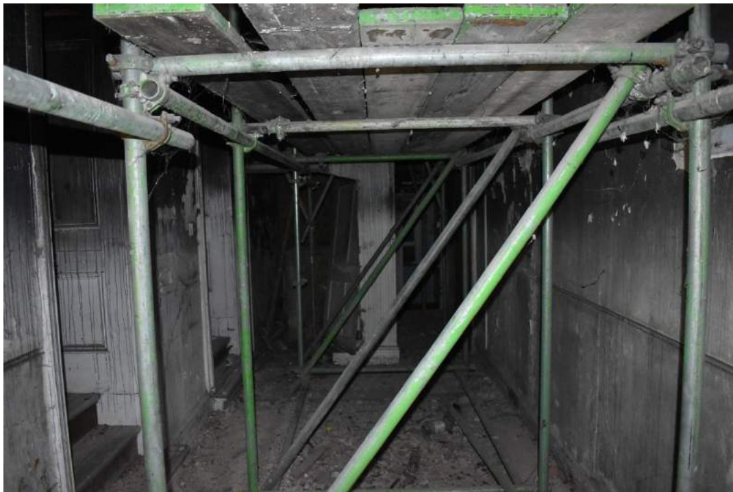
Plate 19 The converted landing of the former stairwell iii , with the inserted shower room, the 1904 ablution block to the rear and the original doorways to the servants' quarters in the left-hand wall – view north-west. Photo from November 2013 above, photo from December 2019 below.
