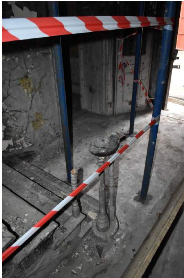
Plate 3 Stairwell iv, detail of the mahogany banister with spiral end and the turned balusters of the open string staircase. Photo from November 2013 above, photo from December 2019 below.
