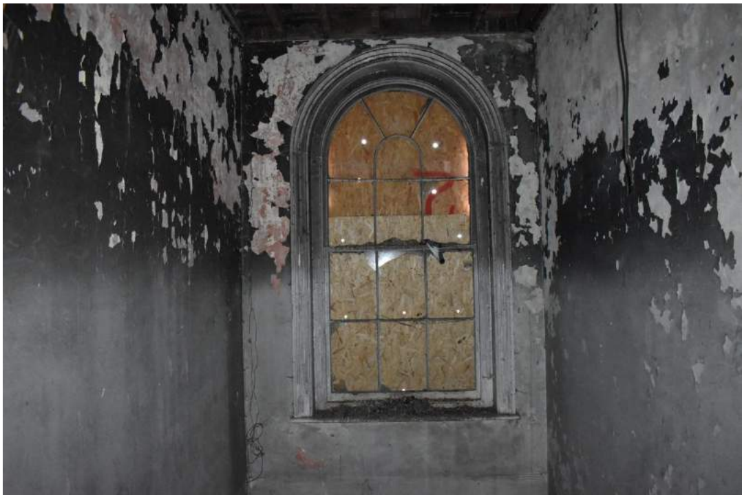
Plate 15 Example of the Italianate sash windows found in rooms 18-21. Photo from November 2013 above, photo from December 2019 below.
