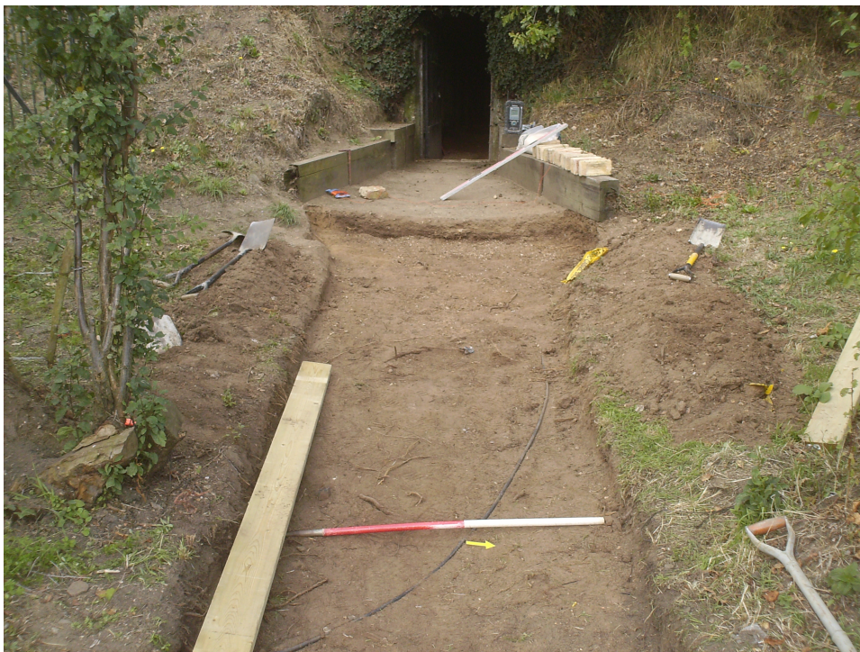
Photo 2 Stripped area for access path, viewed from the east.
