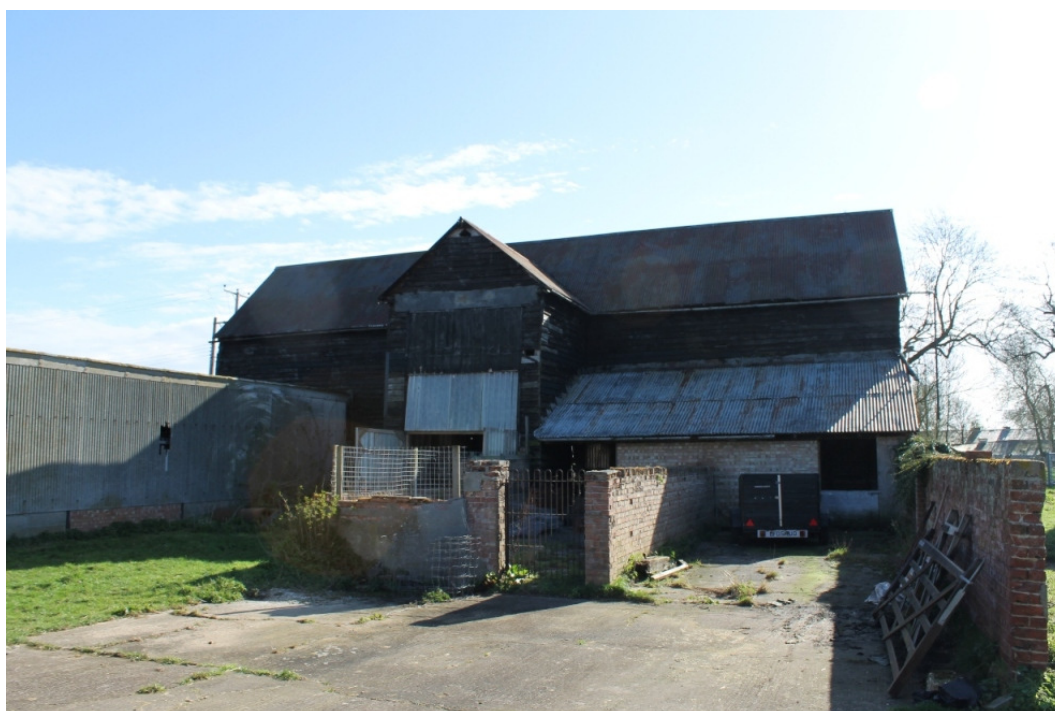
Plate 1 North-west elevation of the barn - view north-east
