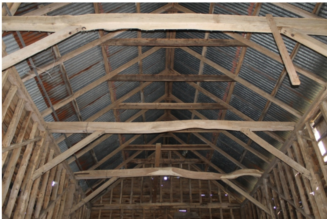
Plate 9 The original tie-beams with the replacement roof above - view north-east.
