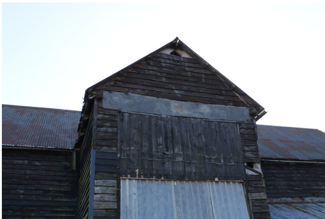
Plate 3 Surviving portion of the full-height barn doors in the midstrey - view south-east
