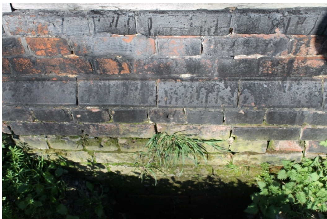
Plate 2 Detail of the brick plinth, with Flemish bond above the chamfered course and English bond below
