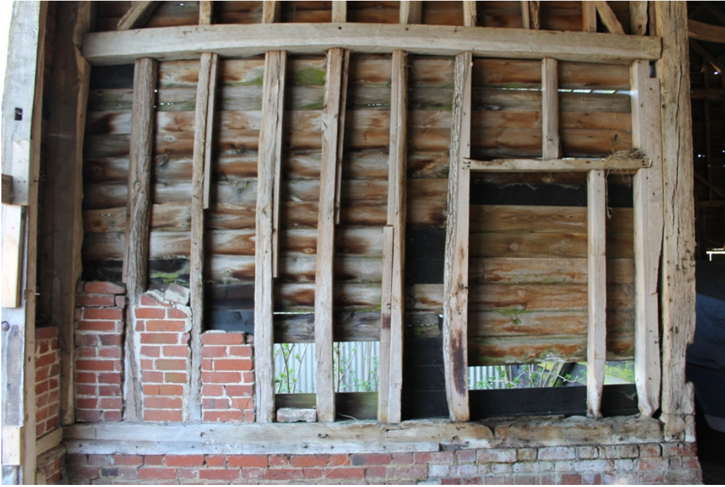
Plate 13 Remains of brick nogging between studs of midstrey wall - view north-west
