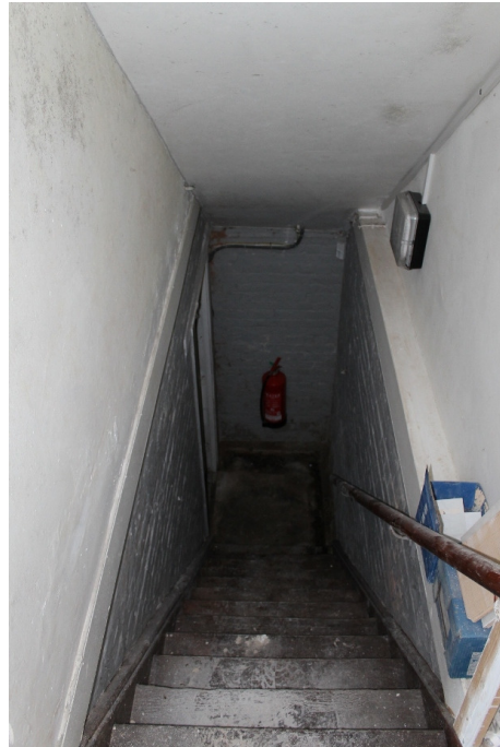
Plate 7 Internal staircase to basement of Spurrier's House - view north-west
