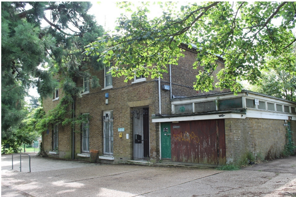
Plate 11 Spurrier's House with 1960s toilet block attached - view south-east
