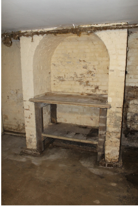
Plate 8 Original brick alcove in basement of Spurrier's House – view south-east
