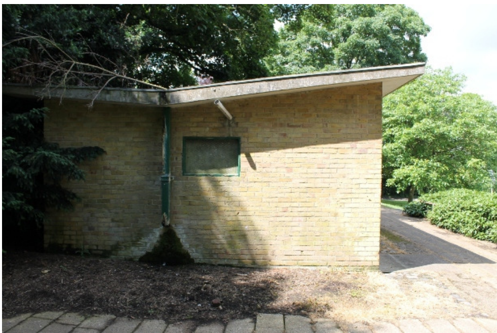
Plate 35 The Greyhound toilets with the integrated roof drainage - view west
