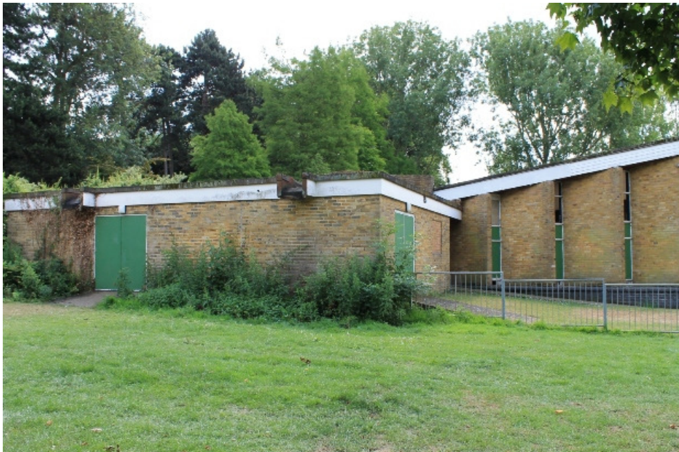
Plate 31 The ancillary structure at the side and rear of the Bandstand, housing the green room and dressing rooms – view south-east
