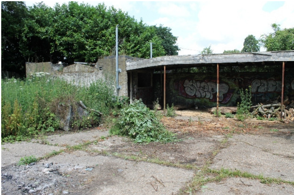
Plate 33 Remains of the gardener's office and an open-fronted shed in the Nursery - view north-west
