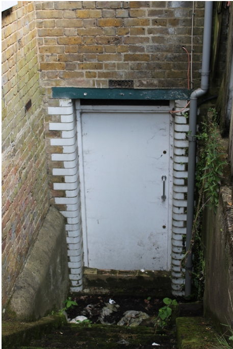
Plate 6 Basement entrance to Spurrier's House - view south-east
