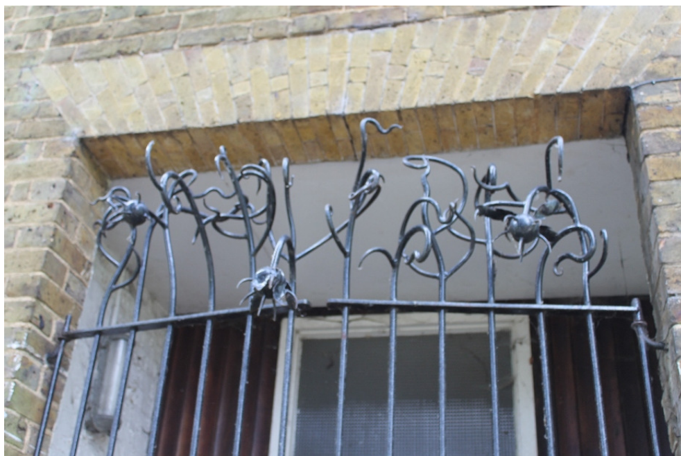
Plate 2 Detail of wrought iron security bars in the shape of seed pods - view south-east
