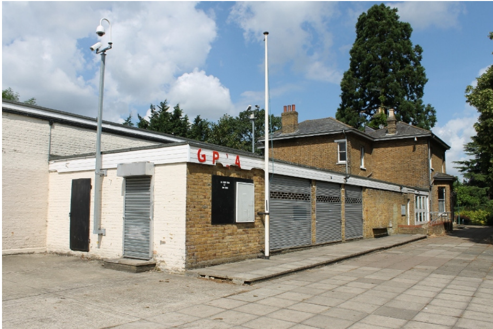
Plate 16 Spurrier's Core with Spurrier's House to the right and the cafe extensions - view south
