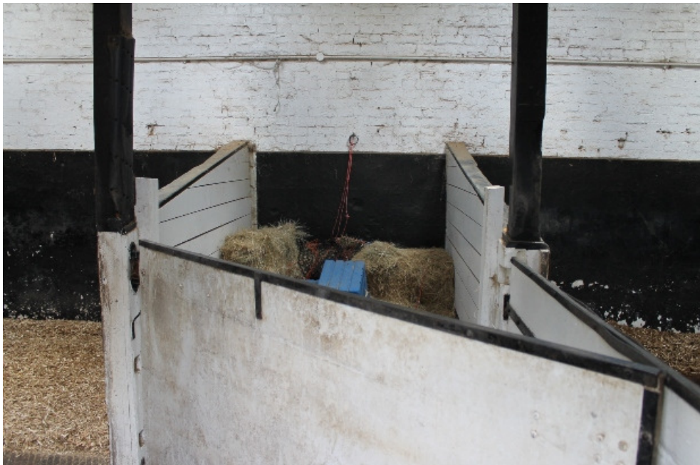
Plate 21 Original stall dividers in the stable block - view north-east
