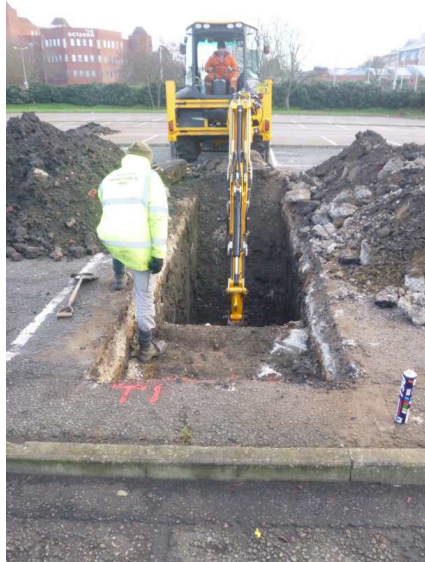
Plate 1: TP1 under excavation
