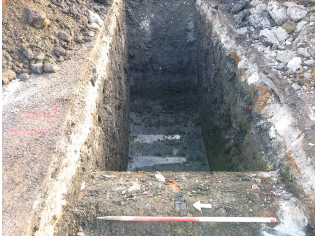
Plate 2: TP1 fully excavated.
