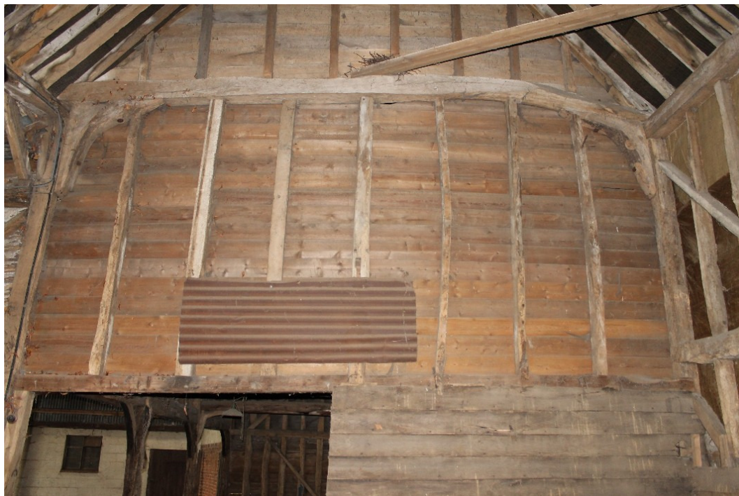
Plate 13 Inserted dividing wall between bays 3-4 of the Church Barn - view south-west
