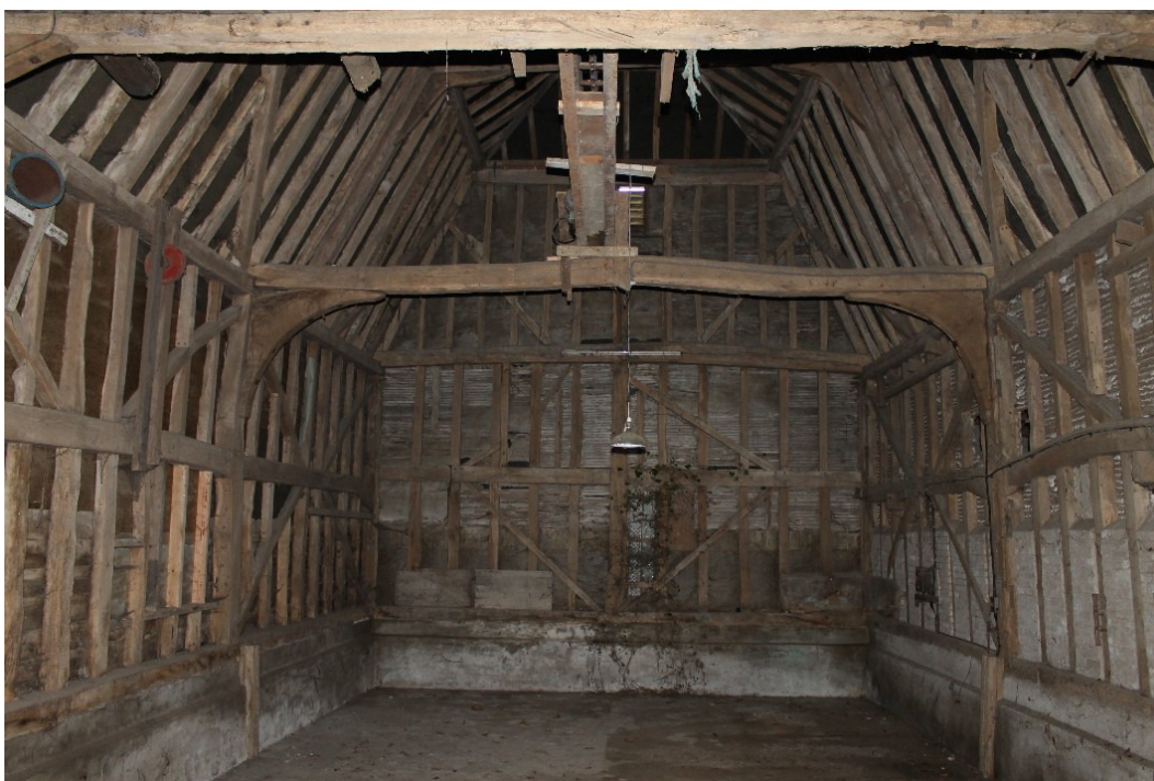
Plate 4 Interior of the Grain Barn - view north-west
