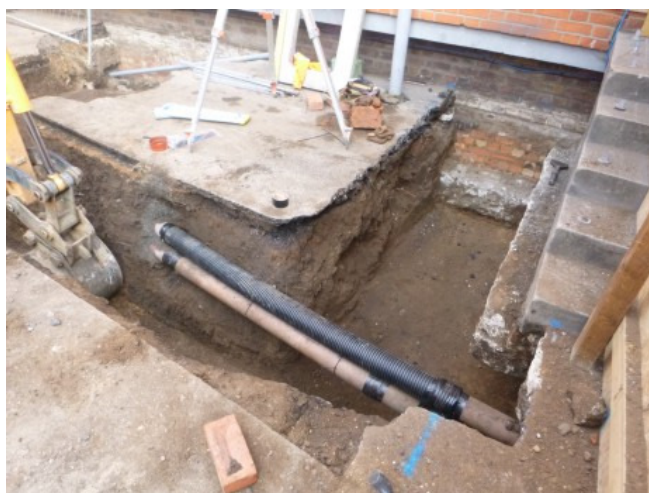
Photograph 8 Foundation trenches for gym extension
