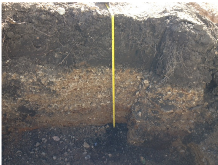
Photograph 5 Section through road surface F1
