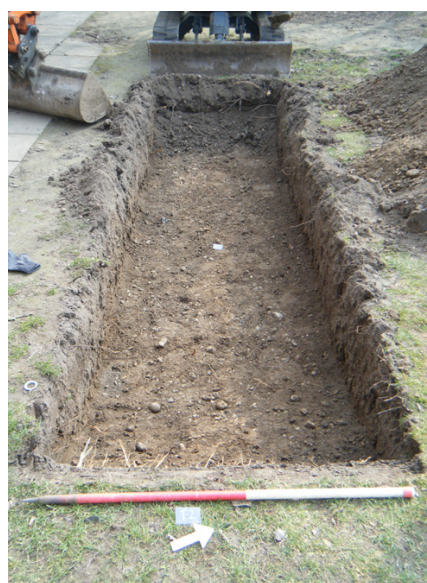
Plate 2: T2, view north-west.
