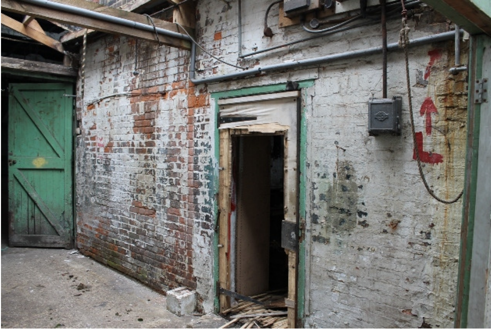
Plate 3 South elevation of the converted 1830 house, showing the inserted doorway and blocked windows – view north-west
