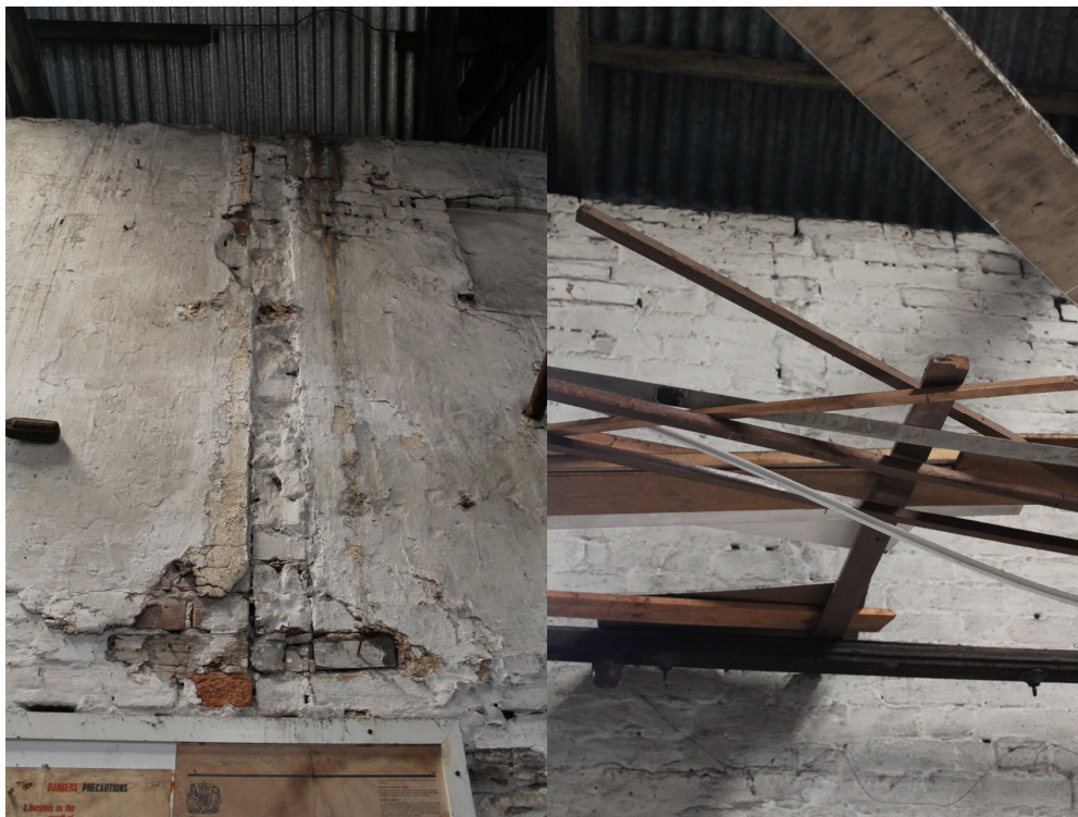
Plates 7 and 8 Evidence for the removed dividing wall in the converted 1830 house
