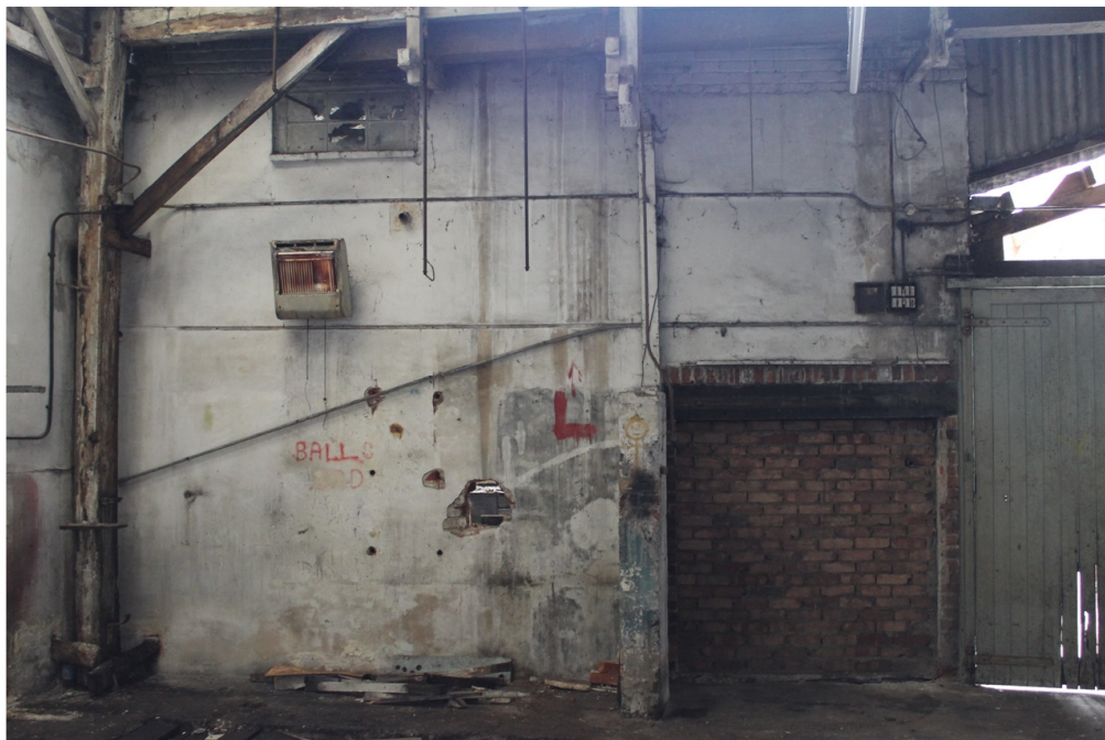
Plate 5 The replacement west wall of the converted 1830 house - view east
