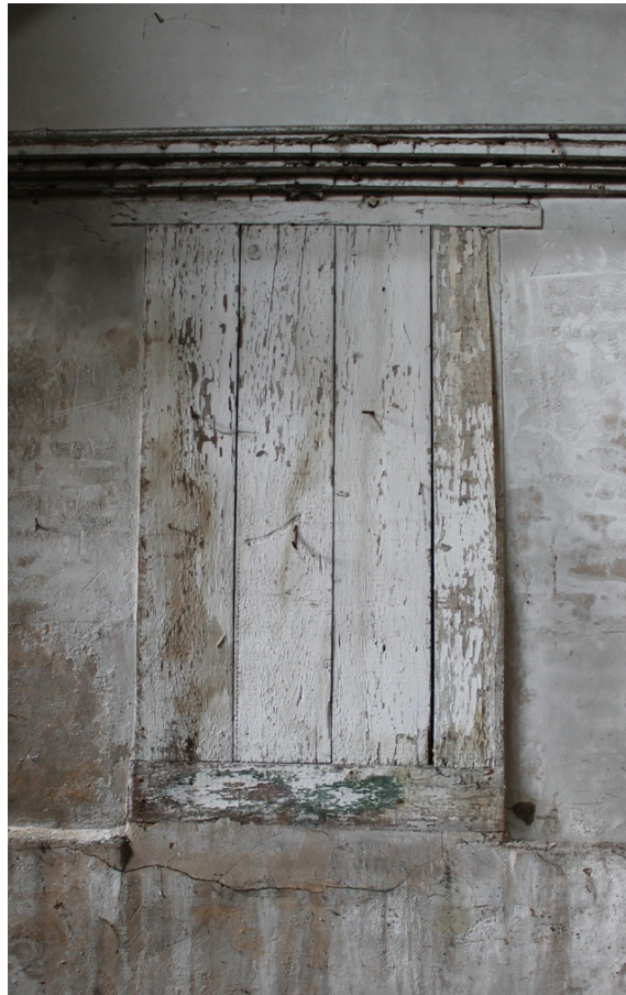
Plate 11 Possible entrance from former Cups Hotel stables into workshop – view north
