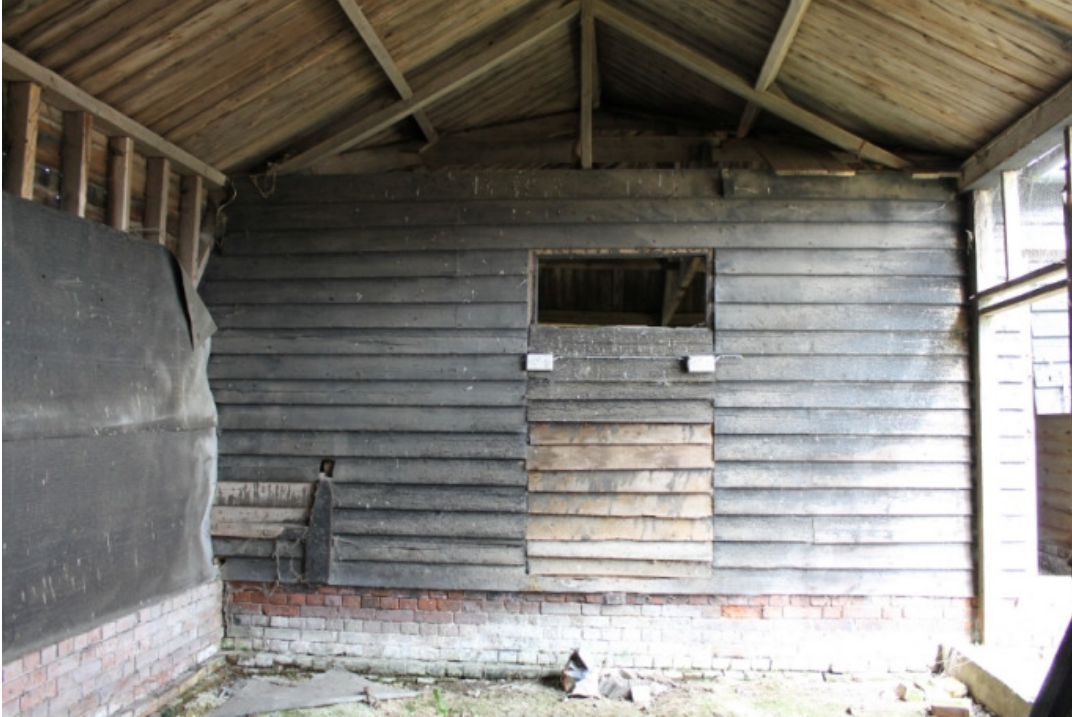
Plate 22 Interior of the 'four-bayed' cattle shed showing the original short king post truss and remains of the manger – view north-west
