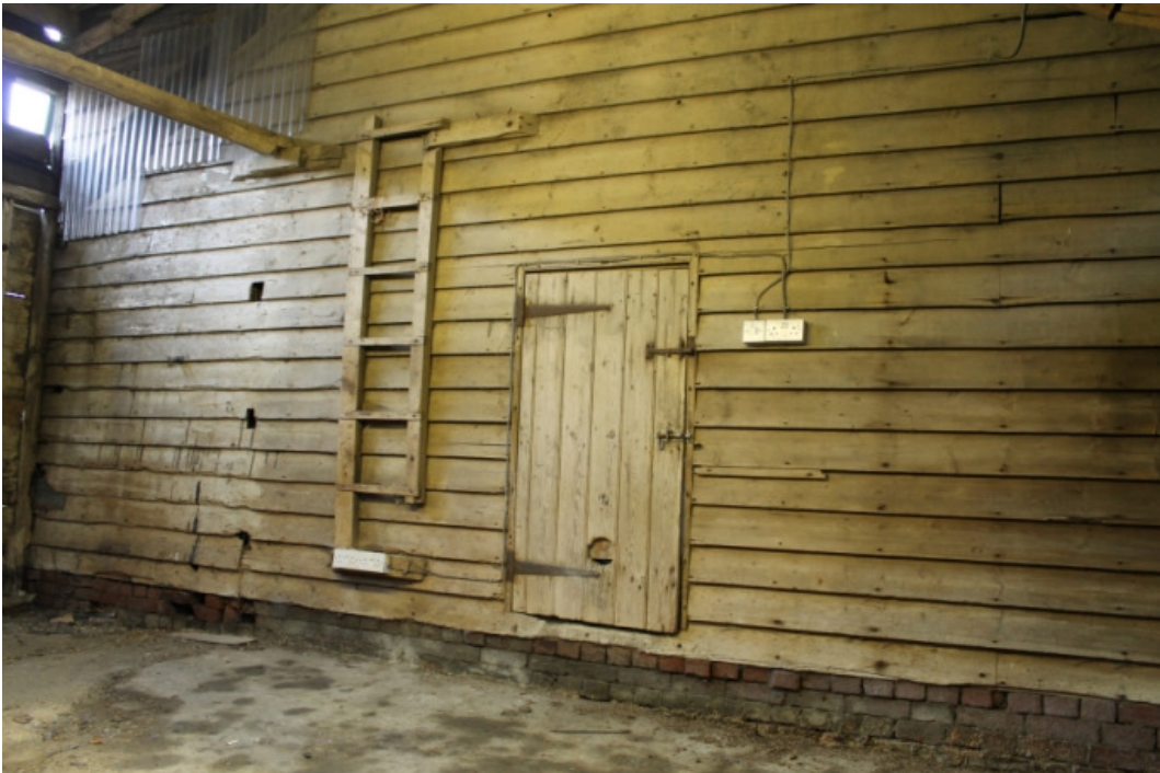
Plate 17 Cow house interior showing fixed ladder to chaff loft with slots for the rails of the calves' pounds to the left of the ladder - view north-west
