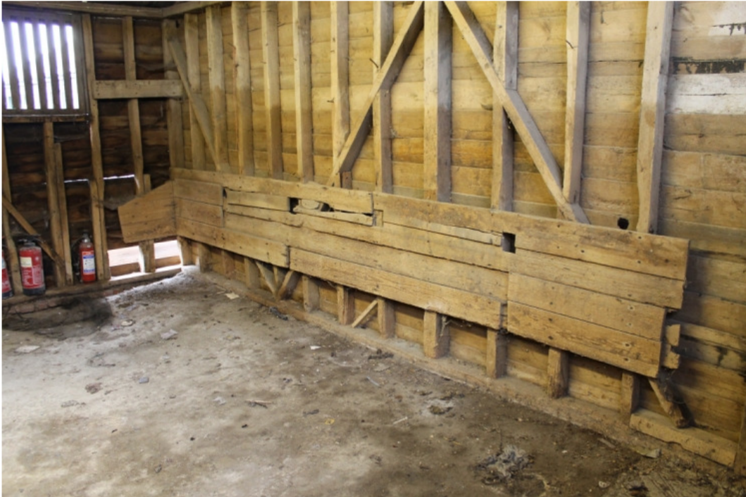
Plate 16 Cow house interior showing remains of manger - view south-west
