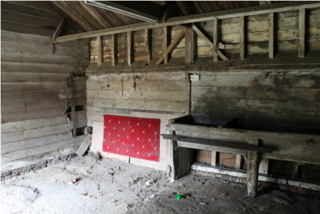
Plate 14 Stable block, two-bayed horse shed showing surviving manger and hay rack – view north
