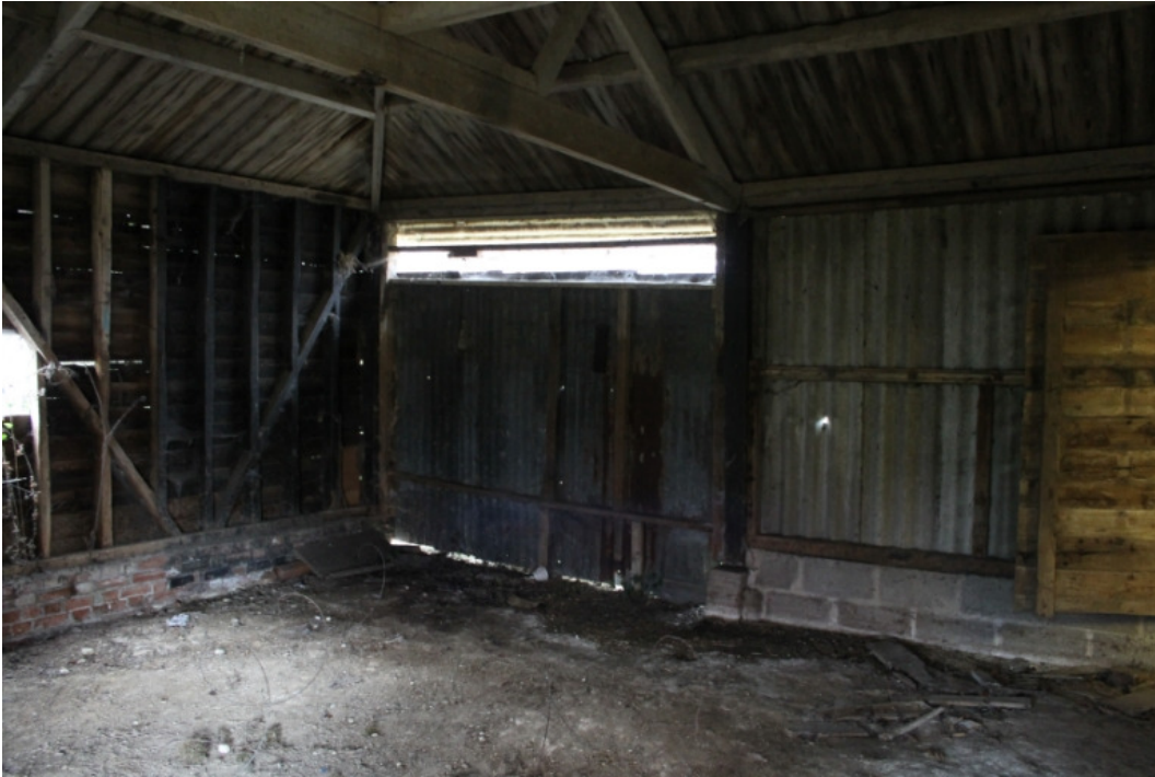
Plate 18 Chaise house interior showing the blocked open front with the central post and concrete buffer - view north-west
