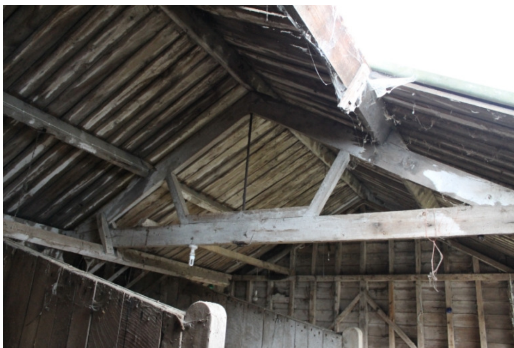
Plate 13 Carthorse stable, truss A - view south-east
