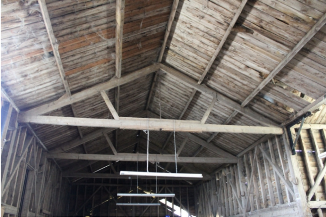
Plate 8 Barn, detail of truss C – view south-west
