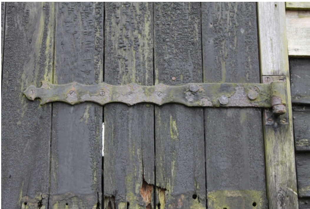
Plate 4 Detail of ornate strap hinge to midstrey door
