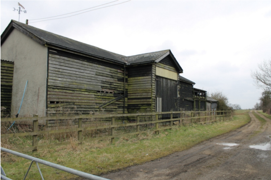
Plate 1 North-west elevation of barn - view south-east
