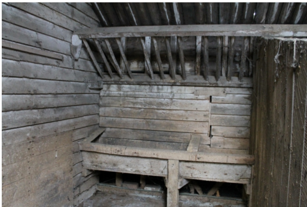
Plate 12 Carthorse stable, stall one showing manger and hay rack – view north-east
