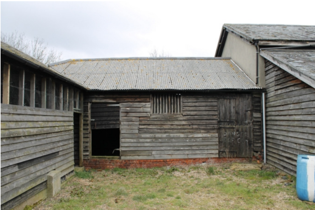
Plate 15 Cow house with hit-and-miss window and traditional stable door - view north-west
