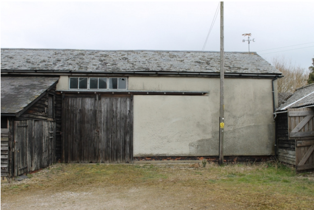
Plate 2 South-east elevation showing inserted Henderson sliding door, with lean-to cattle shed to the left and stable block to the right – view north-west
