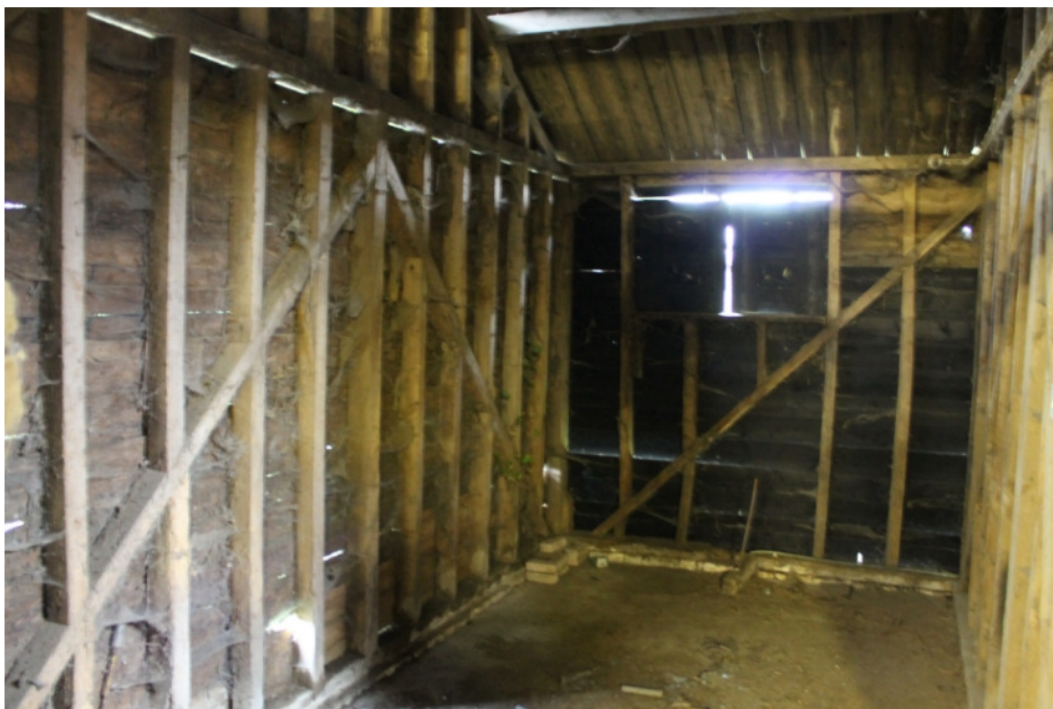
Plate 10 Stable block showing north-west tack room - view north-east
