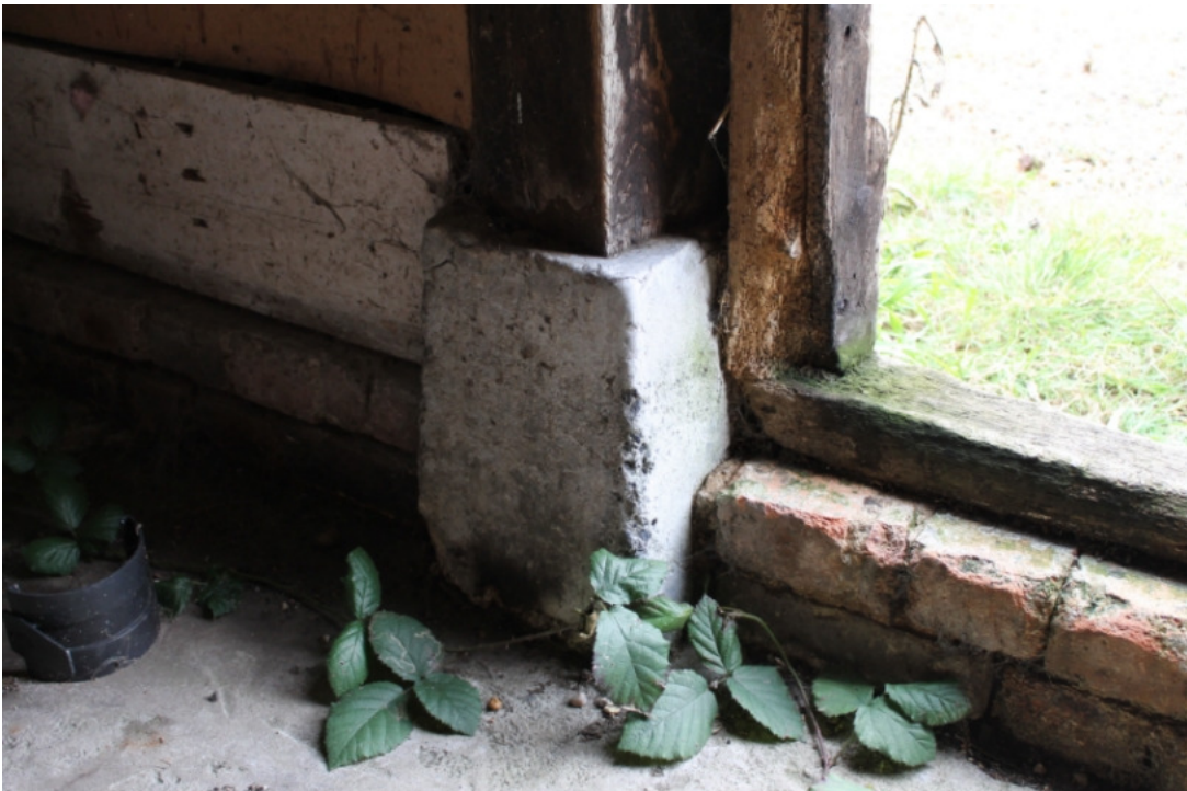
Plate 25 Detail of post with concrete buffer indicating an open front to the lean-to cattle shed
