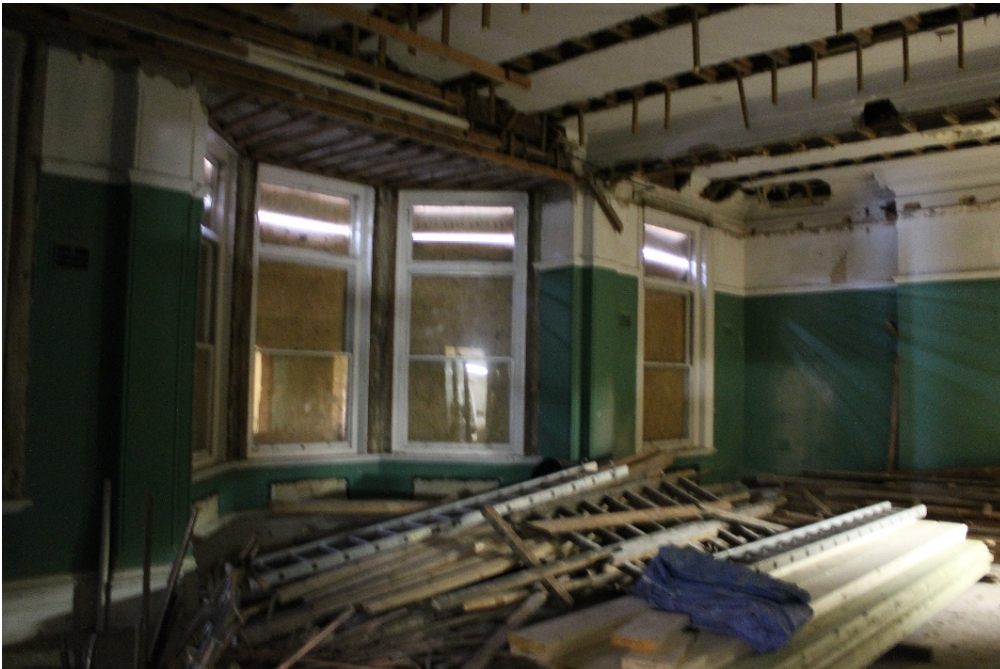
Plate 38 HYD 08 Mess Room, showing artificially lowered ceiling – view north-west
