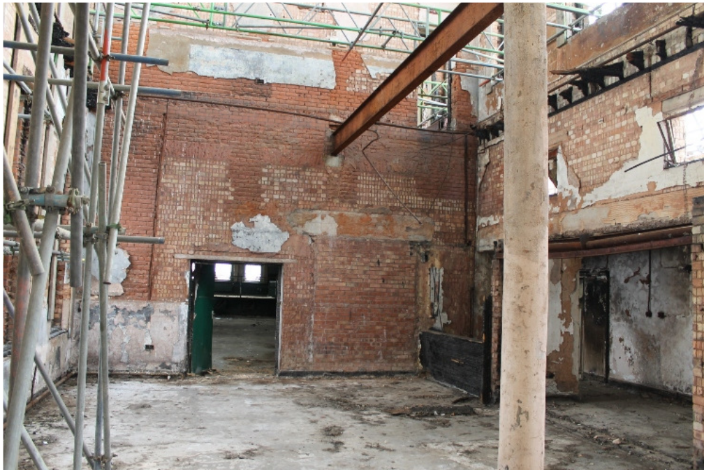
Plate 55 HYD 11 1938 interior, showing blocked windows of the 1904 structure – view east
