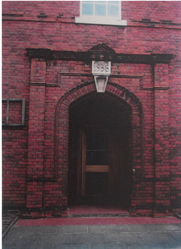
Plate 51 HYD 11 entrance to 1938 structure – view south
