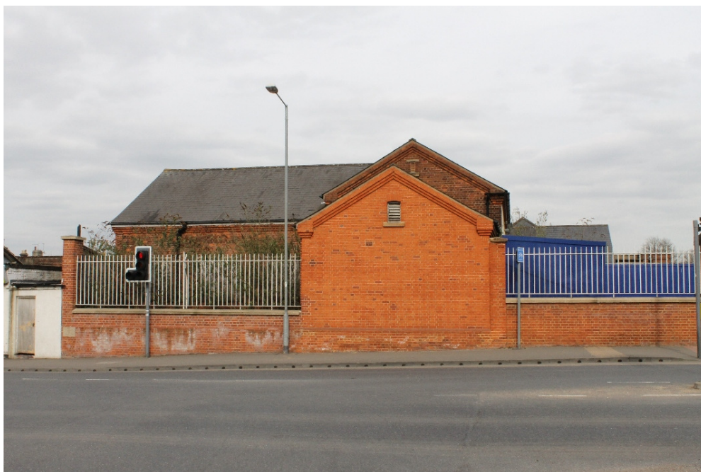
Plate 9 West elevation of MEE 03 built into barracks boundary wall - view east
