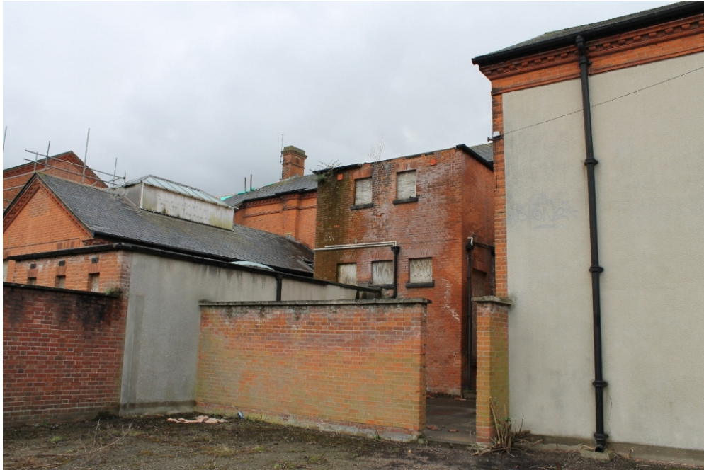
Plate 35 HYD 08 rear of the main range showing projecting service buildings – view south-west
