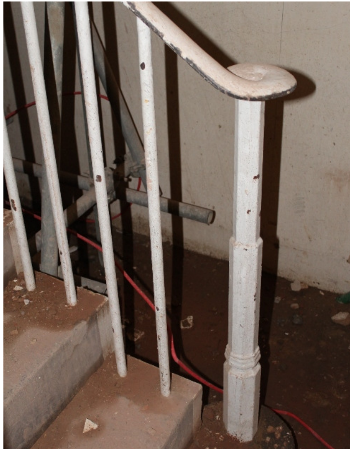
Plate 44 HYD 08 south wing servants' stairs – view north-east
