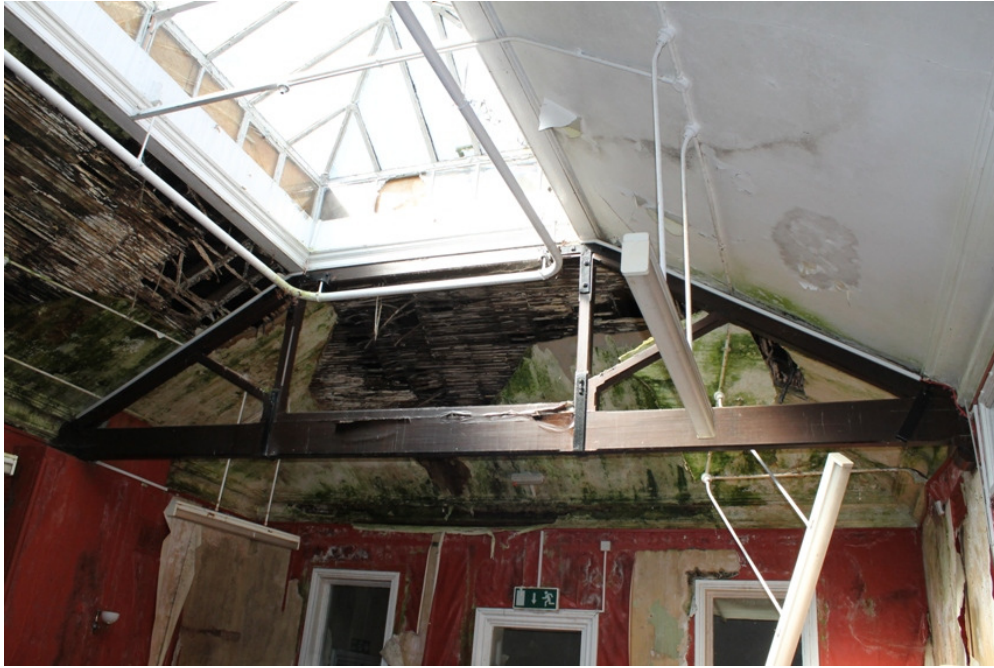
Plate 23 MEE 17 the queen post truss of the Billiard Room, supporting the skylight and the pipe work for the original gas lighting - view south-east
