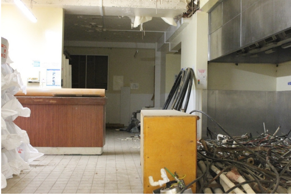
Plate 39 HYD 08 kitchen converted from the First Officer's rooms – view north
