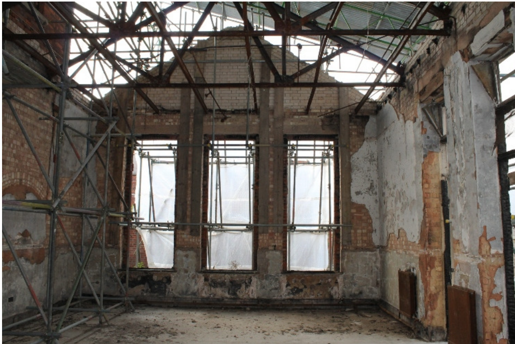
Plate 56 HYD 11 interior of the 1938 Corporals' Restaurant – view south
