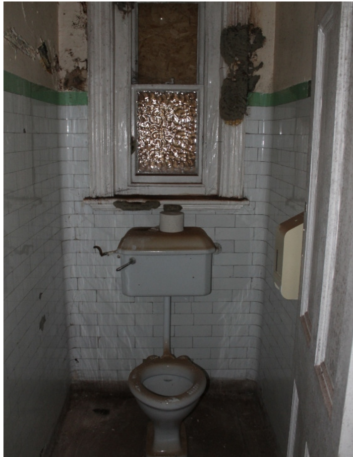
Plate 40 HYD 08 lavatory block, with 1961 'New Lindone' toilet – view east
