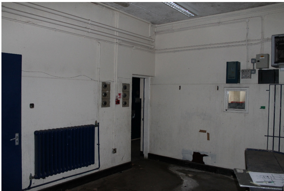
Plate 4 Day reception of MEE 01, showing the gun safes and the viewing window into the holding cell – view north-west
