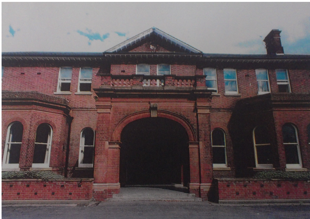
Plate 13 Main entrance to MEE 17, showing the Italianate windows of the ground floor – view east (Ingram, 2000)
