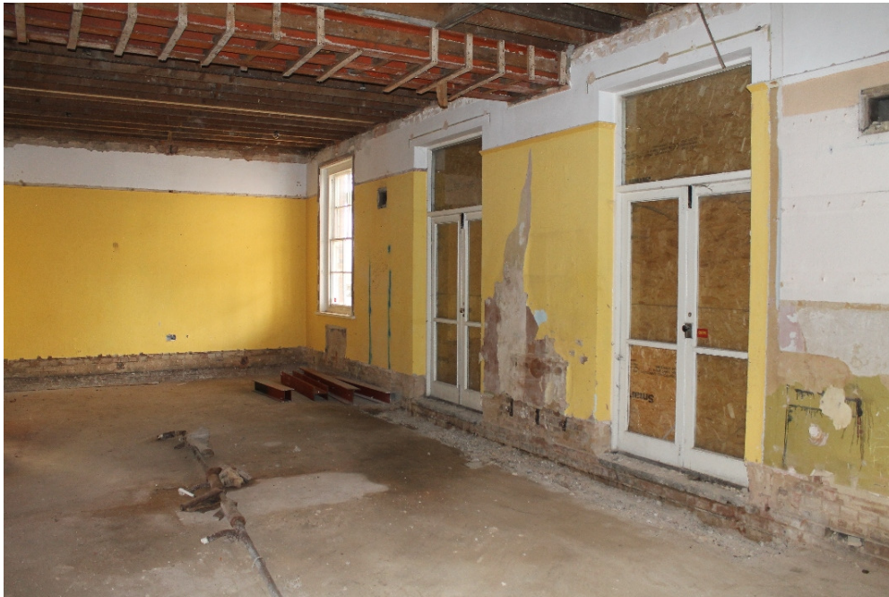
Plate 43 HYD 08 bedrooms converted to bar, with windows altered to French doors – view north
