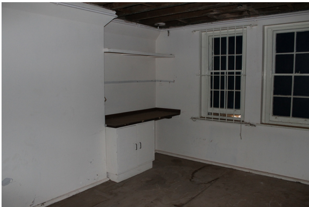
Plate 26 MEE 17 ground floor servants' room with ?original unit – view north-west
