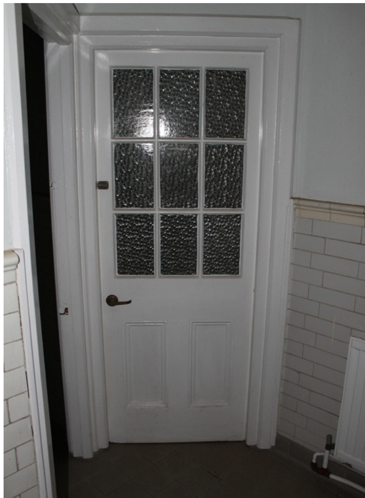
Plate 30 MEE 17 first floor, original door to bathroom
