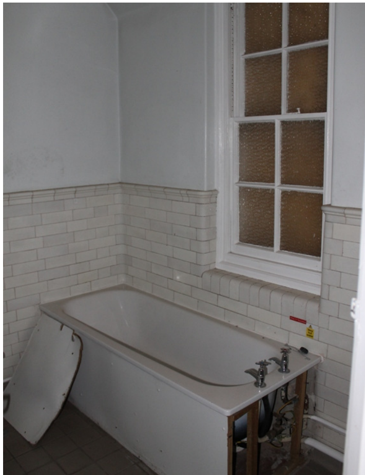
Plate 31 MEE 17 first floor bathroom, original tiling and hammered window glass
