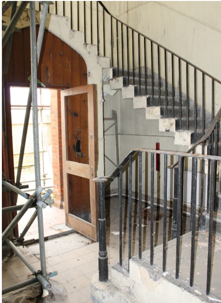
Plate 52 HYD 11 1904 entrance and staircase – view north-east
