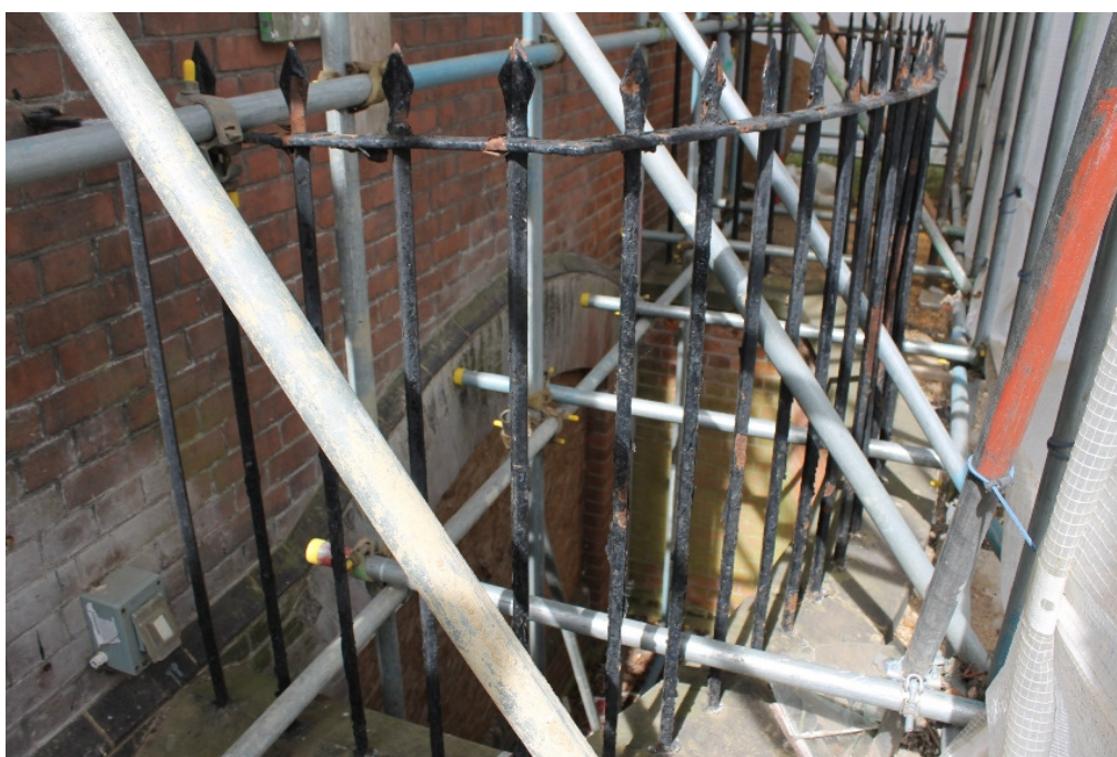
Plate 50 HYD 11 light well for basement on east elevation – view north-west
