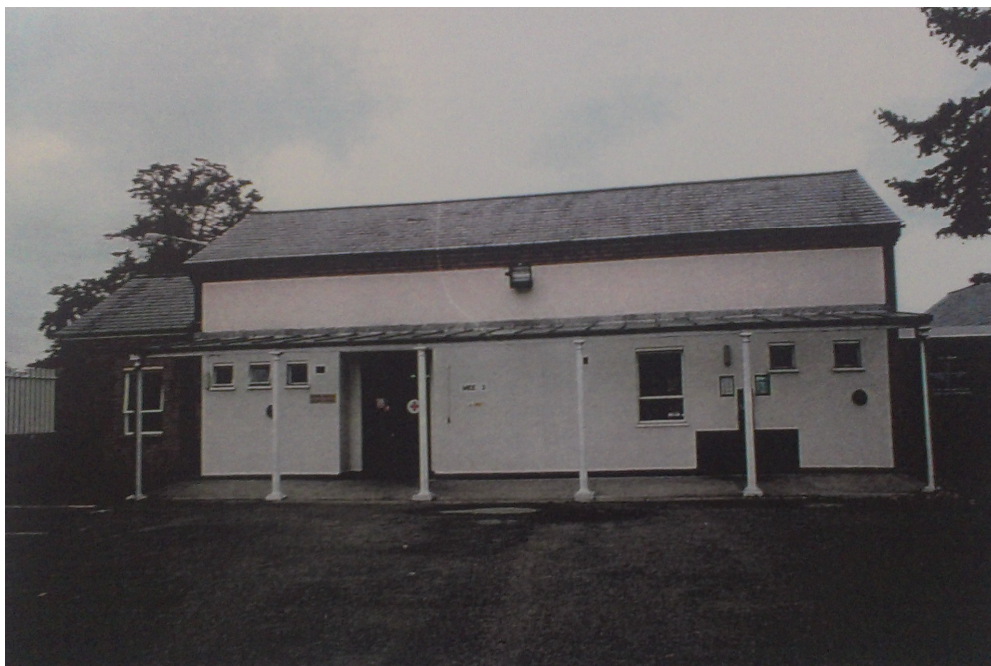
Plate 8 MEE 03 original Guard House converted to Medical Centre – view north (Ingram, 2000)
