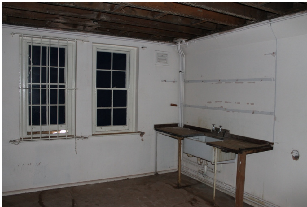
Plate 25 MEE 17 ground floor servants' room with ?original Belfast sink – view north-east
