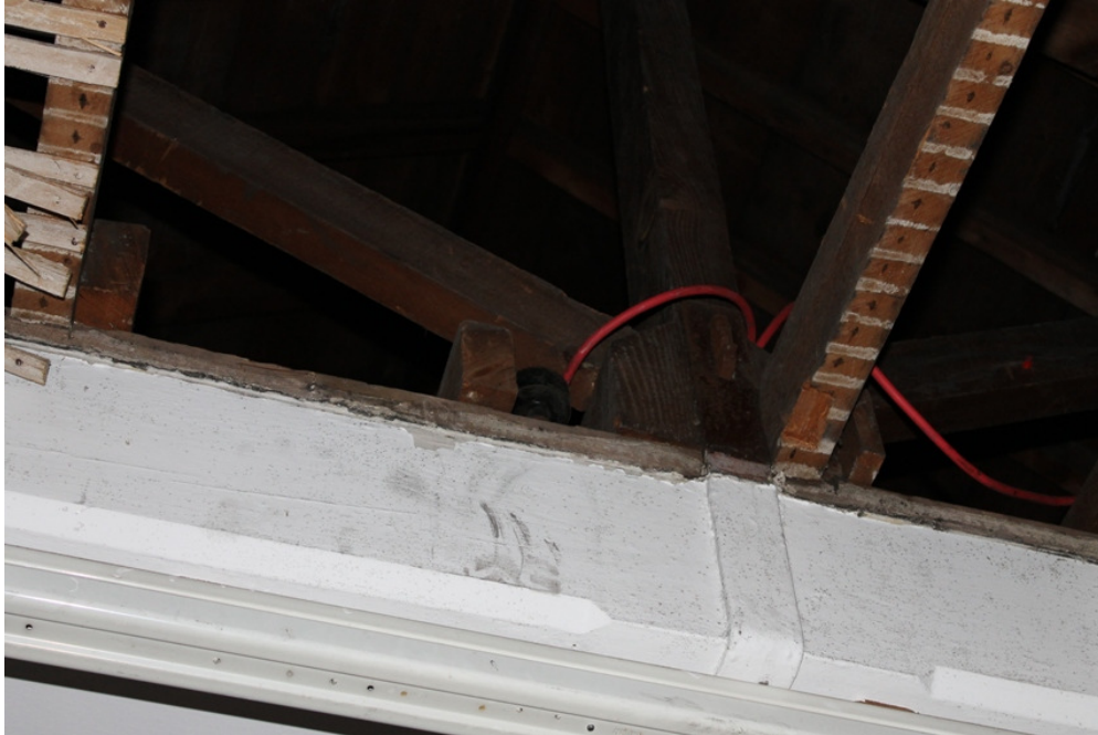
Plate 29 Exposed king post roof truss in MEE 17
