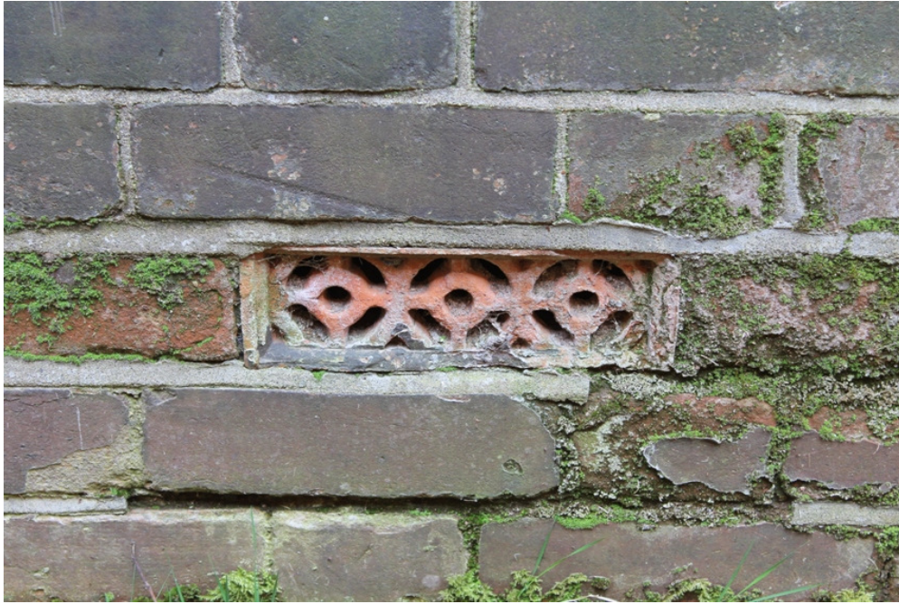
Plate 17 Detail of air brick in south wall - view north
