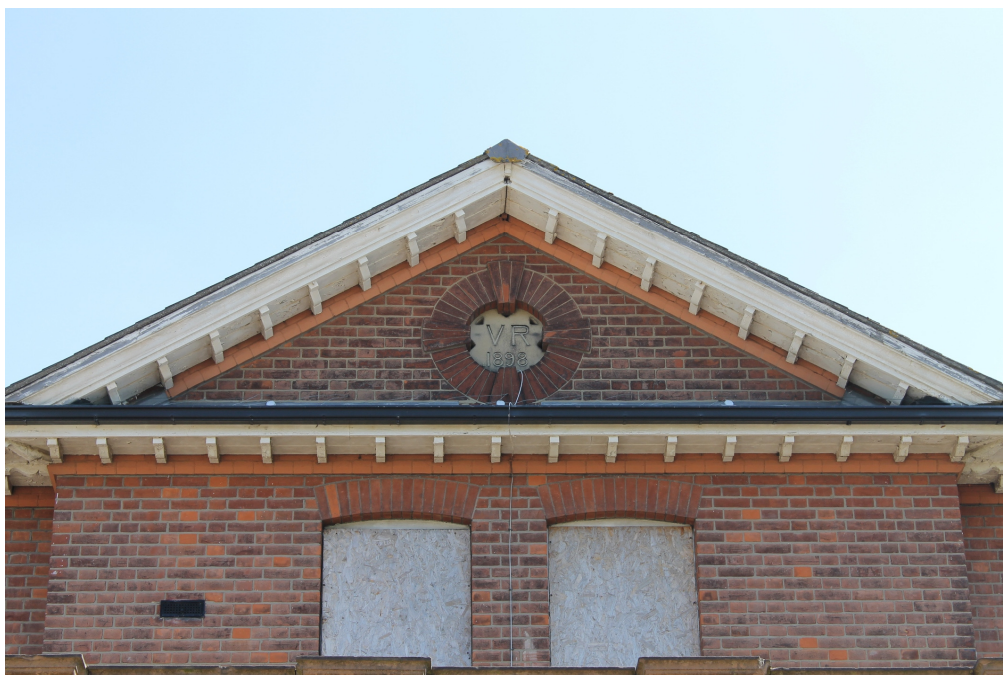
Plate 14 MEE 17, inscription in pediment above main entrance - view east
