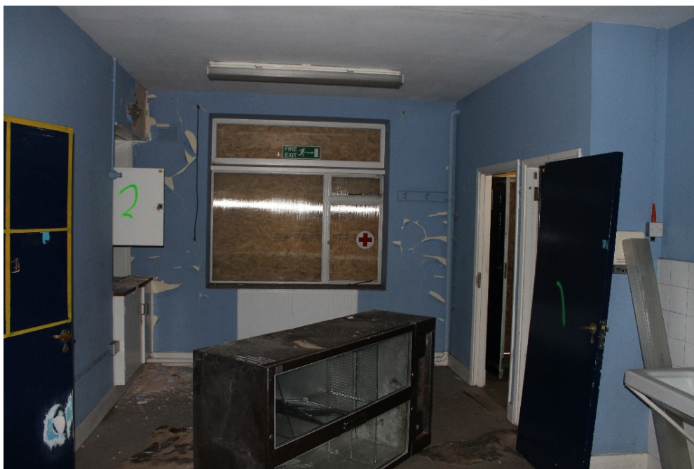
Plate 11 MEE 03 Medical Centre interior, showing replacement metal-framed window – view north
