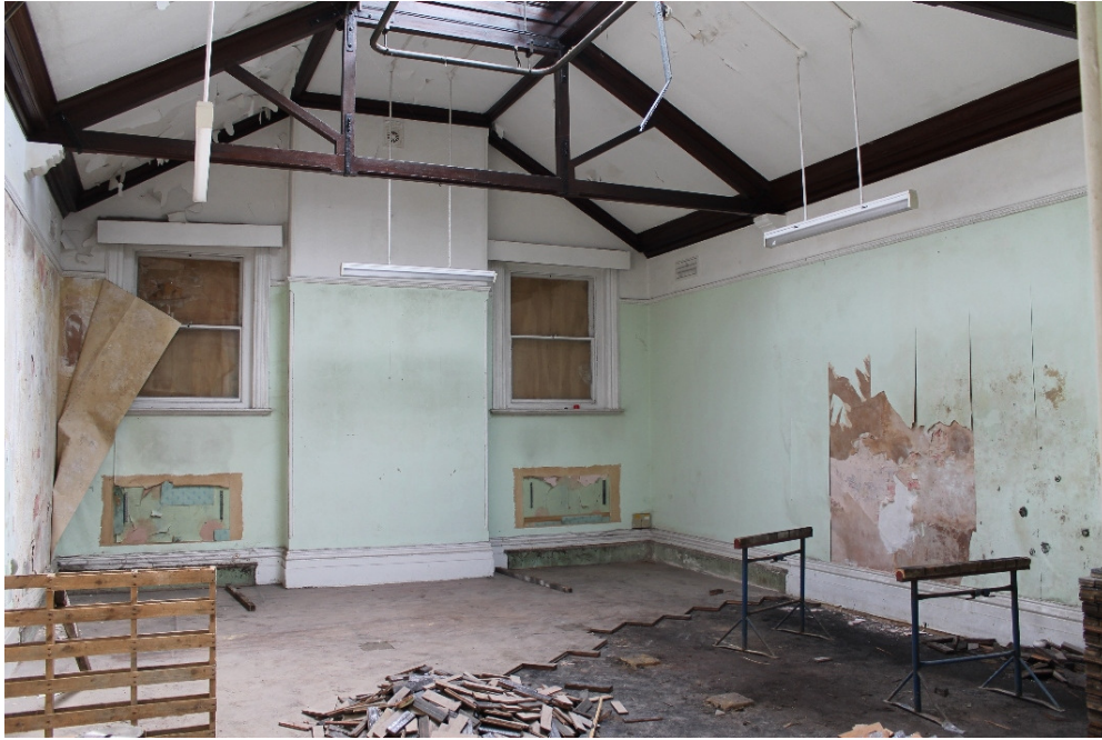
Plate 41 HYD 08 Billiard Room with parquet floor and queen post trusses – view east
