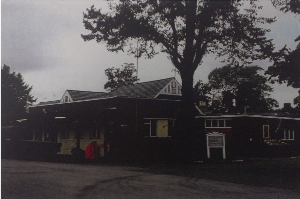
Plate 1 MEE 01, the modern Guard House with the original Brigade Offices visible in the background - view north-west (Ingram, 2000)
