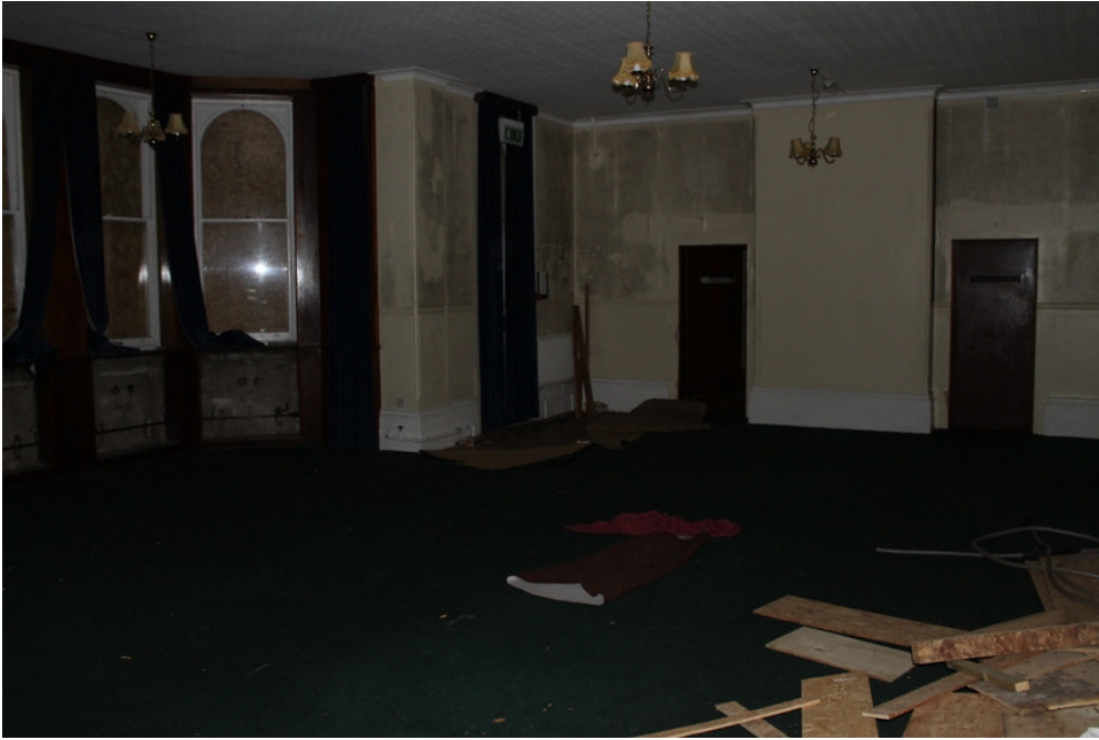
Plate 21 MEE 17 Mess room, showing the inserted doors to the kitchen in the north wall – view north-west
