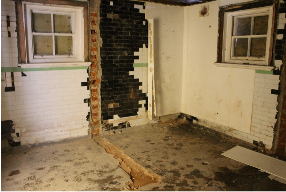
Plate 45 HYD 08 interior of the first floor Officers' bathroom - view north-east
