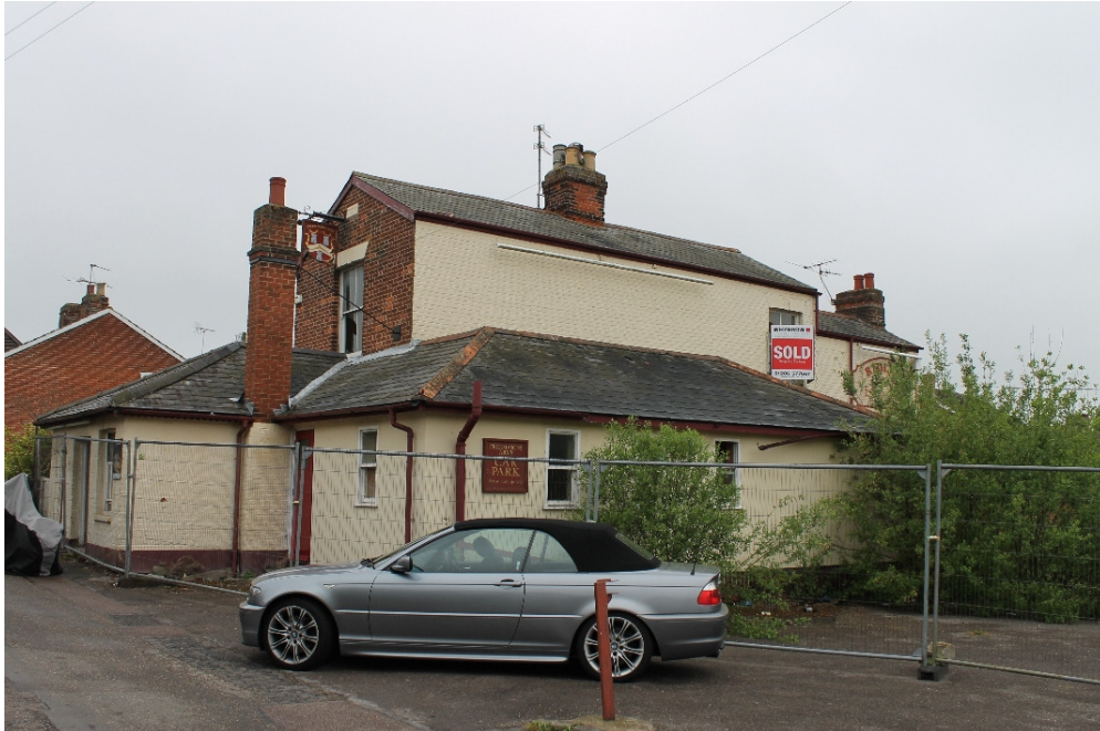
Plate 1 The Freemasons Arms with the original Wright Villa in the background and the phase 2 and phase 3 extensions in the foreground - view north-west
