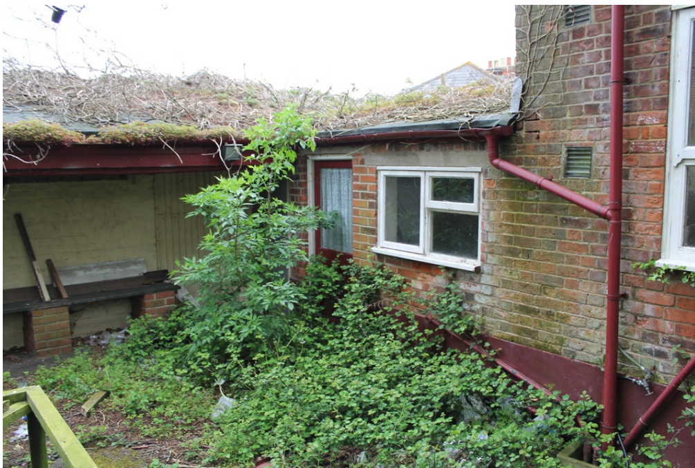
Plate 17 Phase 3 extension to service wing - view north
