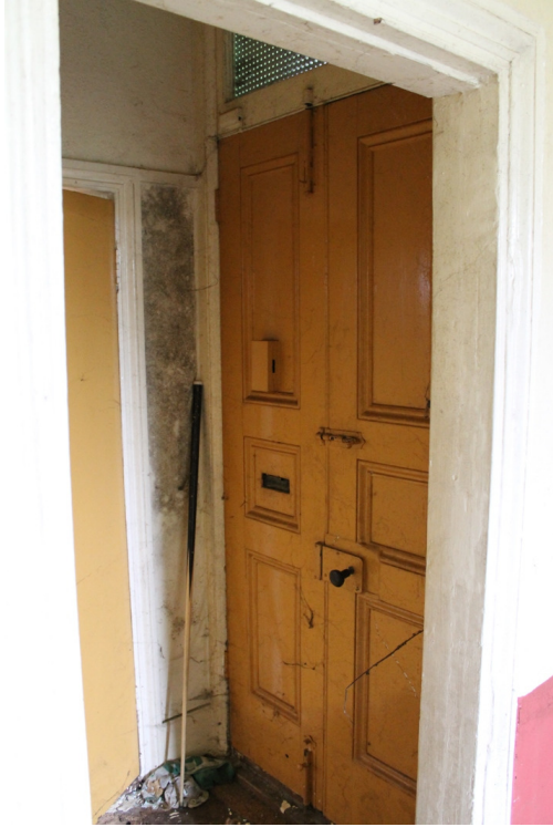
Plate 9 Detail of original front door
