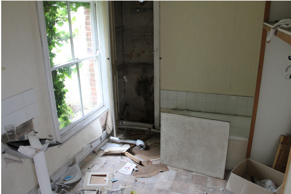
Plate 14 Bathroom, with blocked fireplace behind bath – view north-west
