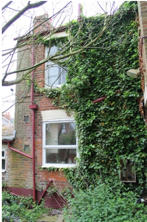
Plate 4 West elevation of service wing – view north-east
