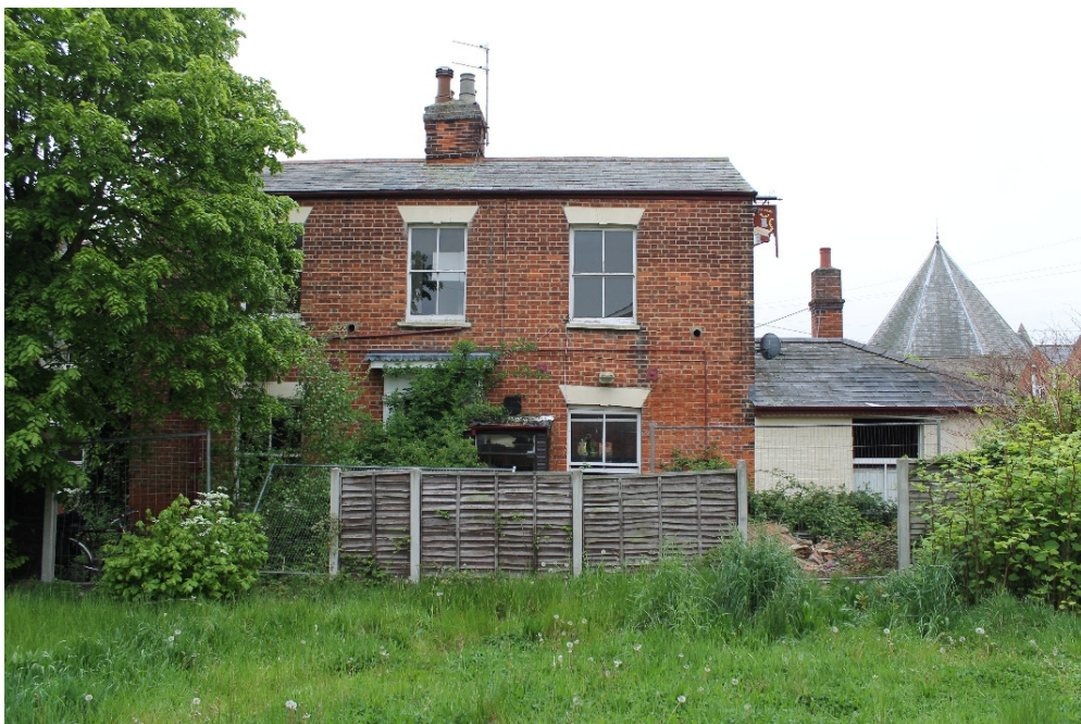
Plate 2 West elevation of Wright Villa - view east
