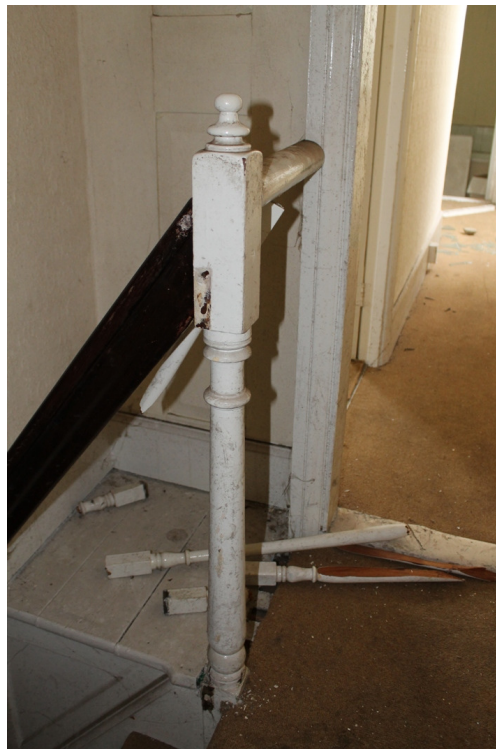
Plate 11 Detail of wood panelling to landing and turned newel post
