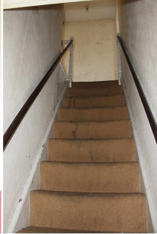
Plate 10 Staircase with original banisters and turned newel posts
