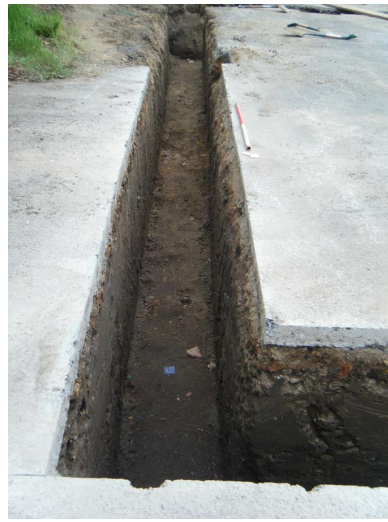
Plate 4 Archive store footings, pit F2. Facing south-west.
