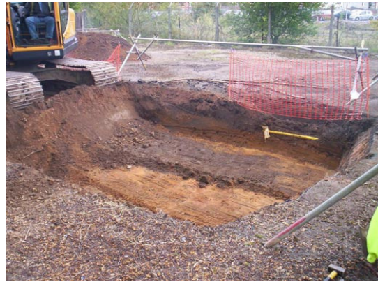
Plate 2 Bat hibernaculum foundations, showing modern service. Facing west.
