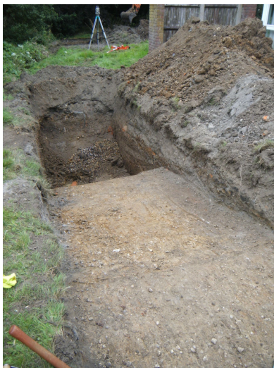
Plate 1: T1, facing north.
