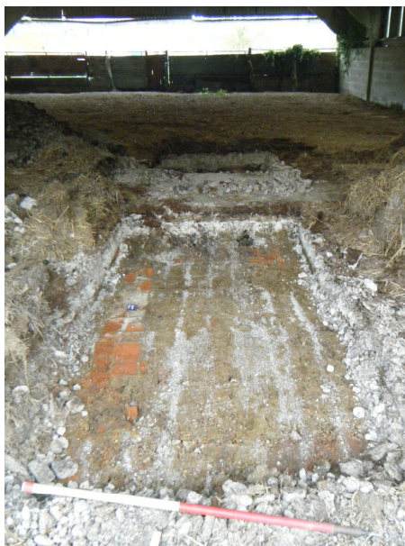
Plate 3: T6, facing south-west. (F8 is visible to the left.)
