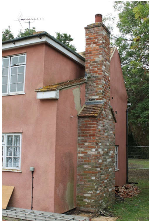
Plate 14 Phase 2 single-storey extension with the Phase 3 second storey extension above – view south-west
