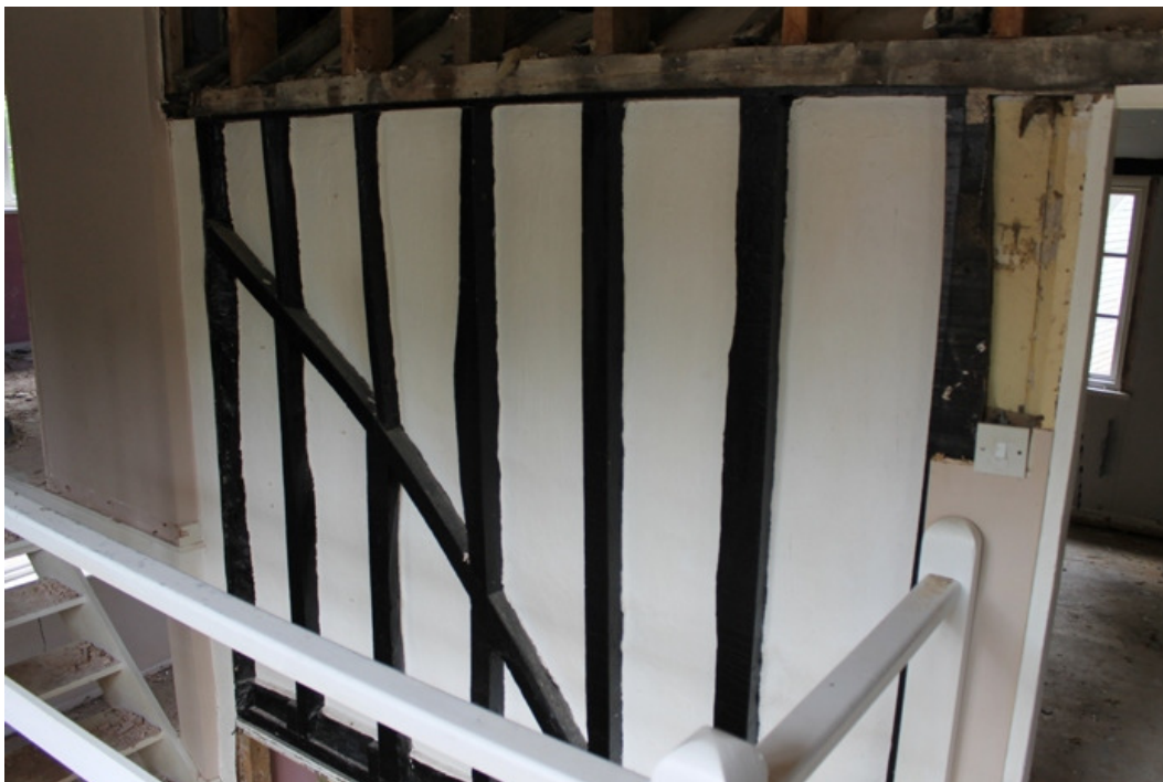
Plate 6 Surviving timbers of the first floor frame - view south-west
