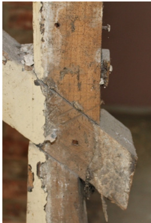
Plate 5 Carpenter's mark (II) on brace and stud – view west
