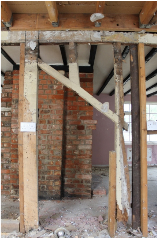
Plate 4 Surviving timbers of the east wall - view west
