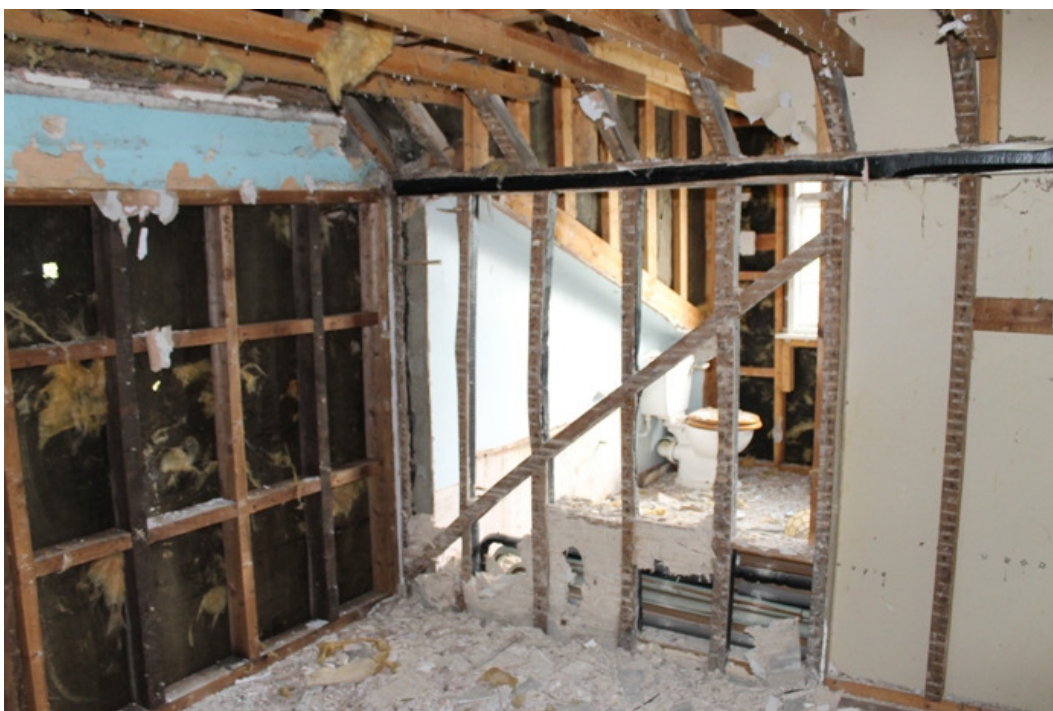
Plate 7 Surviving timbers of the first floor frame, with modern replacements to the left - view north-east
