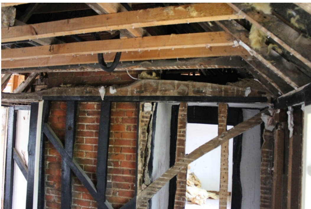
Plate 11 The relocated tie beam in bedroom 4 - view south
