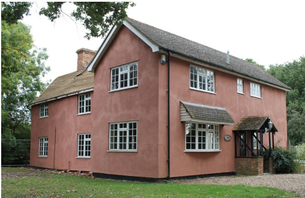
Plate 15 Phase 3 extension with the original structure to the rear – view north-east
