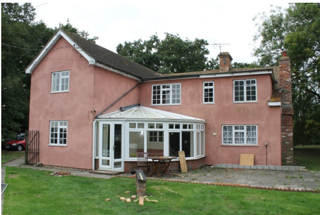
Plate 16 The Phase 3 extensions to the left of and above the Phase 2 extension, with the original structure in the background – view west
