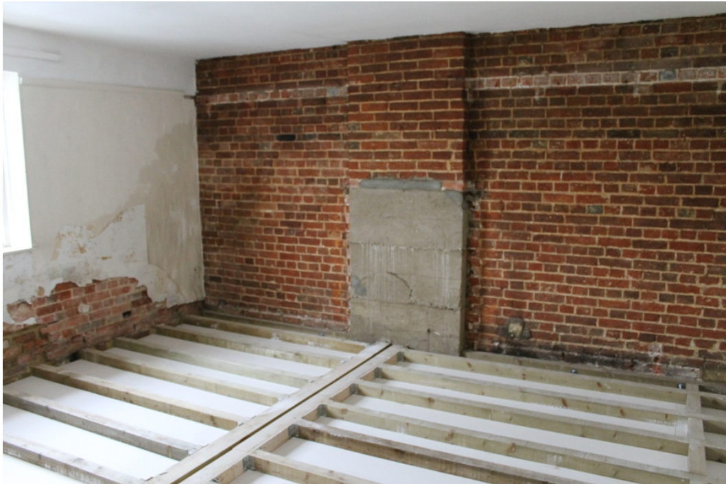
Plate 18 Bedroom 1, showing the blocked fireplace in the Phase 2 brickwork – view south-west
