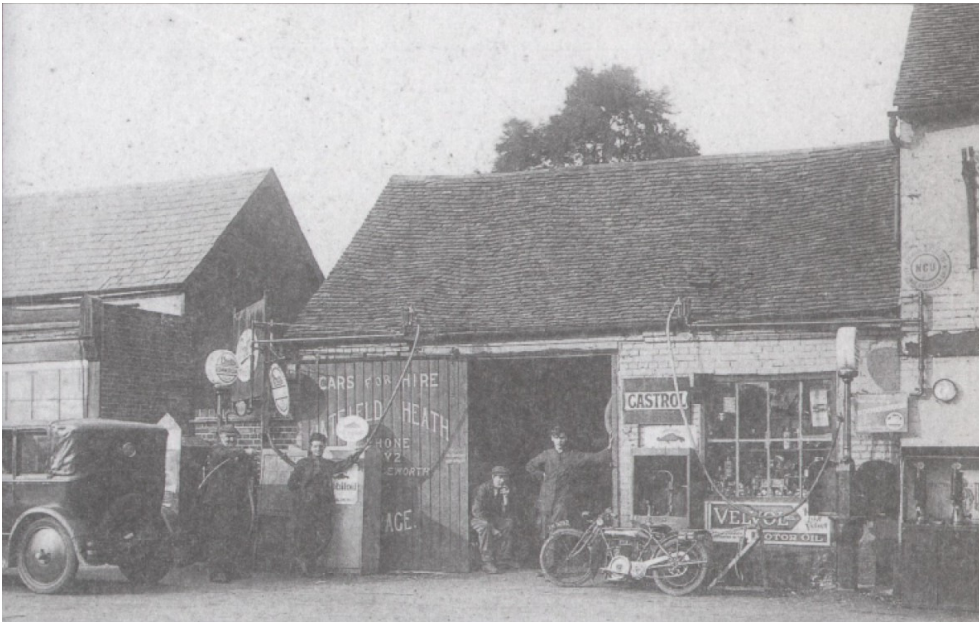
Illustration 3 Halls' garage converted from Aaron Hawkins' Coal Depot (A History of Hatfield Heath)
