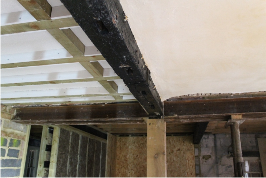
Plate 5 Girding beam at the rear of the Phase 1 structure, with exposed mortices in underside of beam and single peg holes - view west
