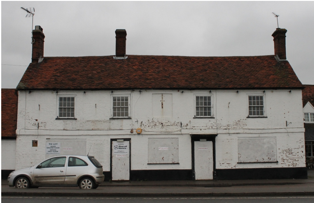
Plate 1 South elevation of the Stag Inn - view north
