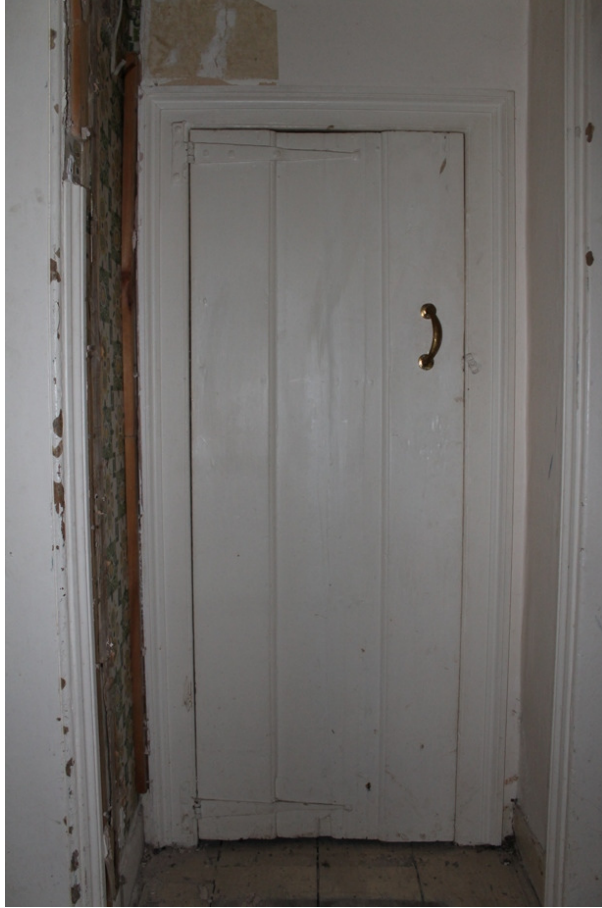
Plate 21 Cupboard at head of Phase 3 staircase with original plank door – view west
