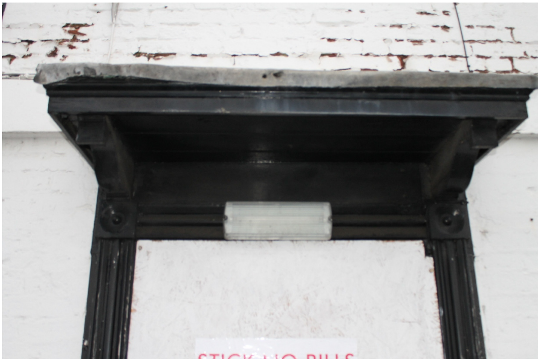
Plate 2 Detail of original Georgian hood and fluted door surround with bull's eye corner decoration – view north
