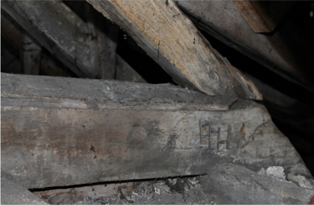
Plate 23 Chiselled carpenter's mark on the end of an attic tie beam – view north-west.
