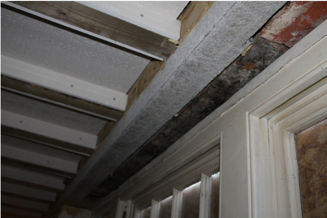
Plate 12 Phase 2 timber window lintel above 20th-century window in dining area - view south-east
