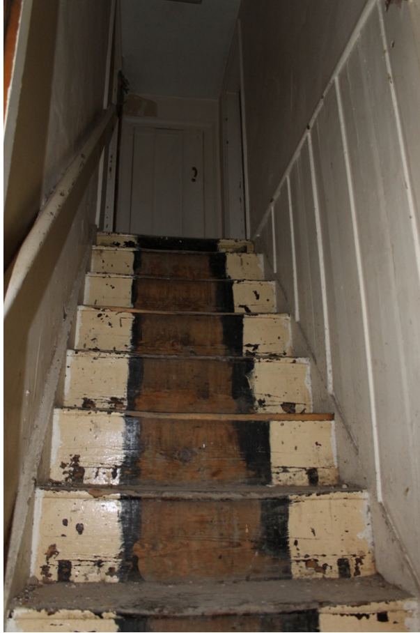
Plate 15 Phase 3 staircase to first floor - view west
