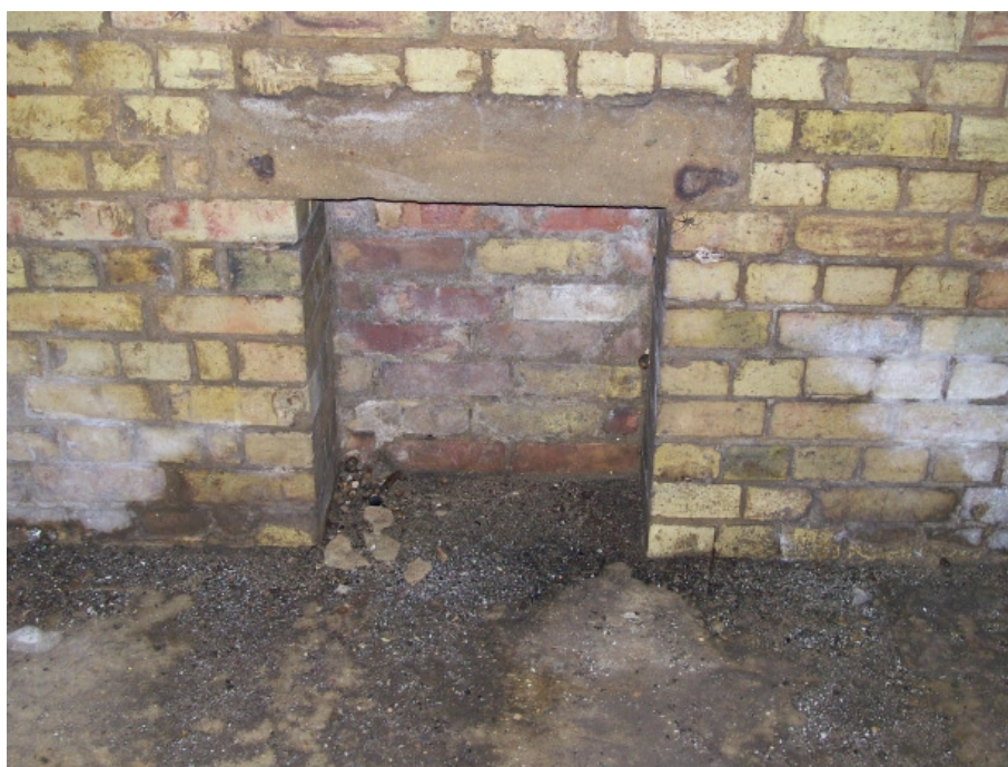
Plate 6 Emergency escape hatch in west wall - view south-west.
