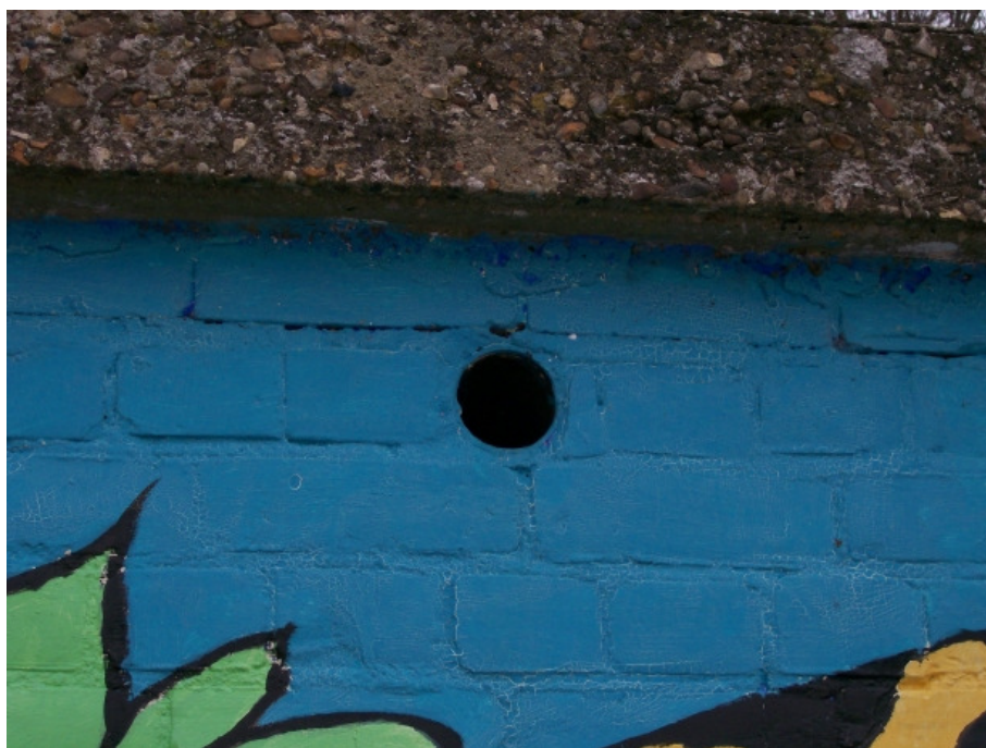
Plate 5 Detail of ventilation hole.
