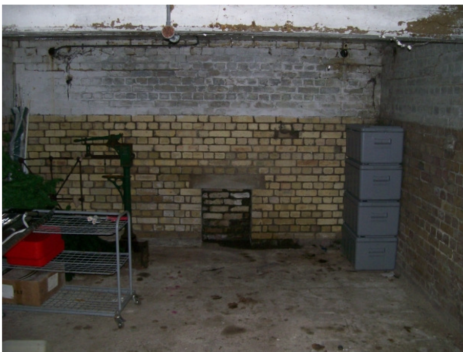
Plate 3 East shelter interior - view north-east.
