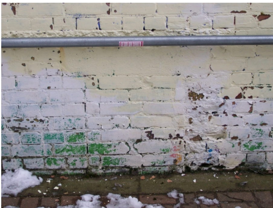
Plate 7 Exterior of the air-raid shelter showing the emergency escape hatch in the west wall - view north-east.
