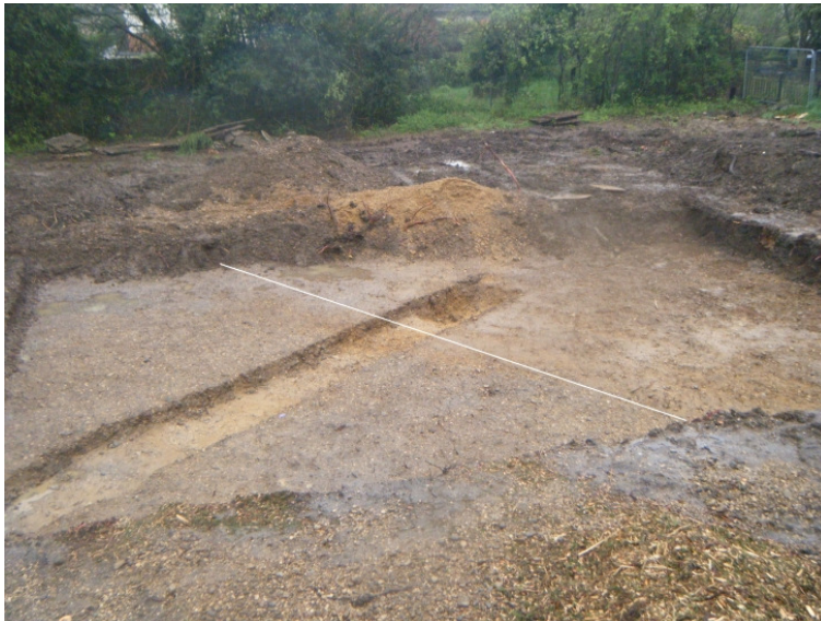
Plate 1 F10 metalled track - view north-west
