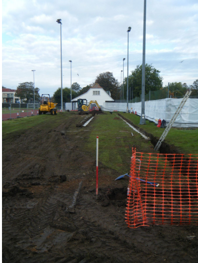
Plate 1 Site shot showing footings trenches.
