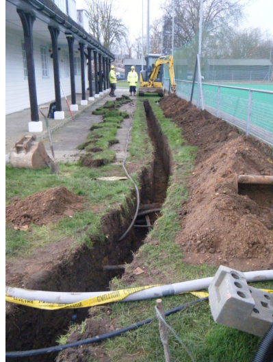
Plate 2 The trench for the new services.
