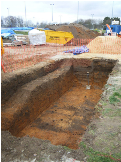
Plate 3 The pit for a new soakaway
