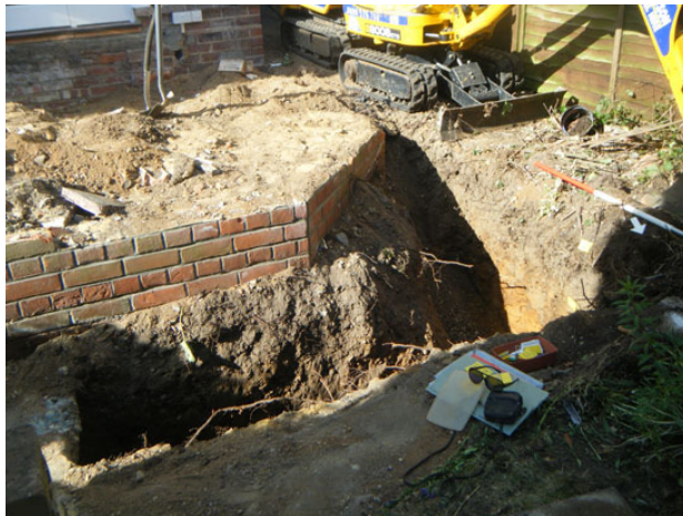
Photograph 1 Foundation trench, looking S
