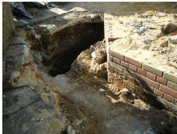
Photograph 2 Foundation trench, looking SE
