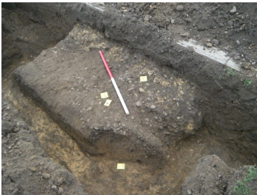
Photograph 1 Wall foundation F1 and gravel surface L4
