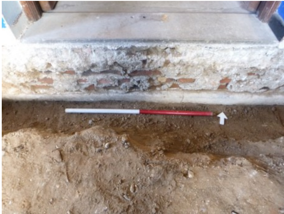
Photograph 3 20th-century doorway, course of bricks and early threshold stone
