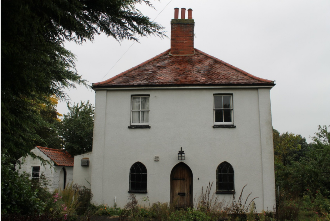
Plate 1 South-east elevation - view north-west.
