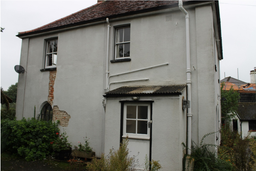
Plate 5 South-west elevation with 20th-century porch - view north-east.
