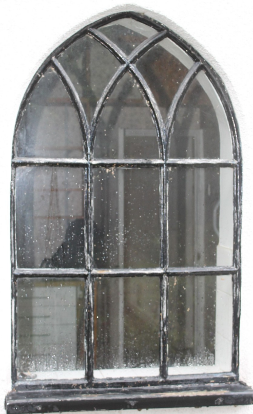
Plate 2 Detail of original timber-framed Gothic Revival window to south-east elevation - view north-west.
