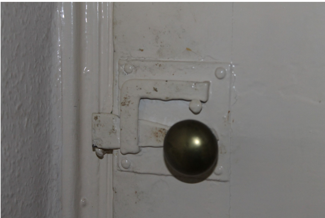
Plate 8 Detail of original? latch to cupboard in sitting room 2.
