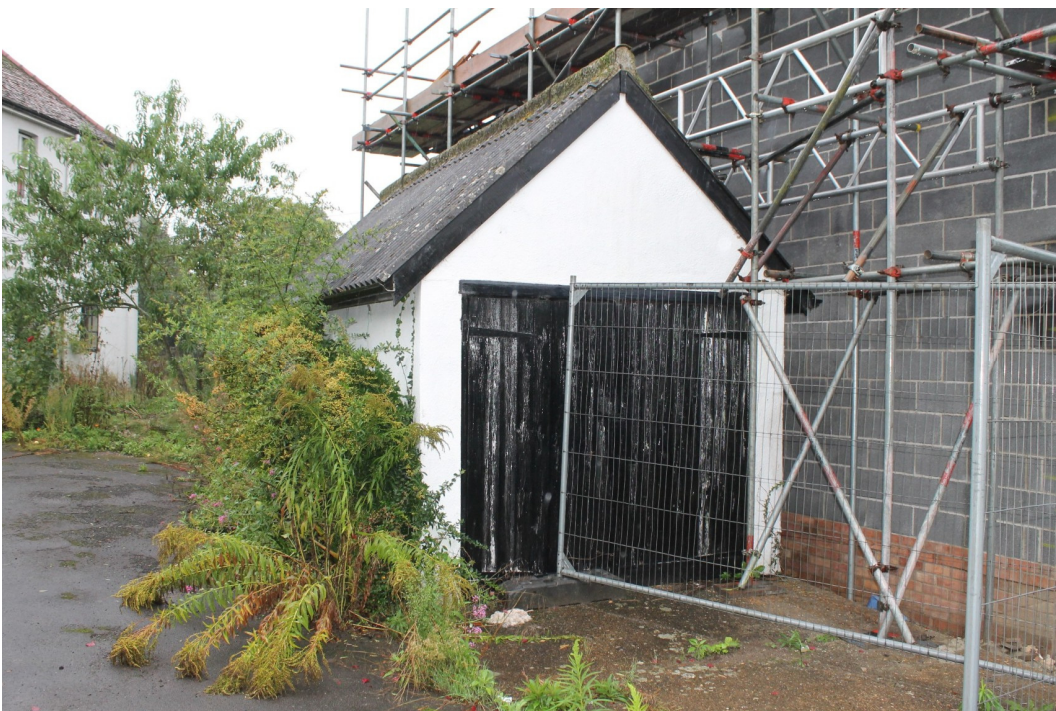
Plate 16 20th-century garage - view west.
