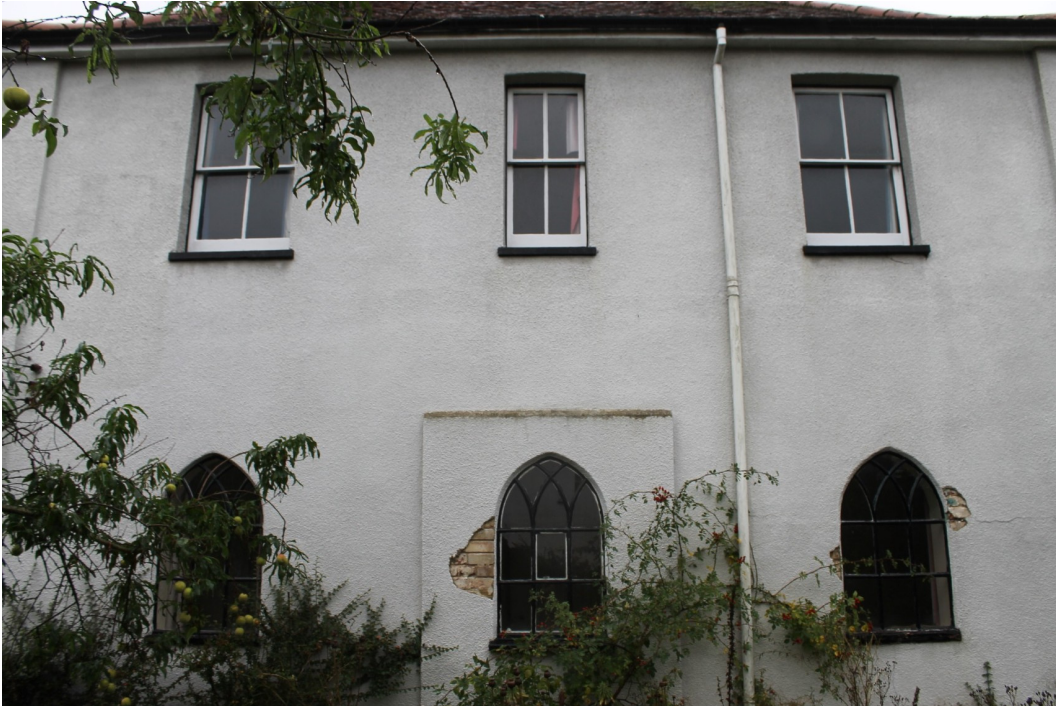
Plate 3 North-east elevation showing the replacement metal-framed Gothic window inserted into the original entrance way - view south-west.
