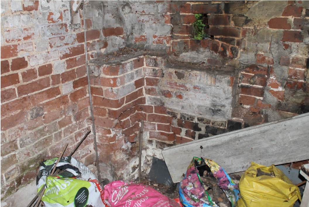
Plate 15 Interior of the wash house showing the former position of the copper and the blocked stoking arch - view north-west.
