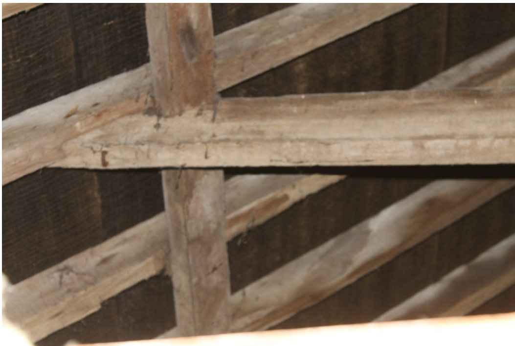
Plate 13 Detail of trrenched collar and through purlin in roof.
