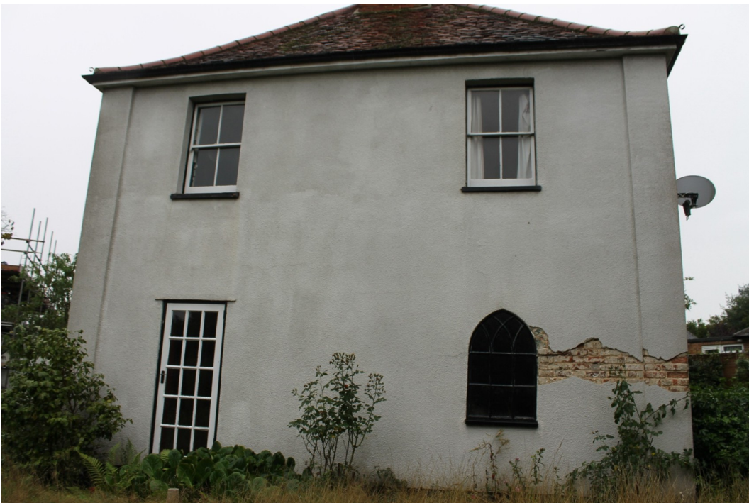
Plate 4 North-west elevation showing the 20th-century doorway inserted through an original Gothic Revival window opening - view south-east.
