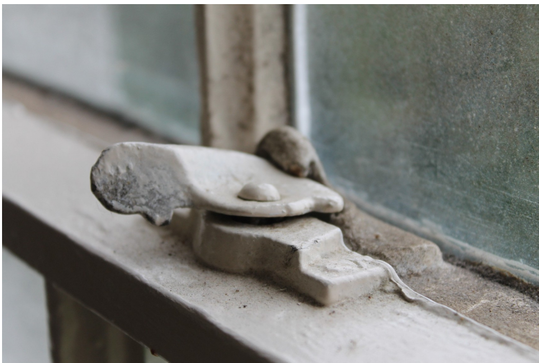
Plate 11 Detail of original catch to window in bedroom 1.
