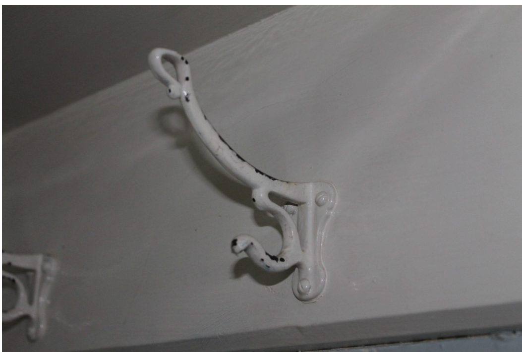
Plate 12 Detail of original? coat hook in bedroom 2.
