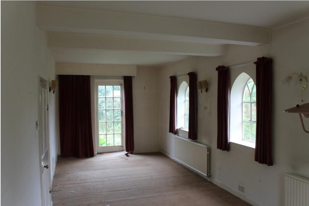
Plate 7 Sitting room 1 viewed from the dining room, showing the original entrance hallway indicated by the beams and the original entrance converted to a window on the right, and the doorway in the far wall inserted through an original window opening - view north
