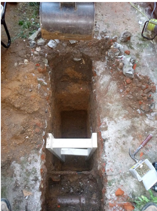
Photograph 2 Foundation trench, looking NE
