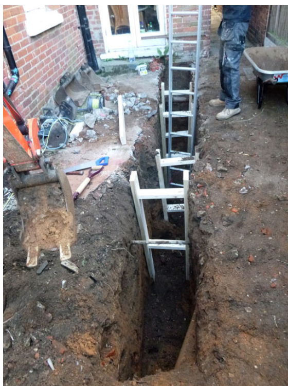
Photograph 3 Foundation trench, looking SW
