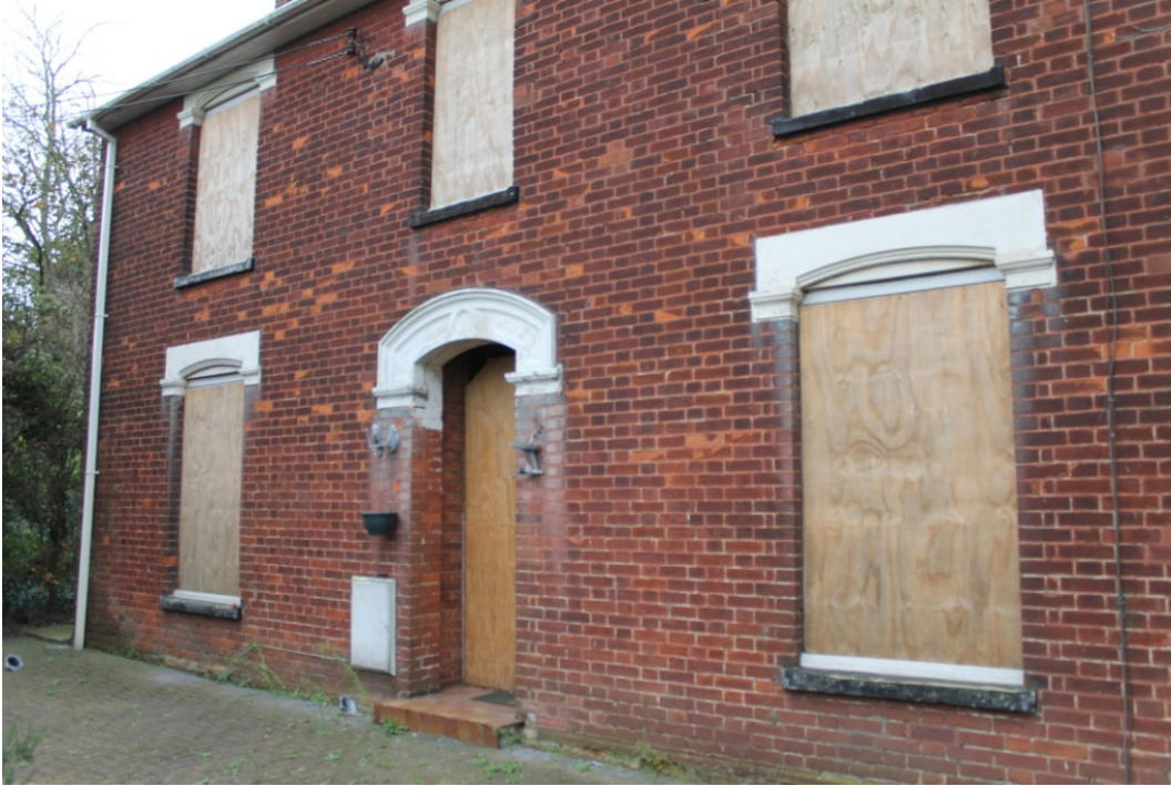
Photograph 3 North-west elevation of 'The Warrens' - view north-east.
