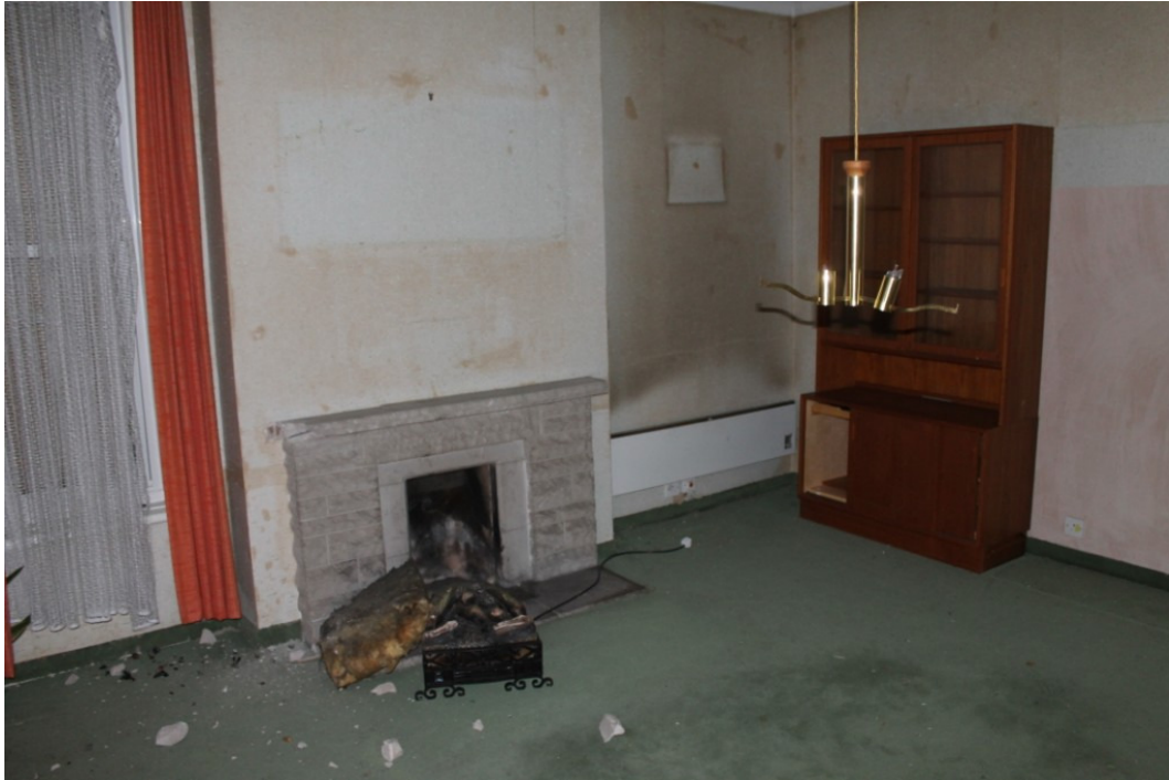
Photograph 8 Interior of GF1 showing the replacement fire surround - view east.
