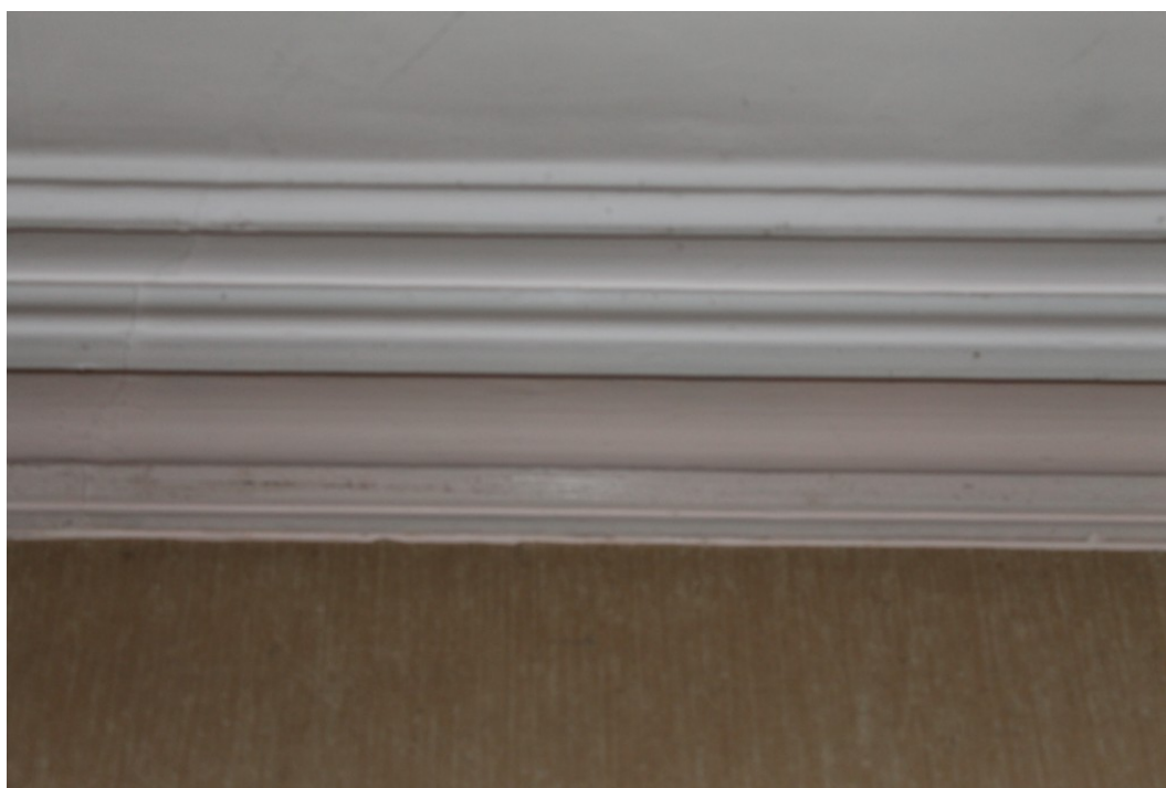
Photograph 13 Detail of original coving in GF2.
