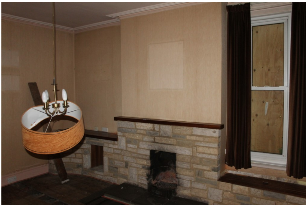
Photograph 9 Interior of GF2 showing the replacement fire surround – view south.
