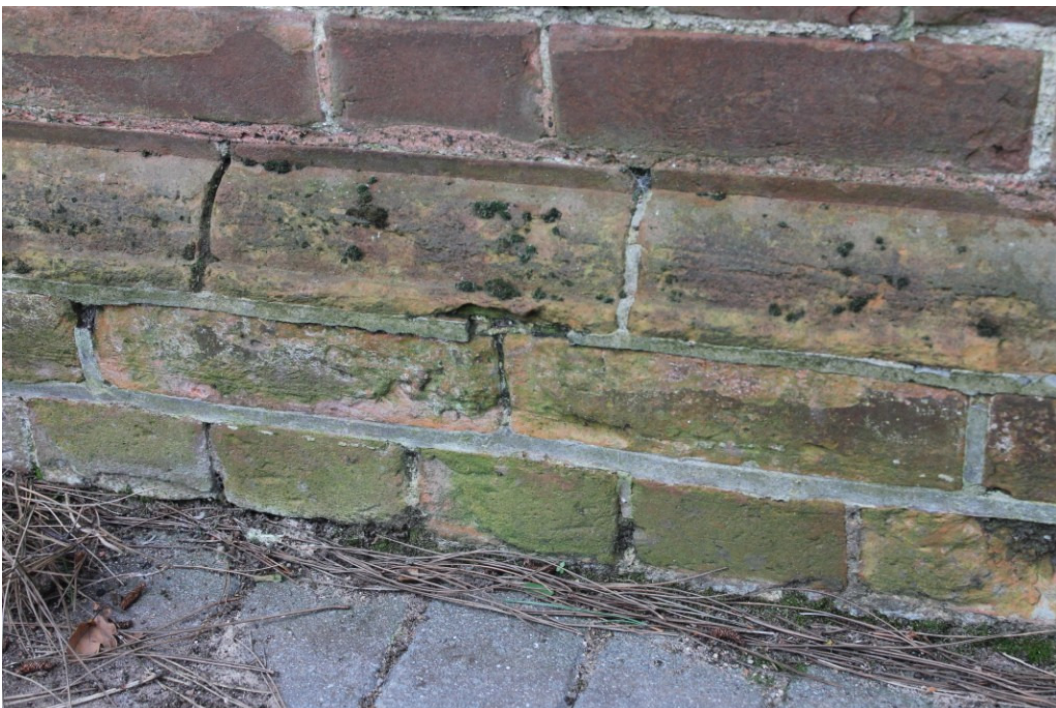
Photograph 2 Detail of the moulded brick plinth to 'The Warrens'.
