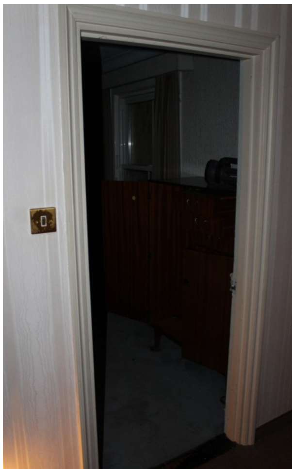
Photograph 12 Original architrave around doorway to FF1 – view east.
