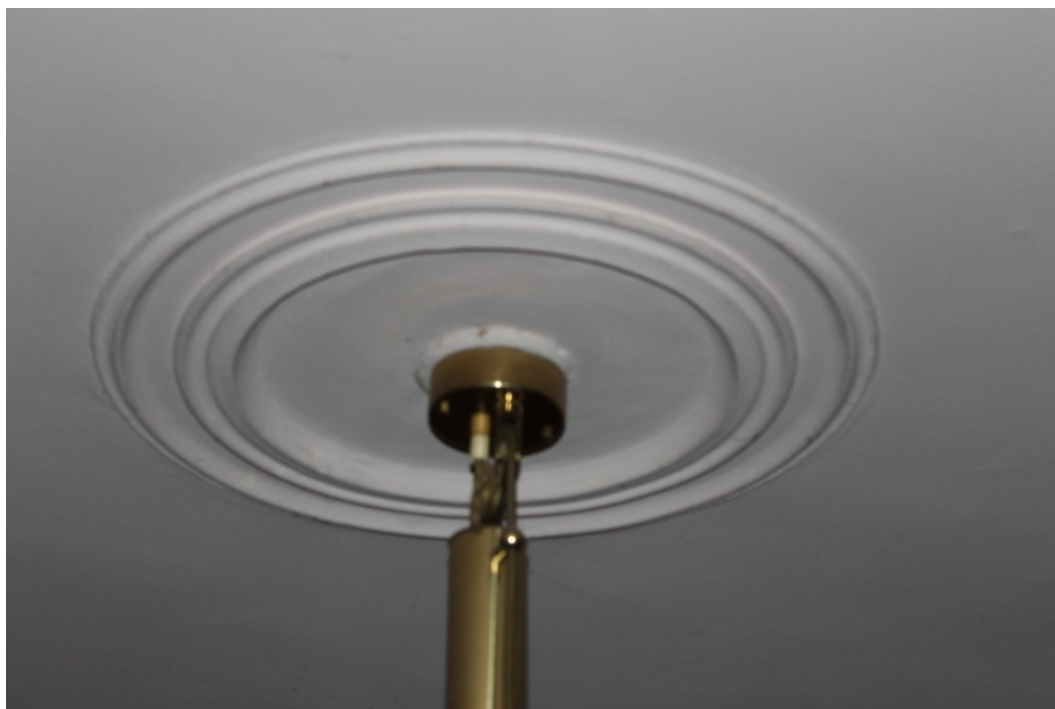
Photograph 14 Detail of original ceiling rose in GF2.
