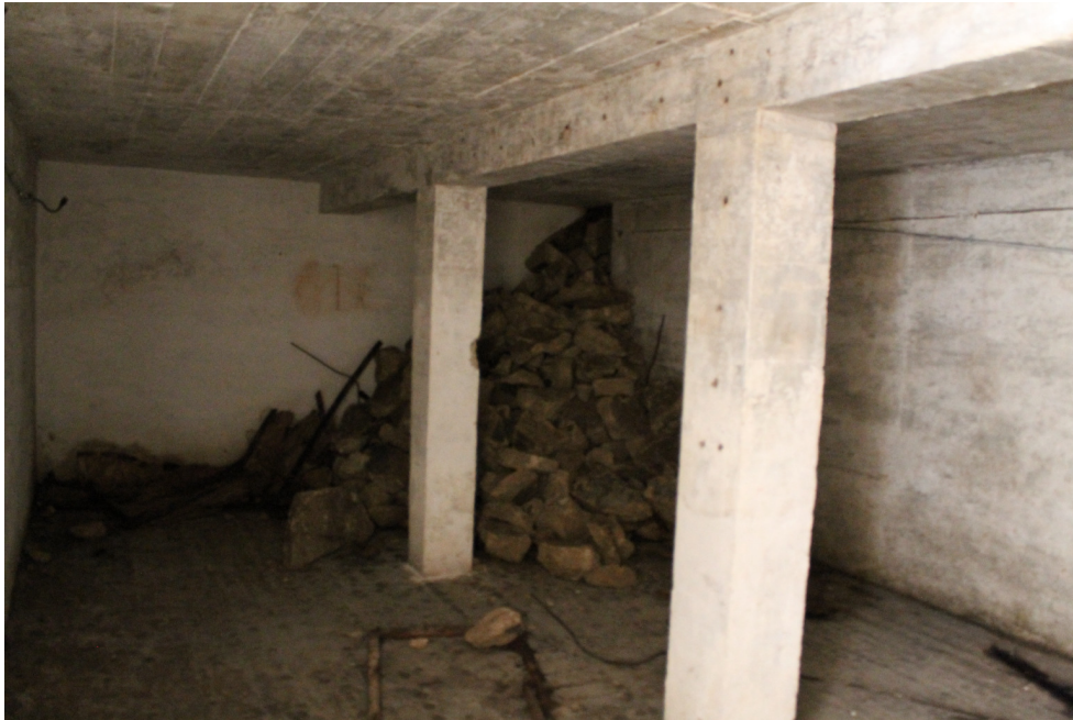
Photo 12 The interior of the air-raid shelter, viewed from the south-west.
