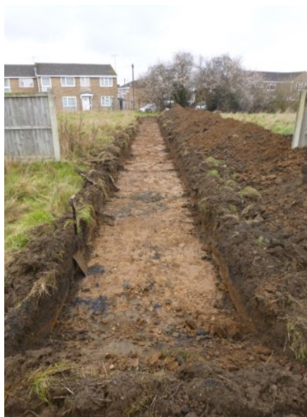
Photograph 2 T2, looking N
