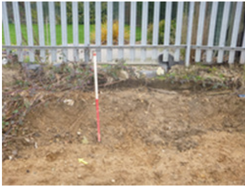
Photograph 1 Ground reduction prior to evaluation
