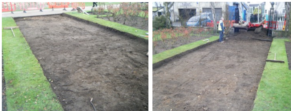
Photograph 9-10 Mid-excavation shots, looking NE and SE
