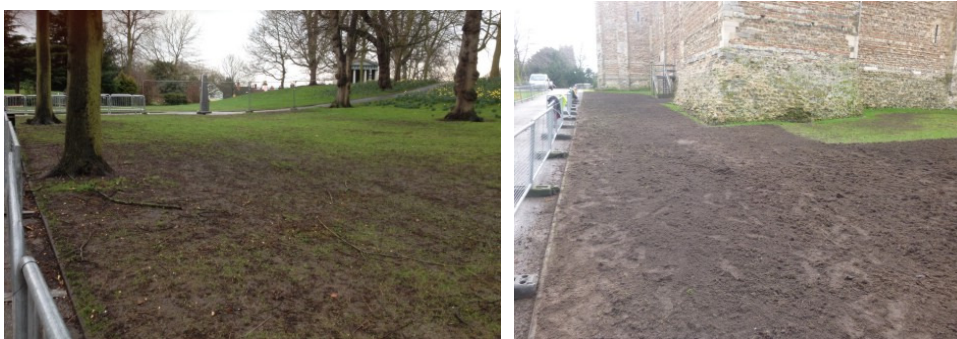
Photographs 15-16 North side of Colchester Castle with after temporary floor removed, looking NW and after rotivation of damaged grass, looking S
