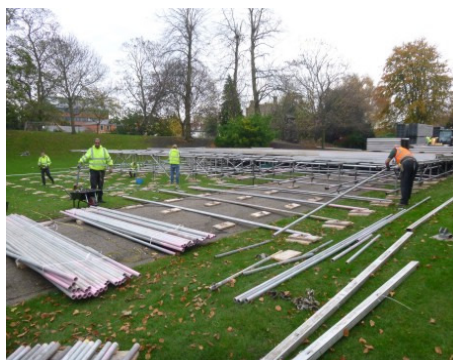
Photographs 9-10 East side of Colchester Castle during construction of raised floor for ice rink, coffee hut and skate exchange, looking SE
