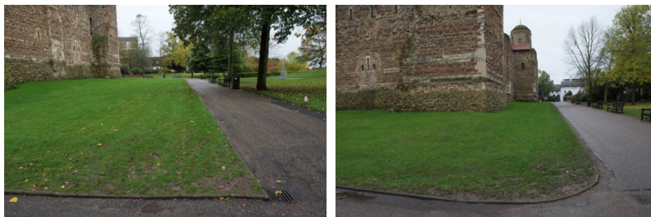
Photographs 1-2 North and east sides of Colchester Castle before construction work, looking W and S
