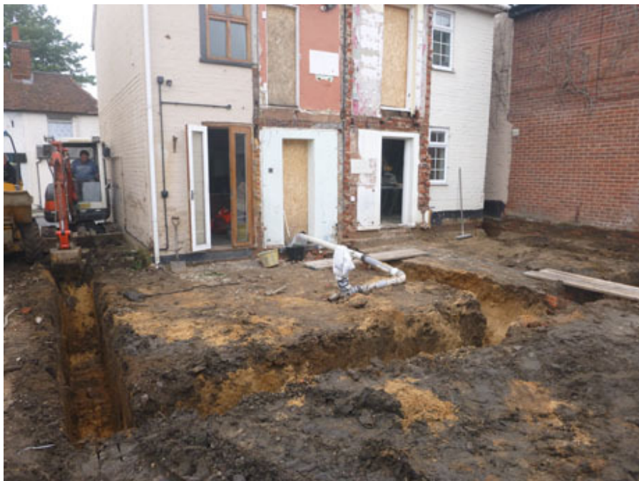
Photograph 1 Rear and side foundation trenches, looking SE
