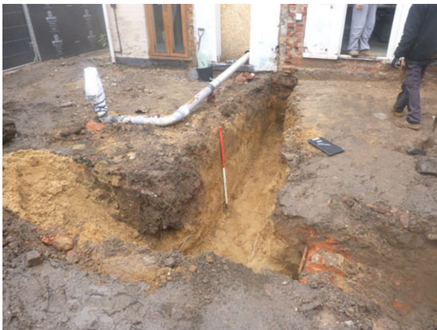
Photograph 2 Rear foundation trench, including brick manhole and pit F2, looking SE
