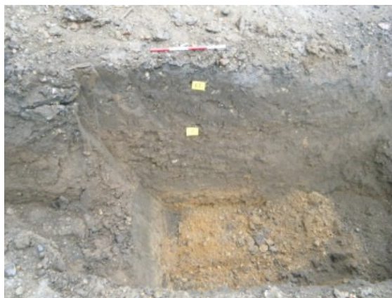
Photograph 11 Manhole representative section, looking E
